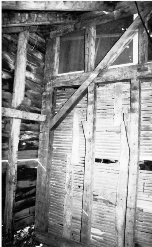
Figure 14. Top. Interior view of north wall of the nonextant 1839 stage inn/tavern. Bottom. Detail of tavern's hewn and whip-sawn framing with nogging removed. Photos 1992 by author.
