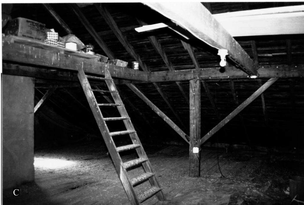
Figure 19. A. Massive foundation stones and hewn timber floor joists. B. View of corbelled arch in brick chimney base. C. View of third floor framing and ladder to former cupola loft. Photos 1992 by author.
