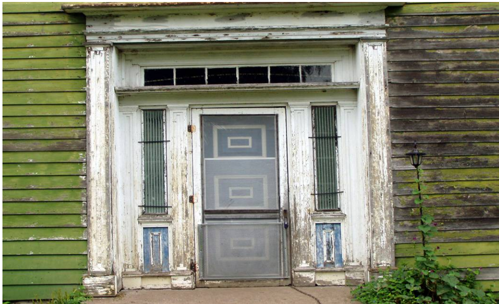
Figure 17. Top. View of the western side. Note fixed half-fan windows flanking double-hung central light. Bottom. Formal entry with Classical entablature with transom and side lights framing a multi-paneled door. Note bases to columns along with simple caps supporting flat entablature. Photos 1992 by author.
