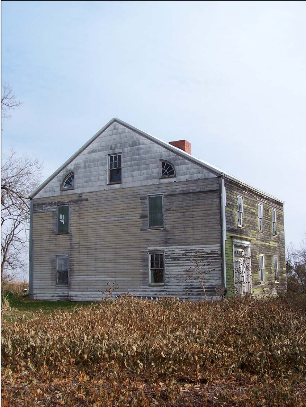
1. View of Beers and St. John Company Coach Inn looking northeast.
