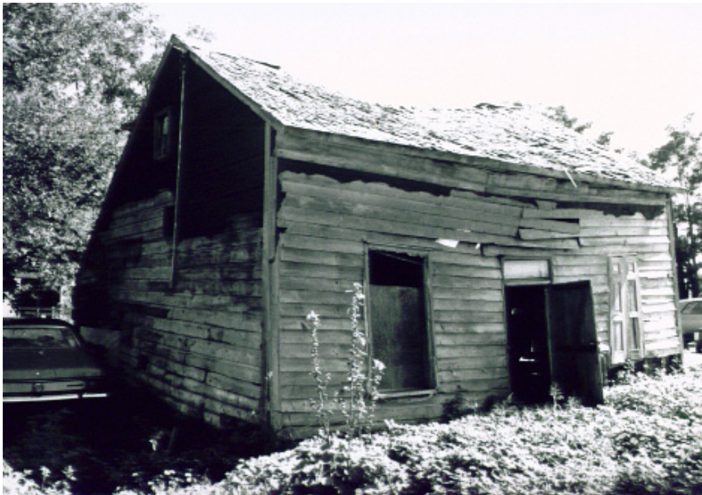
Figure 12. The nonextant 1839 tavern/inn located at angle west of house. Top. View looking north. Bottom. The western and southern sides of same (see Figure 15:top). Photos 1992 by author.
