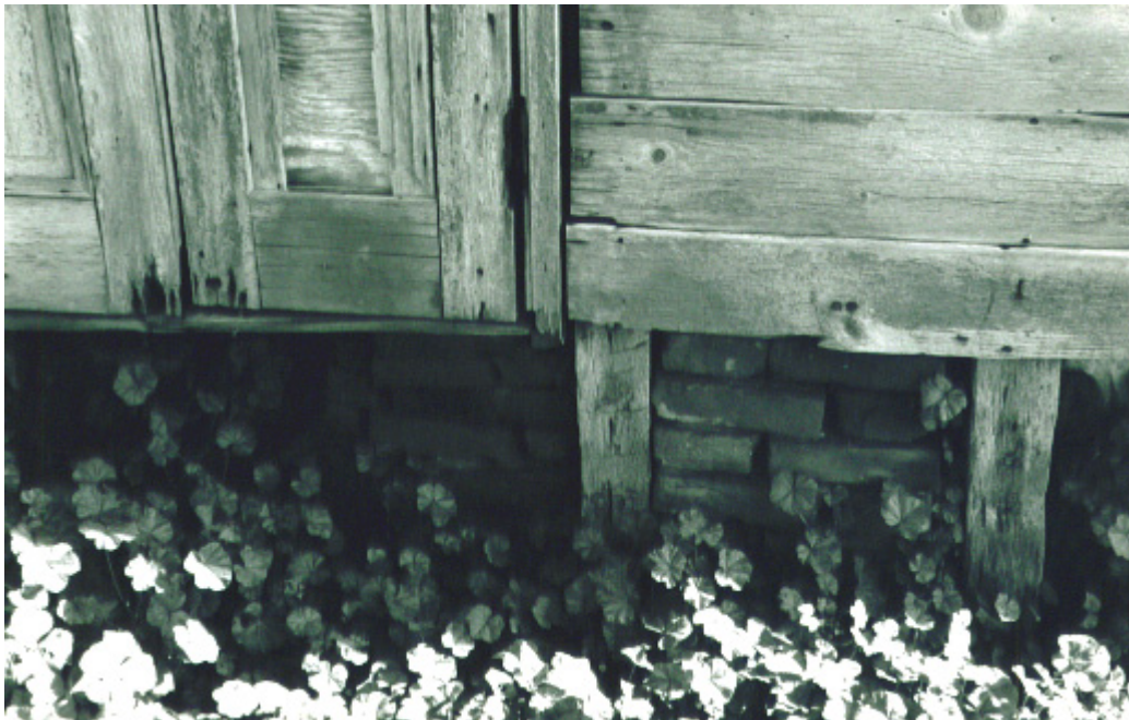
Figure 13. Top. View of lean-to or salt-box roof line on northern side of 1839 inn/tavern. The northwest corner was the reputed location of 1836 to 1838 surveyor's shack. The open part to the left in the picture was where the horses were kept. Bottom. Detail of recess paneled door, cypress siding, whip-sawn and hewn over-full-dimension studs, and soft-paste brick nogging. Photos 1992 by author.
