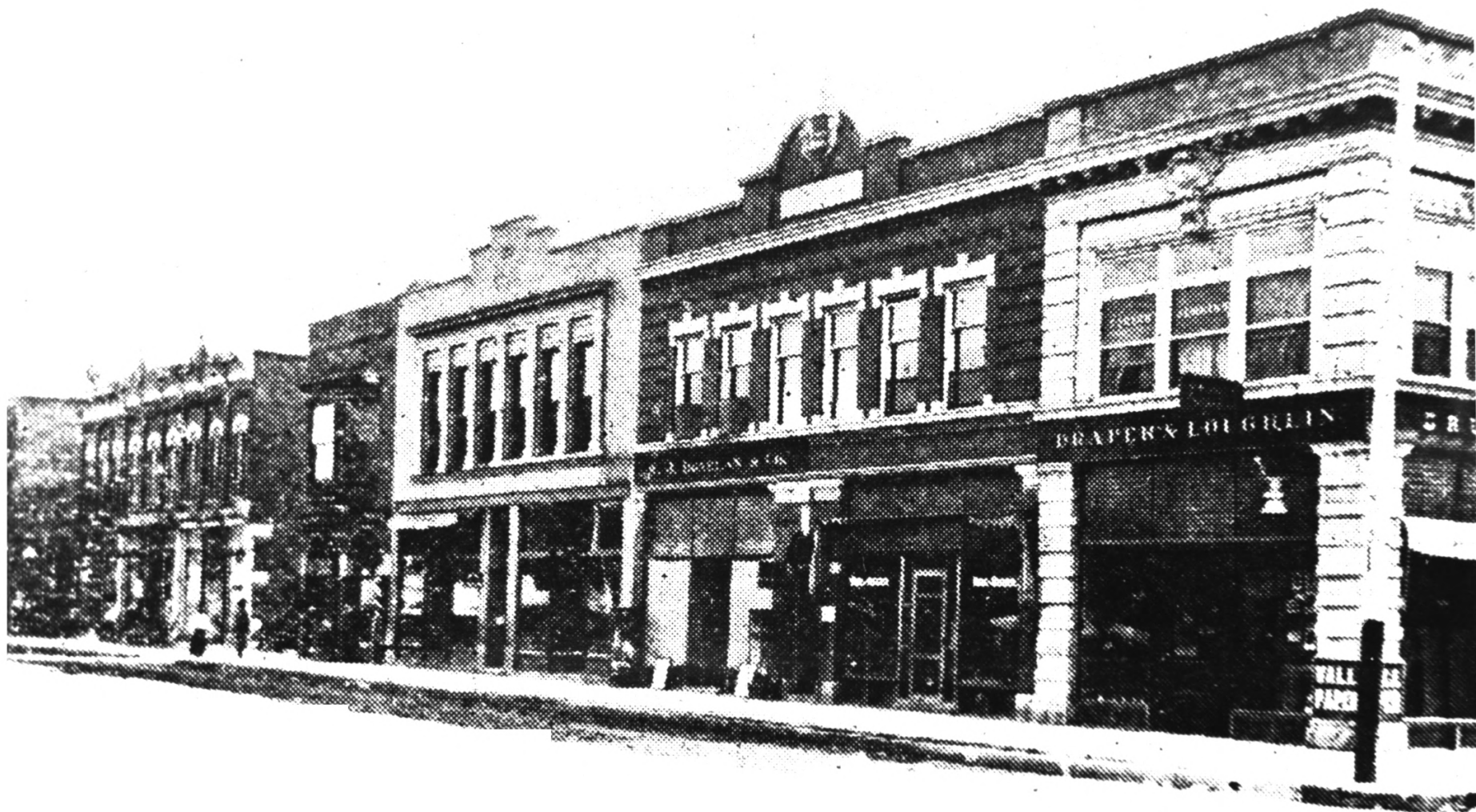
View on South Side of Square.
