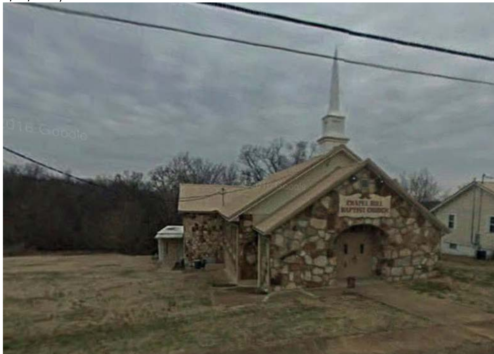
Figure 11: Chapel Hill Baptist Church located at 610 Chestnut Street, in Thayer. This church building was constructed in 1936 with a 1952 addition constructed by Charlie Angotti 41 . (Source Google streetview, accessed 1/27/2017)
