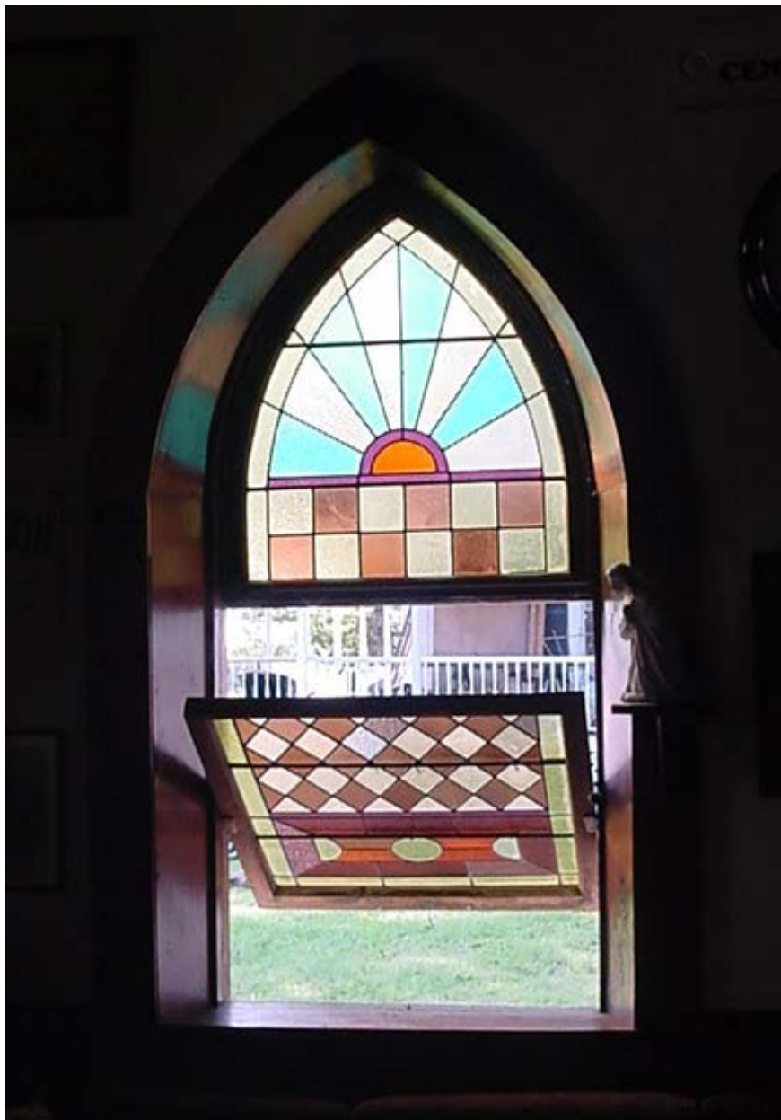
Figure 20: Detailed window, (Source: Kenneth Franke, taken 10/16)
