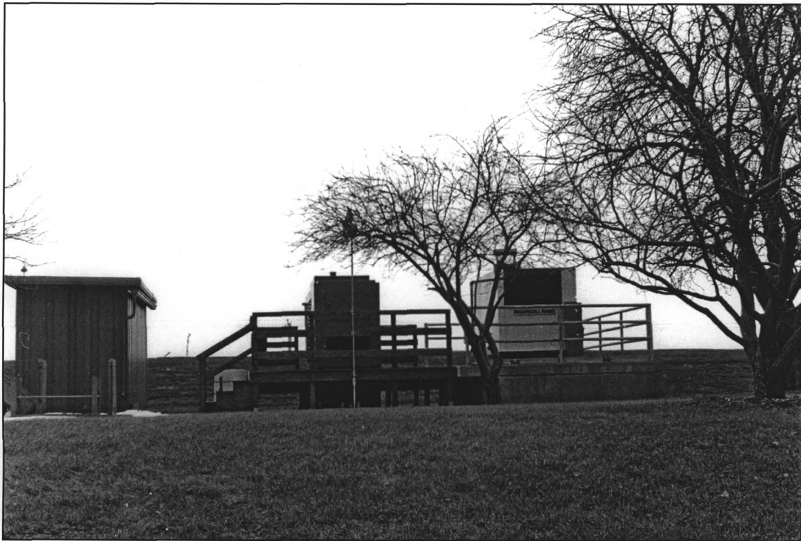
PHOTO 7. Utility Shed, Generator and Compressor.
