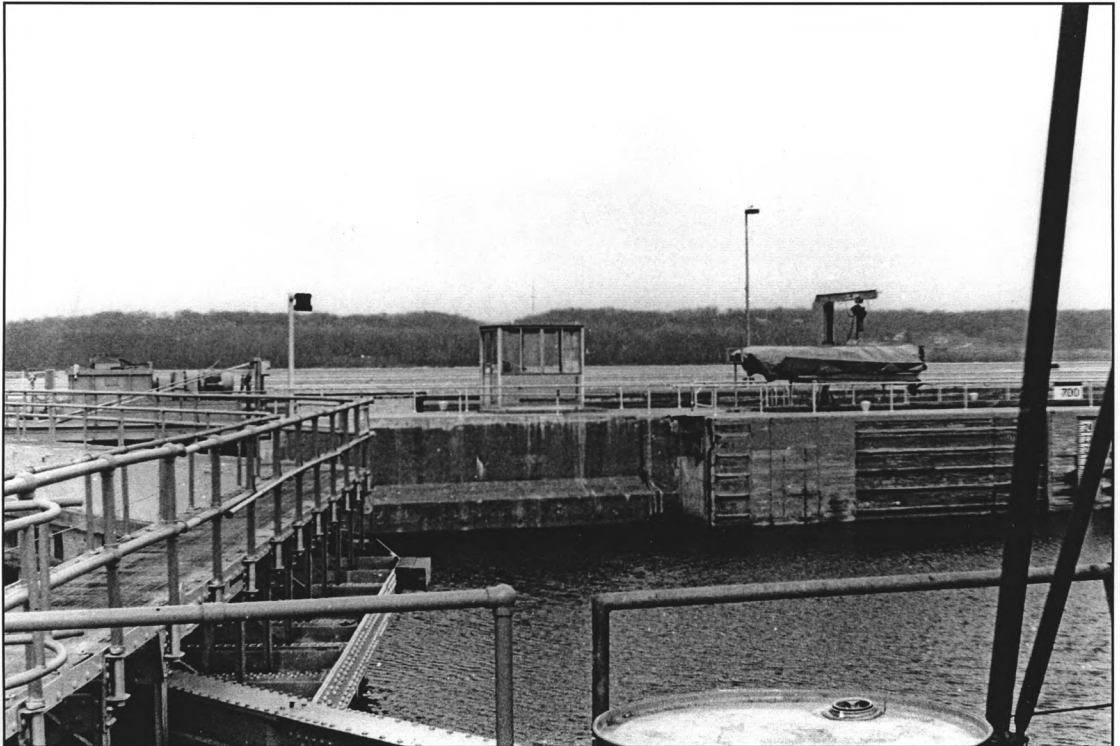
PHOTO 5. Upstream Intermediate Wall Control Stand Shelter. The downstream intermediate wall control stand shelter is identical and its placement mirrors this one at the downstream end. Both were originally constructed for use on the land wall, but were moved to the intermediate wall when new brick and glass land wall control stand shelters were constructed in 1993.
