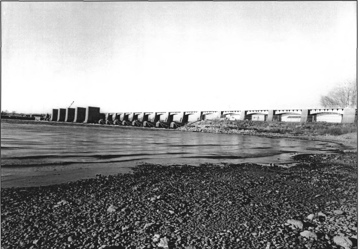
PHOTO 3. General View of Moveable Section of Dam, Downstream Side. Photographer: Peter A. Rathbun Date of Photograph: September 1987 Location of Original Negative: IA-26-1, HAER, IOWA, 70-MUSCA.B,1-HAER Collection, Prints and Photographs Division, Library of Congress, Washington, D.C. View: From west end of Hog Island, looking southeast
