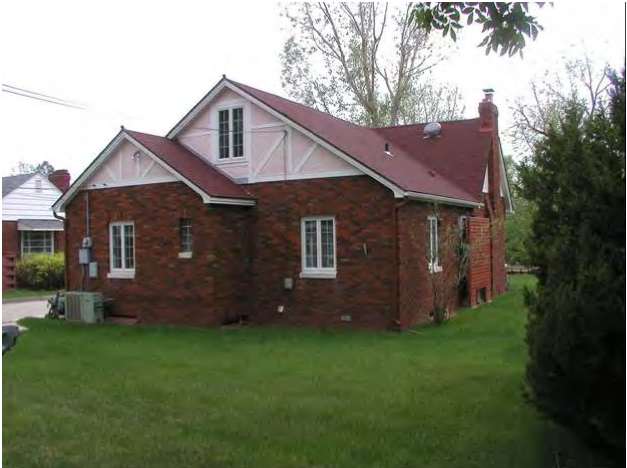
Description and view of camera: North and West elevations, view to southeast Photograph: MT_YellowstoneCounty_ArnoldGrafHouse_0007
