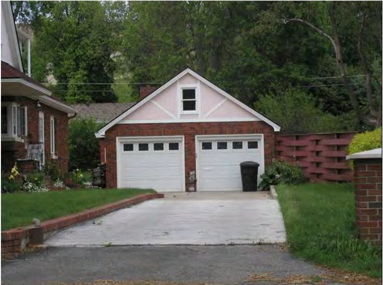
Description and view of camera: South elevation, Garage, view to north Photograph: MT_YellowstoneCounty_ArnoldGrafHouse_0008
