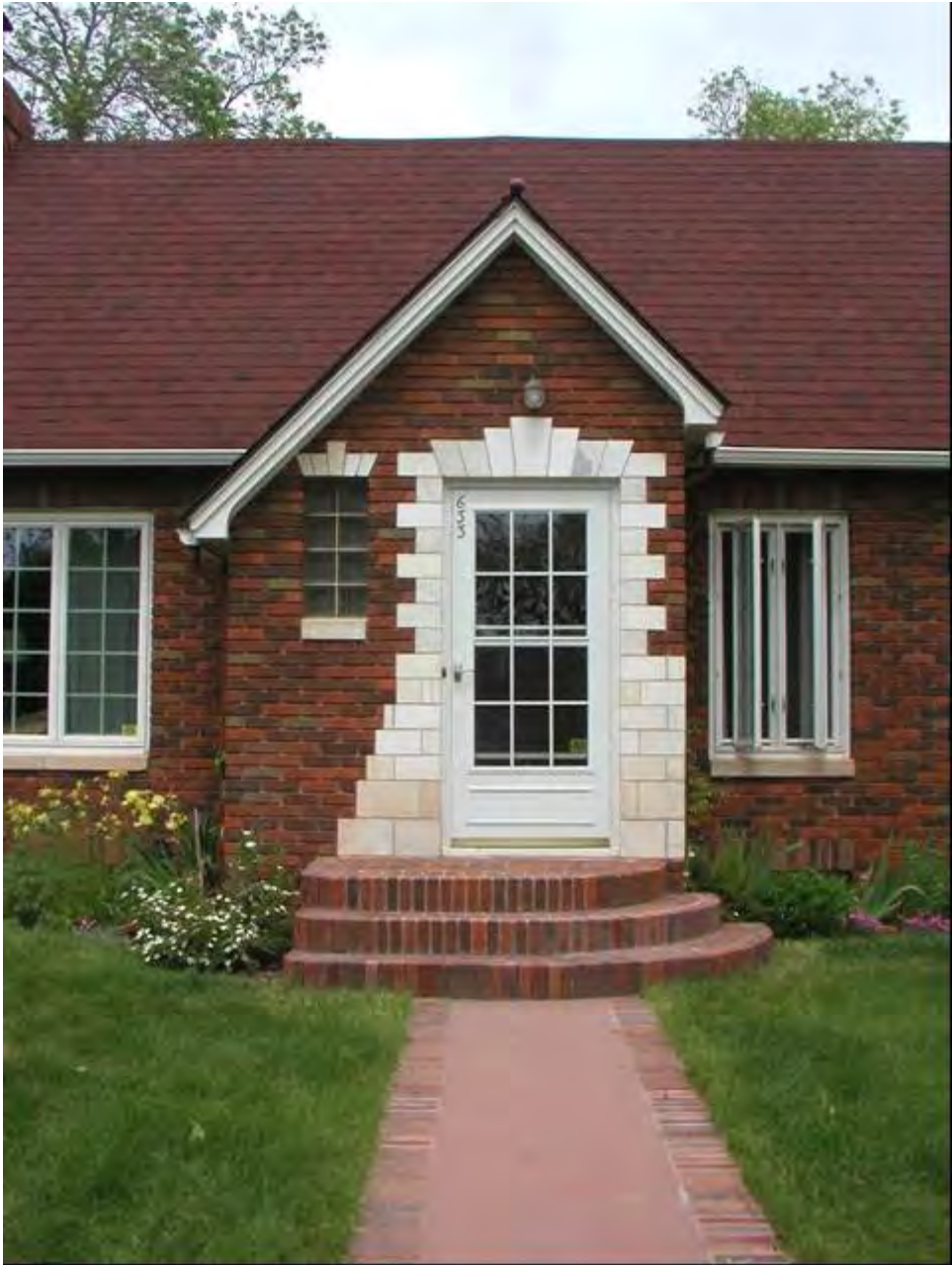
Description and view of camera: Front vestibule, view to north. Photograph: MT_YellowstoneCounty_ArnoldGrafHouse_0003
