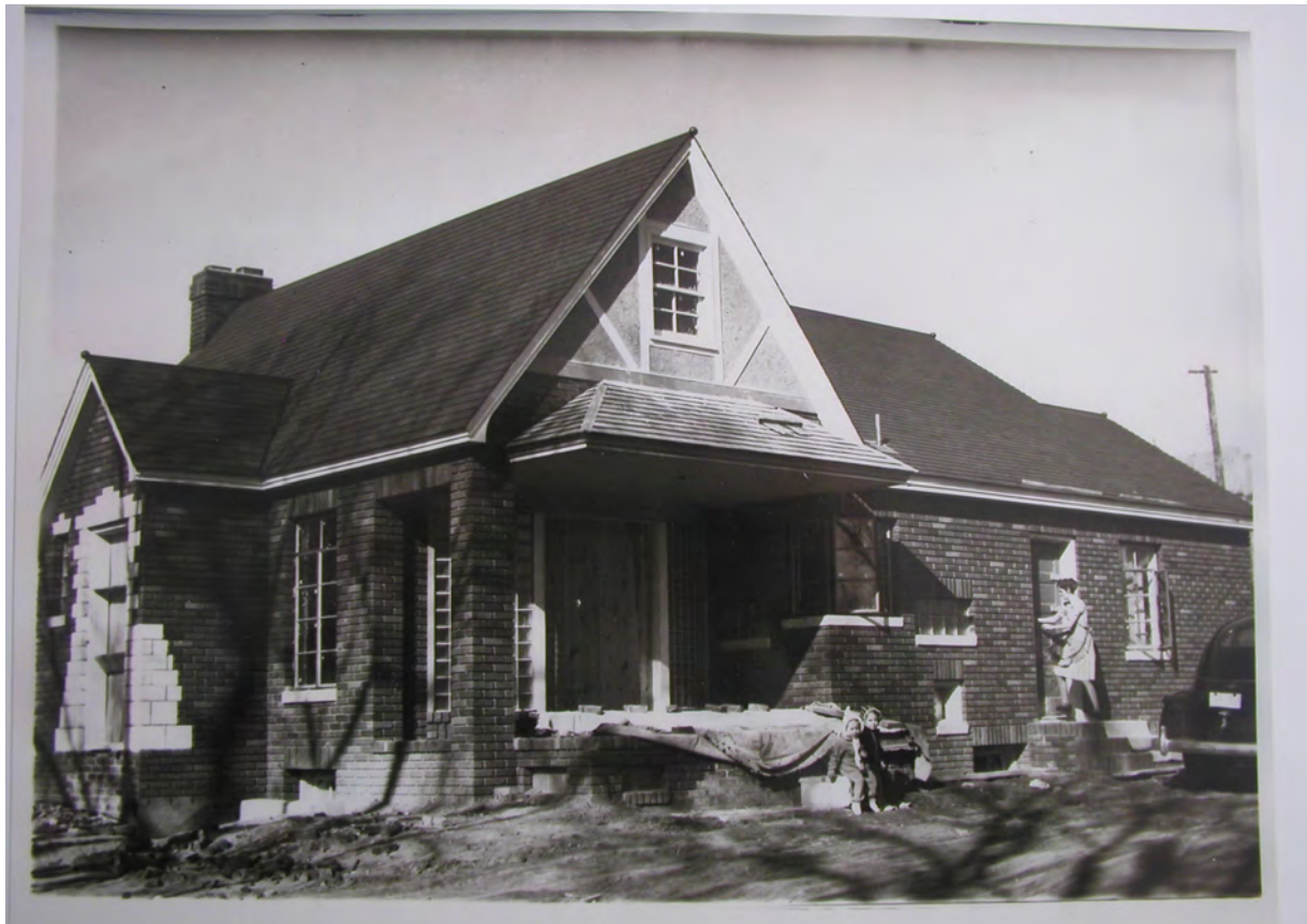
1940 Construction photograph, view to northwest
