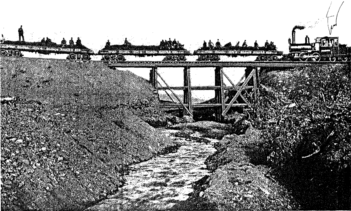
FIRST STANDARD GAUGE TREESTLE IN ALASKA—ROCK CREEK, ON LINE OF COUNCIL CITY & SOLOMON RIVER RAILROAD.
