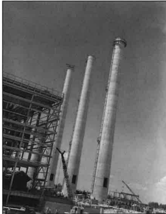
Figure 3. August 19, 1952 image of the construction of the SHF powerhouse.
