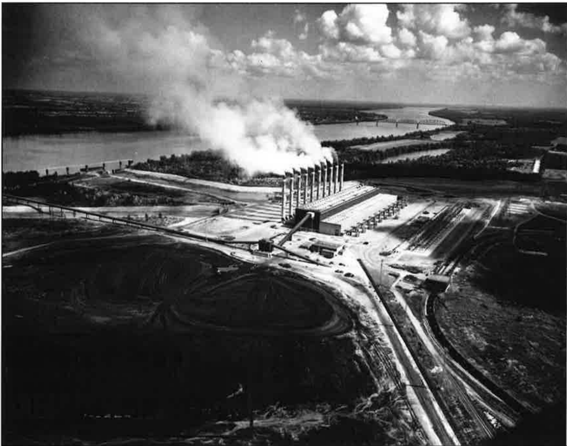
Figure 6. Aerial image from September 1961 showing the completed SHF facility; view is northeast.
