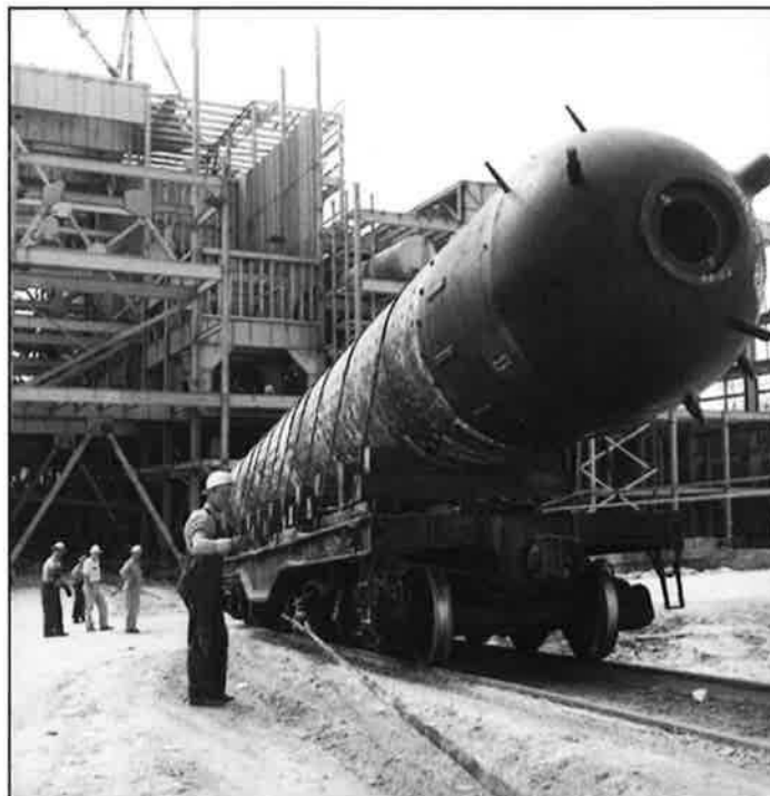
Figure 4. August 19, 1952 image of the installation of SHF's first boiler drum.
