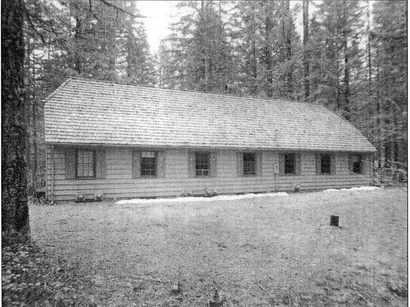
Region 6 Personnel Training Station, G.F. Allen Dormitory Gifford Pinchot National Forest
