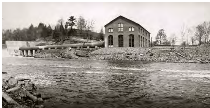
Figure 5 Tariffville Power House. Photo courtesy of the University of Connecticut Archives and Special Collections.
