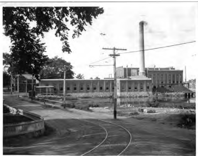
Figure 6 Mystic Power House and Car House. Photo Courtesy of the University of Connecticut Archives and Special Collections.
