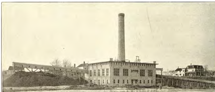
Figure 4 The Power House at Old Saybrook. Photo Courtesy of the 1911 Electric Railway Journal .
