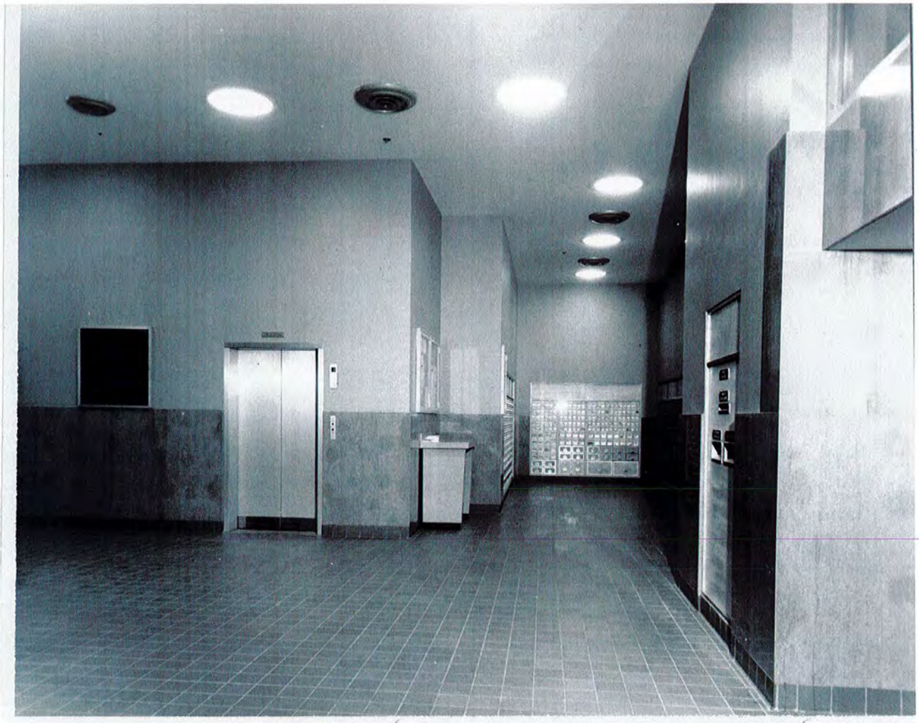
View of the main lobby of the Hot Springs U.S. Post Office and Courthouse, looking south, c.1960. (Courtesy of the General Services Administration Region 7 Office, Fort Worth, Texas.)
