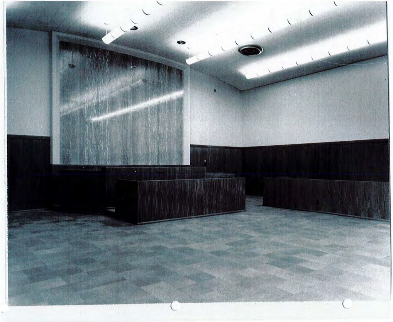
View of the courtroom of the Hot Springs U.S. Post Office and Courthouse, c.1960. (Courtesy of the General Services Administration Region 7 Office, Fort Worth, Texas.)
