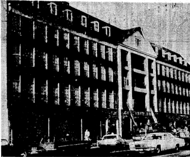
THIS IS VIEW of the exterior of Governor House Motel which showed no effect of the collapse of five floors and the roof. Firemen's ladders rest against the front of the building.
