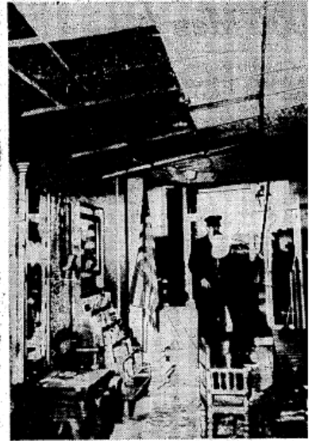
FIREMEN inspect a ceiling which sagged when five floor and roof of Governor House Motel collapsed due to failure of a construction support Friday.
