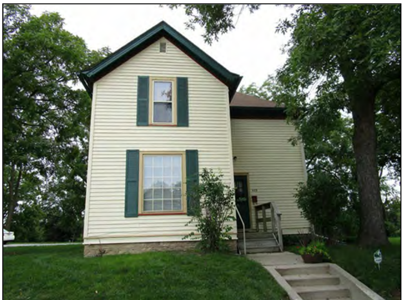
Figure 5. Façade of 423 W 1st Street looking North. Photograph obtained from Black Hawk County Assessor, accessed at http://www2.co.black-hawk.ia.us/ , 2018.
