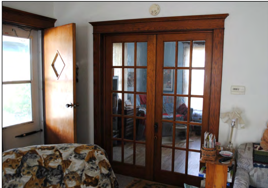
Figure 23. Interior of front rooms of 509 W. 1st Street showing French doors that have oak woodwork including egg-and-dart molding on the lintel. Photograph is looking WSW; taken 08-07-2018 by Tallgrass.
