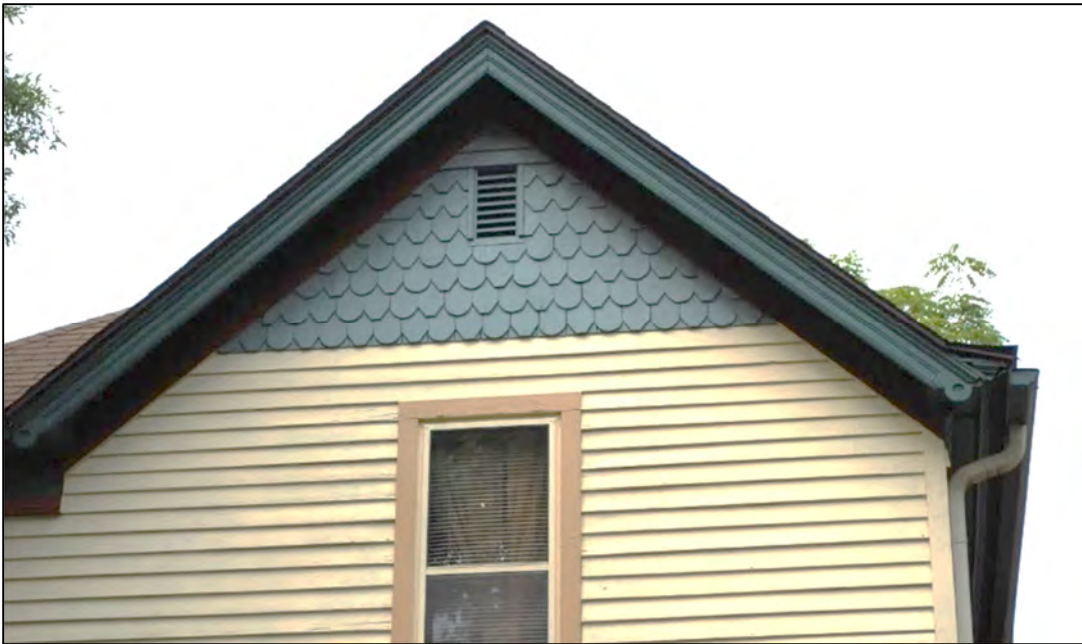
Figure 7. East gable of 423 W. 1 st Street showing the fish-scale siding and decorative vergeboards and flared eaves. Photograph taken 08-07-2018 by Tallgrass.
