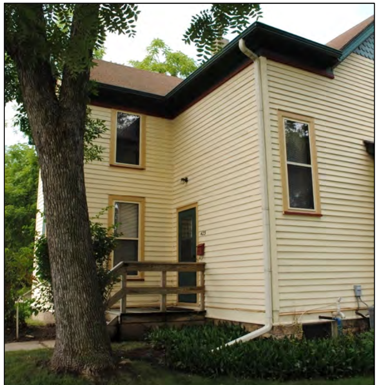
Figure 10. 423 W. 1st Street looking WNW showing area where original front porch was once located. Photograph taken 08-07-2018 by Tallgrass.
