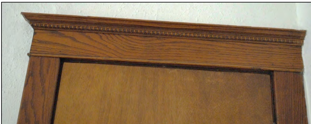
Figure 24. Example of egg-and-dart molding on lintel boards on interior of 509 W. 1st Street. Photograph taken 08-07-2018 by Tallgrass.
