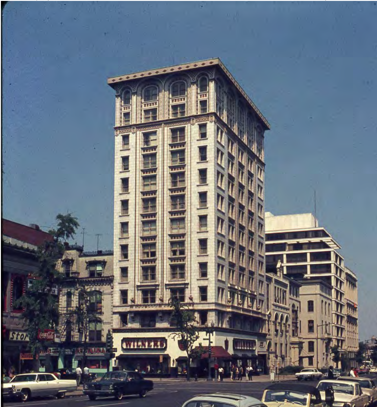
View of Real Estate Trust building (then known as Landmark Building), ca. 1968 (From Historical Society of Washington, #PR1661B)
