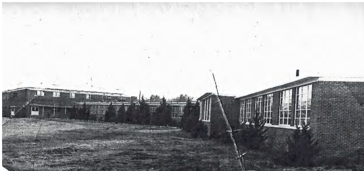
Figure 3: Carver High School, c.1960, with high school building to far right, original building at center, and gymnasium at left.
