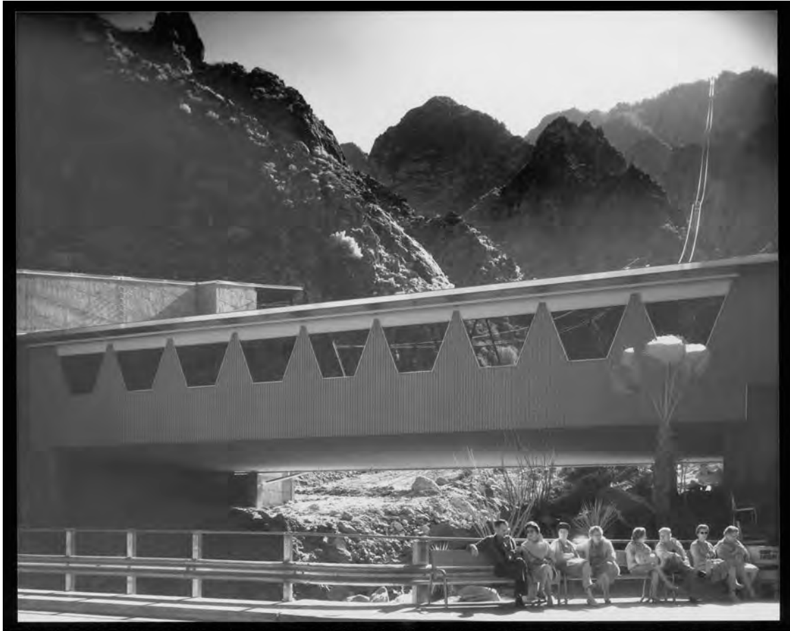
Figure 2. Northeast elevation, looking southwest, 1964.
