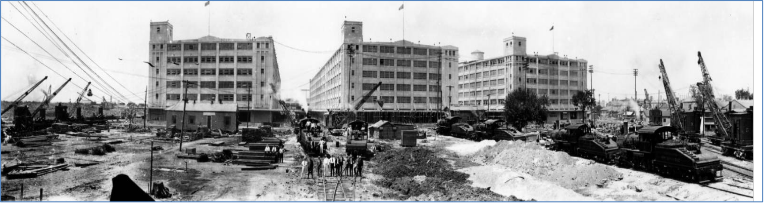
Figure 1. Photo of the three main buildings on the site being constructed in December 1918. Image courtesy of Historic New Orleans Collection; Charles L. Franck; December 18, 1918.
