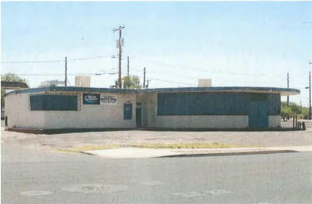
AZ_PimaCounty_MiracleMileHistoricDistrict_0015 Main Avenue, camera looking southeast, rounded café façade.
