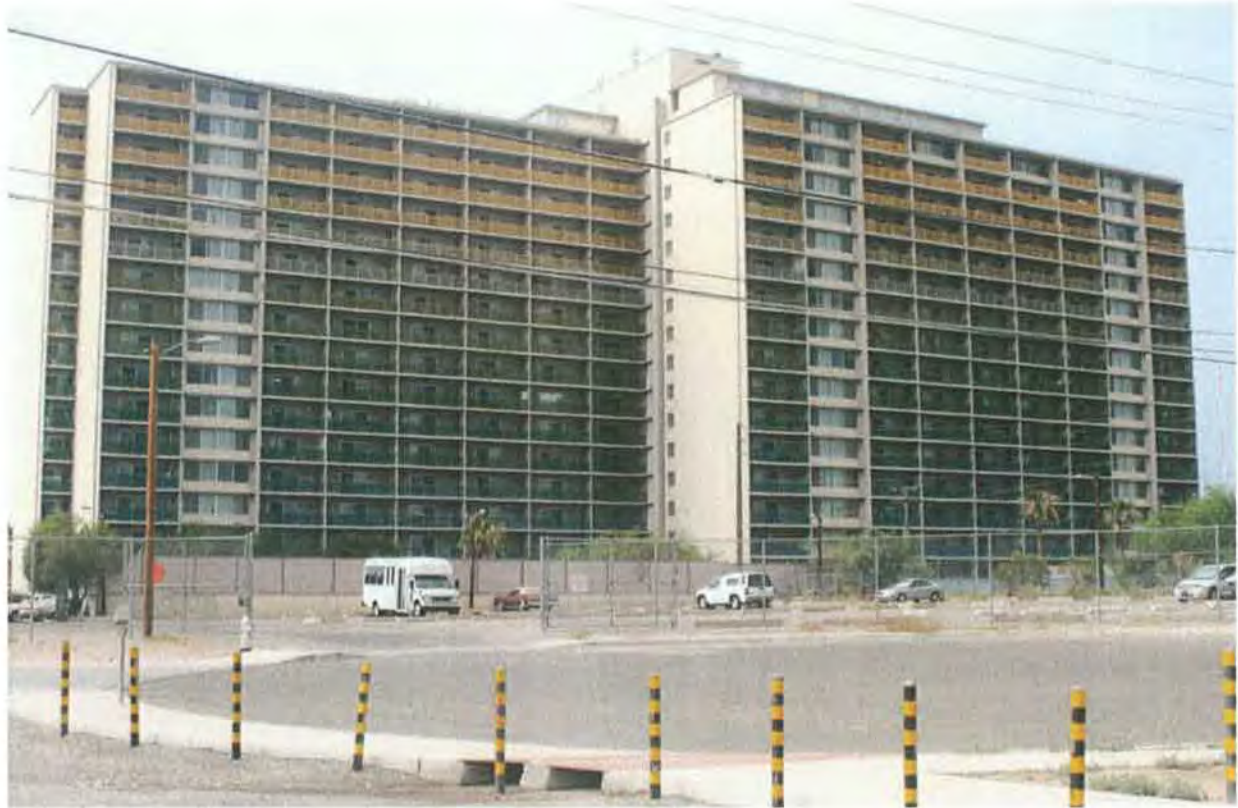
AZ_PimaCounty_MiracleMileHistoricDistrict_0019 Oracle Road, camera looking northeast, Tucson House building south façade.
