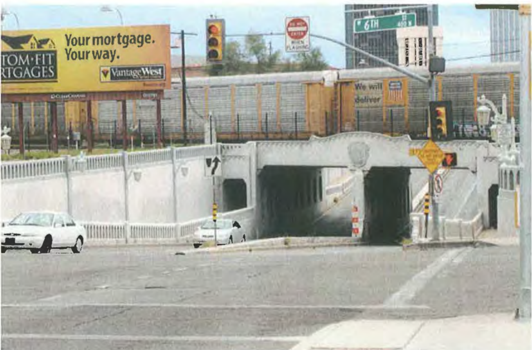
AZ_PimaCounty_MiracleMileHistoricDistrict_0010 Stone Avenue, camera looking southeast, Stone Avenue Underpass.
