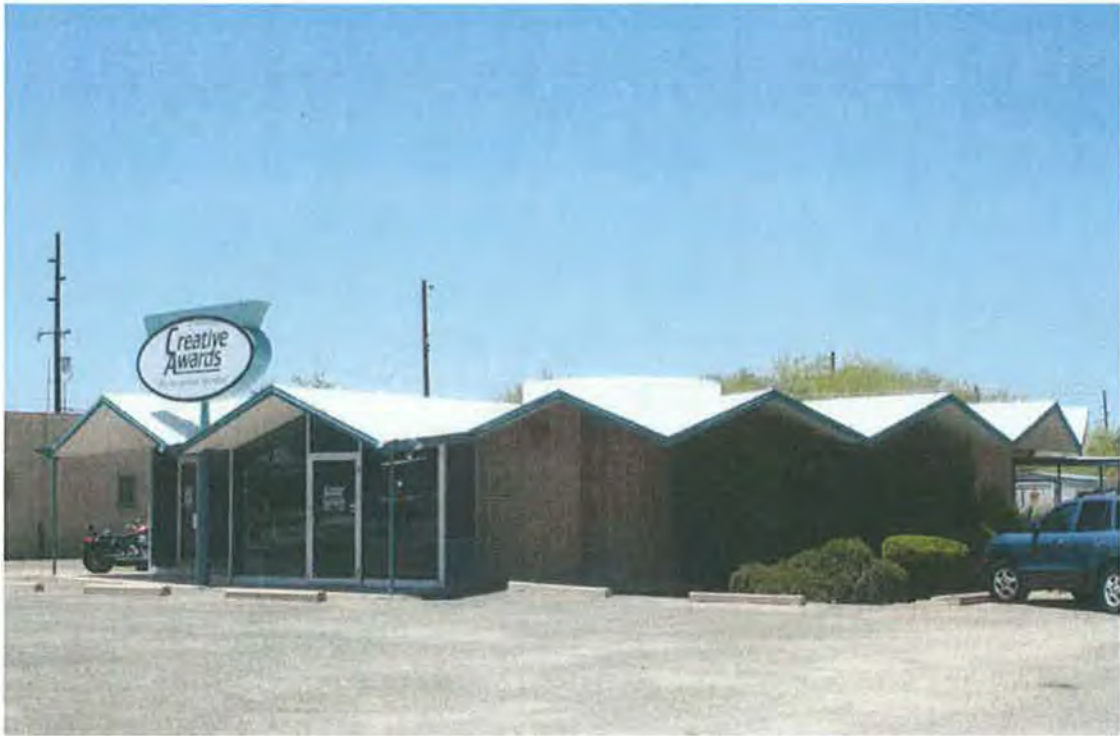
AZ_PimaCounty_MiracleMileHistoricDistrict_0013 Drachman Street, camera looking northwest, exuberant modern form.
