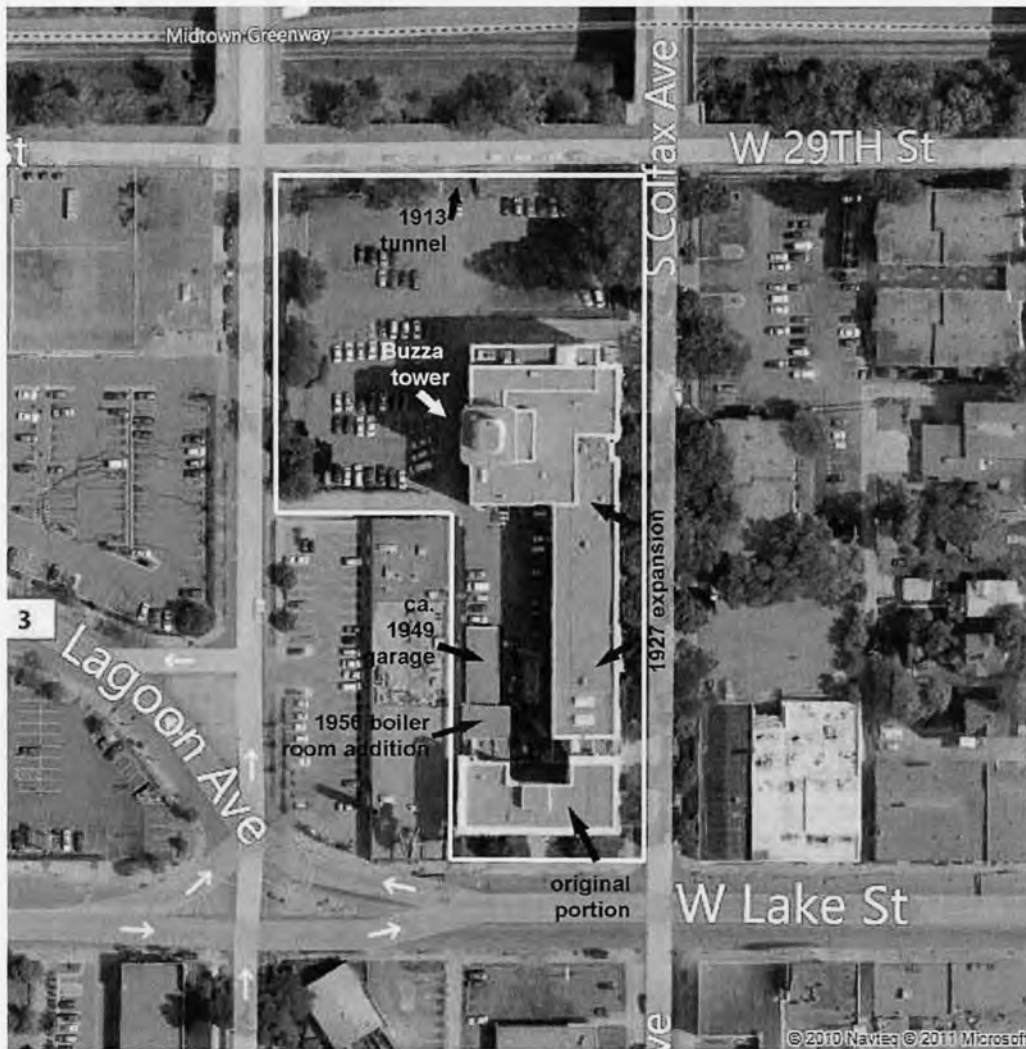
Figure 2: Aerial image of Buzza Company Building, indicating components of the property
