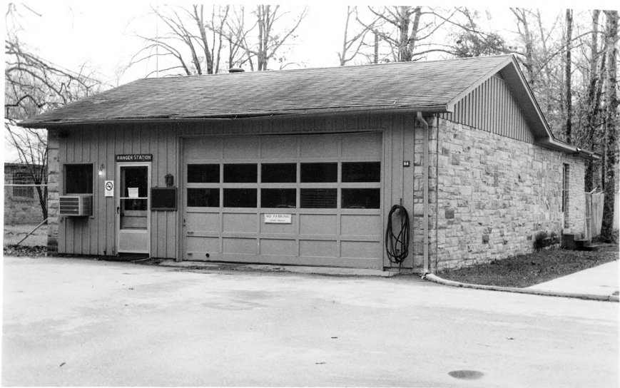
1. Fire Hall (064) Maintenance Area Mammoth Cave National Park, Kentucky
