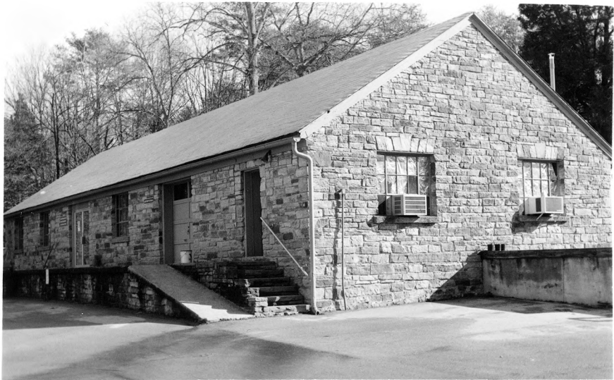
4. Warehouse (063), Maintenance Area Mammoth Cave National Park, Kentucky
