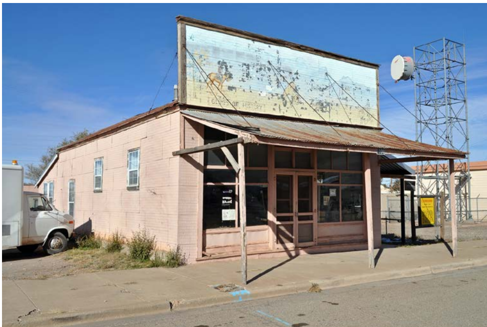
Photo 16 of 27: 1106 E Avenue, Long and Harkey Tin Shop, photographer facing northwest.
