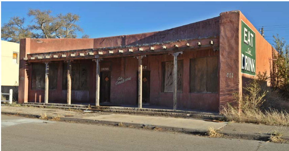
Photo 10 of 27: 411 12th Street, Yucca Bar & Grill/Sargent's Yucca Club, photographer facing northeast.
