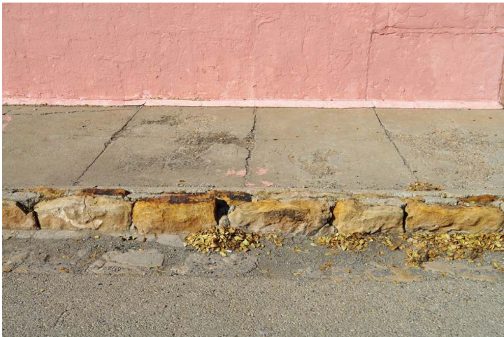
Photo 26 of 27: WPA Rock Curb and Gutter, photographer facing northwest.
