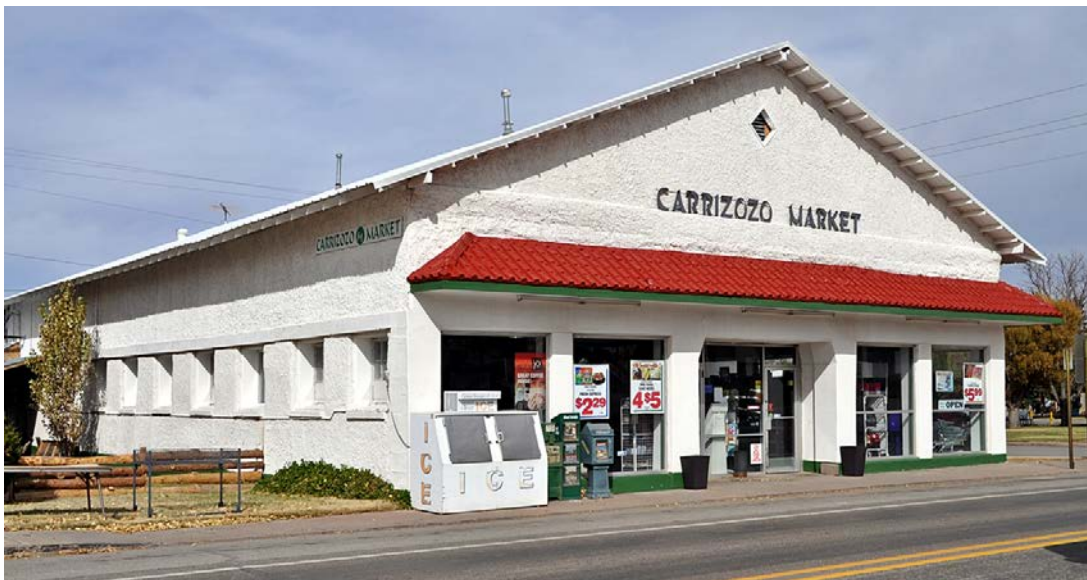
Photo 20 of 27: 400 Central Avenue, Carrizozo Community Hall, photographer facing northwest.
