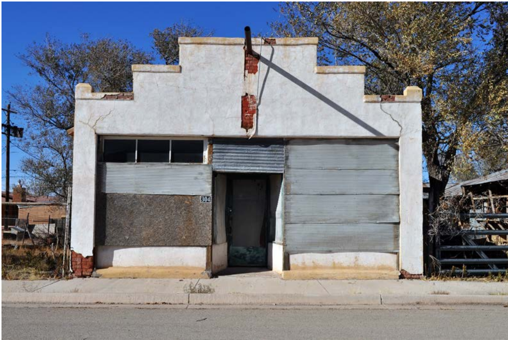
Photo 5 of 27: 304 12th Street, Bill Nickels Hardware, photographer facing northwest.
