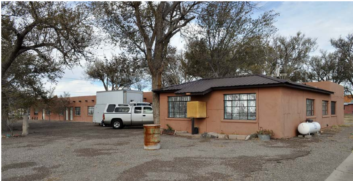
Photo 24 of 27: 1514 12 th Street, Park Motel, photographer facing northwest.
