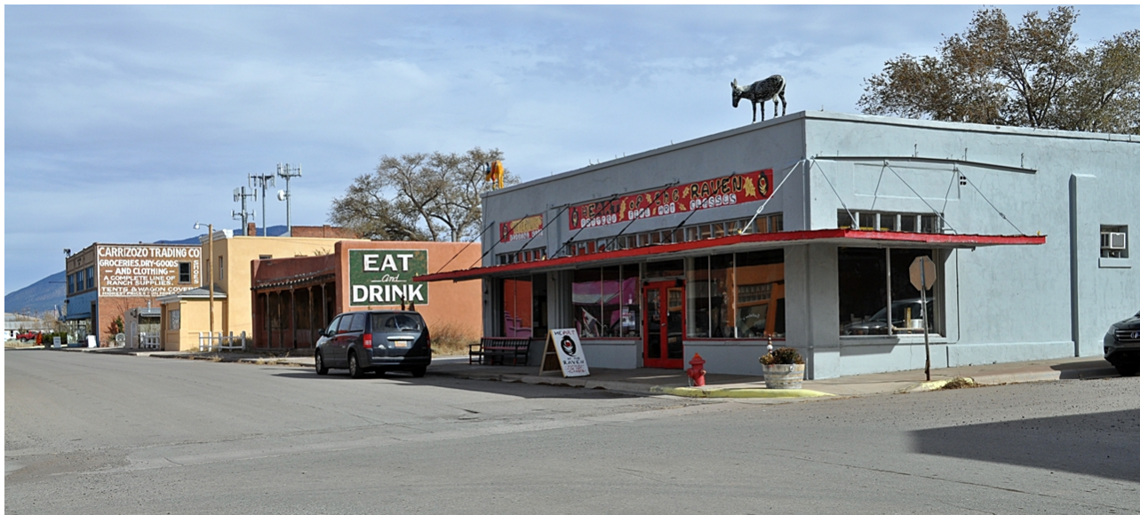
Figure 2 of 27: 300 block of 12 th Street, photographer facing northeast.
