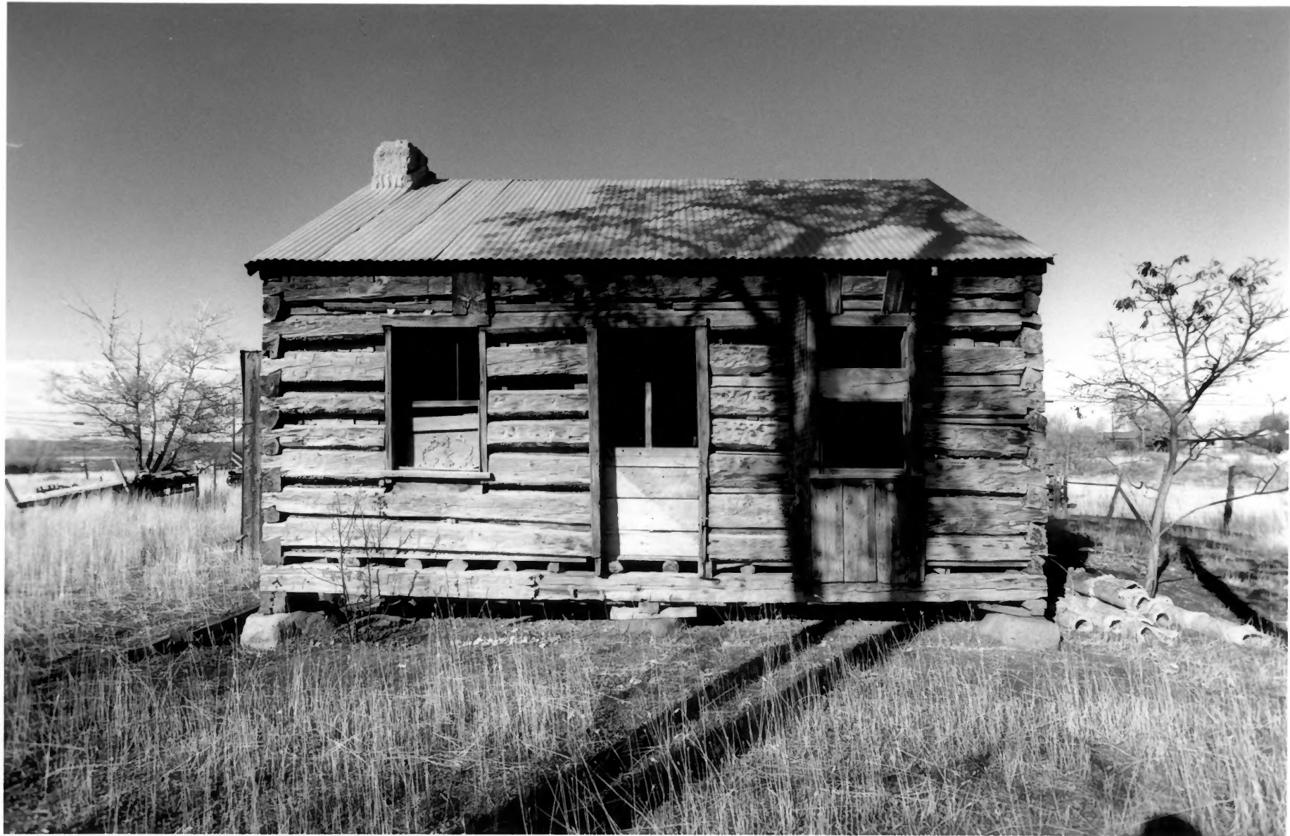
MEEKS/GREEN FARMSTEAD PAROWAN, IRON CO., UT PHOTO #2
