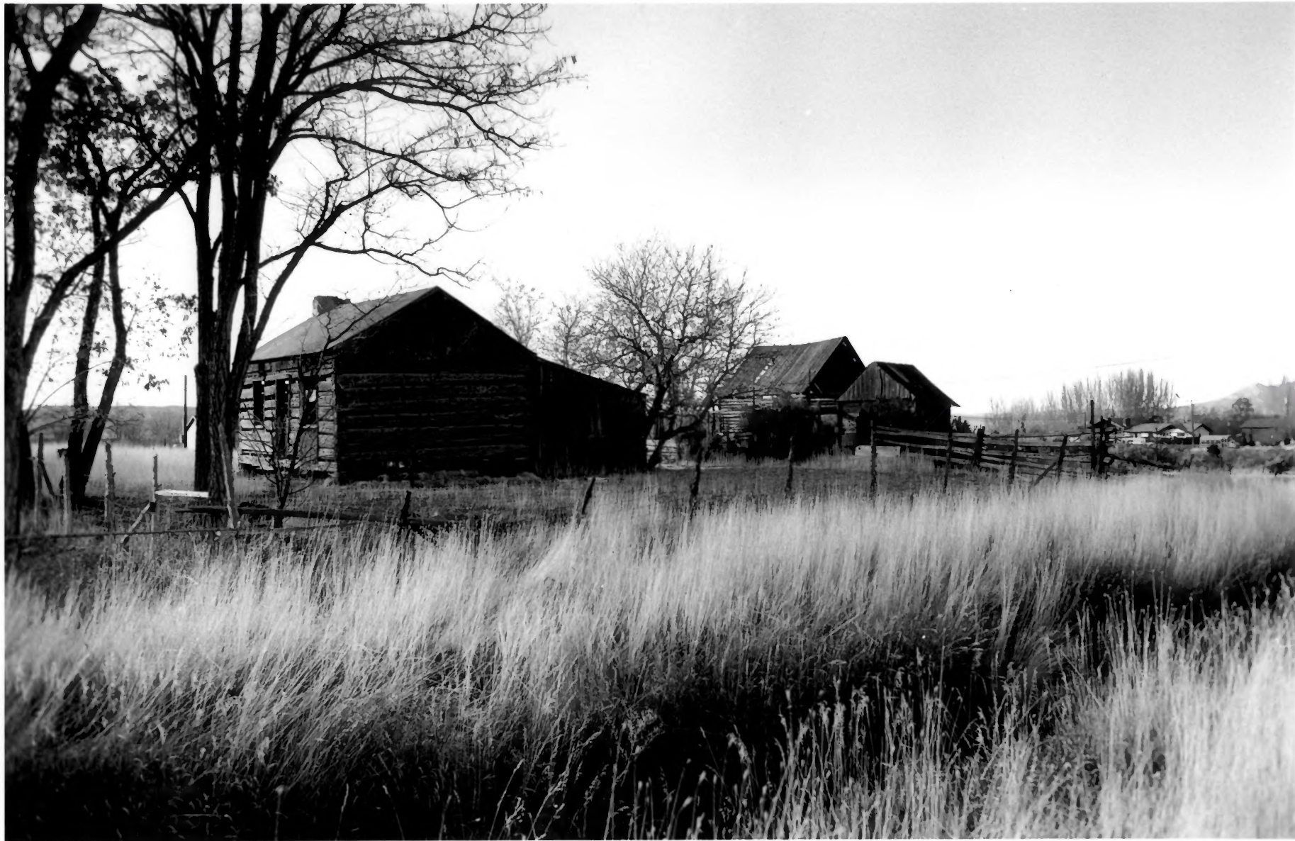
MEEKS/GREEN FARMSTEAD PAROWAN, IRON CO., UT PHOTO#1
