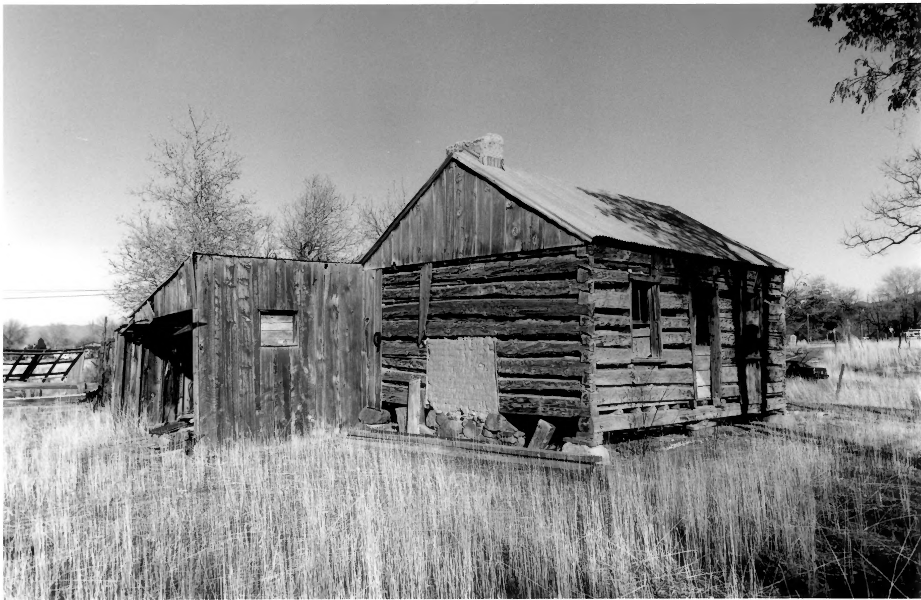
MEEKS/GREEN FARMSTEAD PAROWAN, IRON CO., UT PHOTO#3
