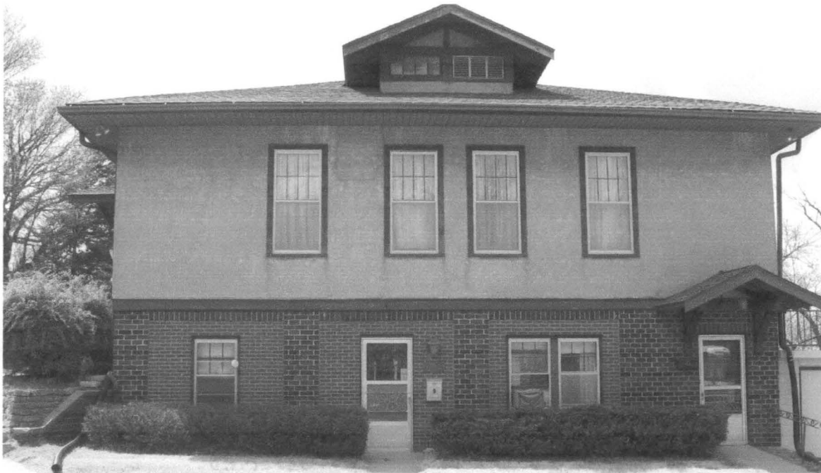
600 Huntington Avenue, Prairie School/Craftsman type (former KOIL Radio Station) Photograph taken by Tallgrass Historians L.C., 2008
