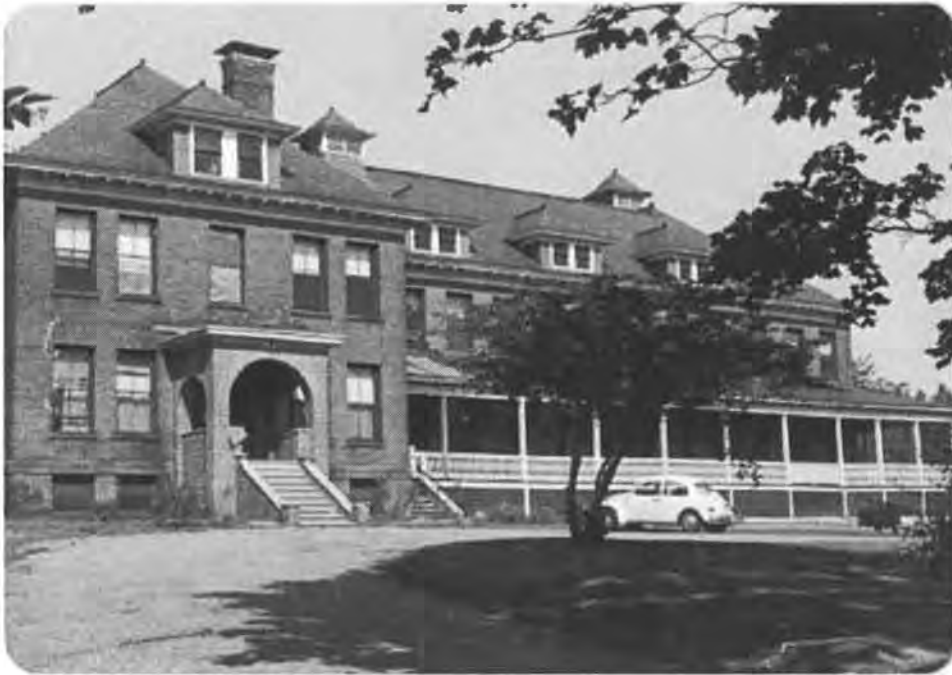
Figure 5, 1978 photograph showing the Worcester State Hospital Farmhouse (NR nomination, Worcester State Hospital)
