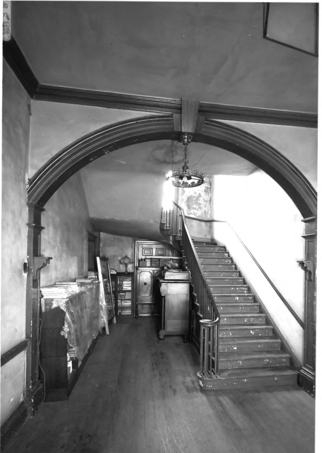
Isaac Meason House, Uniontown, Pa Photo: Jet Lowe HAER 1989 5475/16 Interior Central Hall & Stair S E
