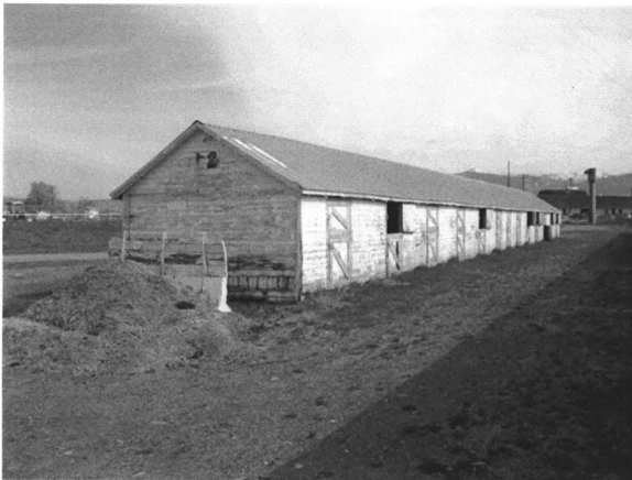
MT_MissoulaCounty_MissoulaCountyFairgroundsHD_0011 Missoula County, Montana, Daniel S. Hall, 05/02/2008, H-2, Horse Stalls, facing northeast. Photo #0011
