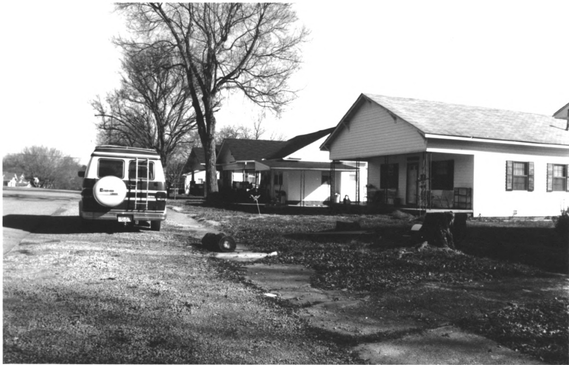
Etowah Historic District McMinn County TN
