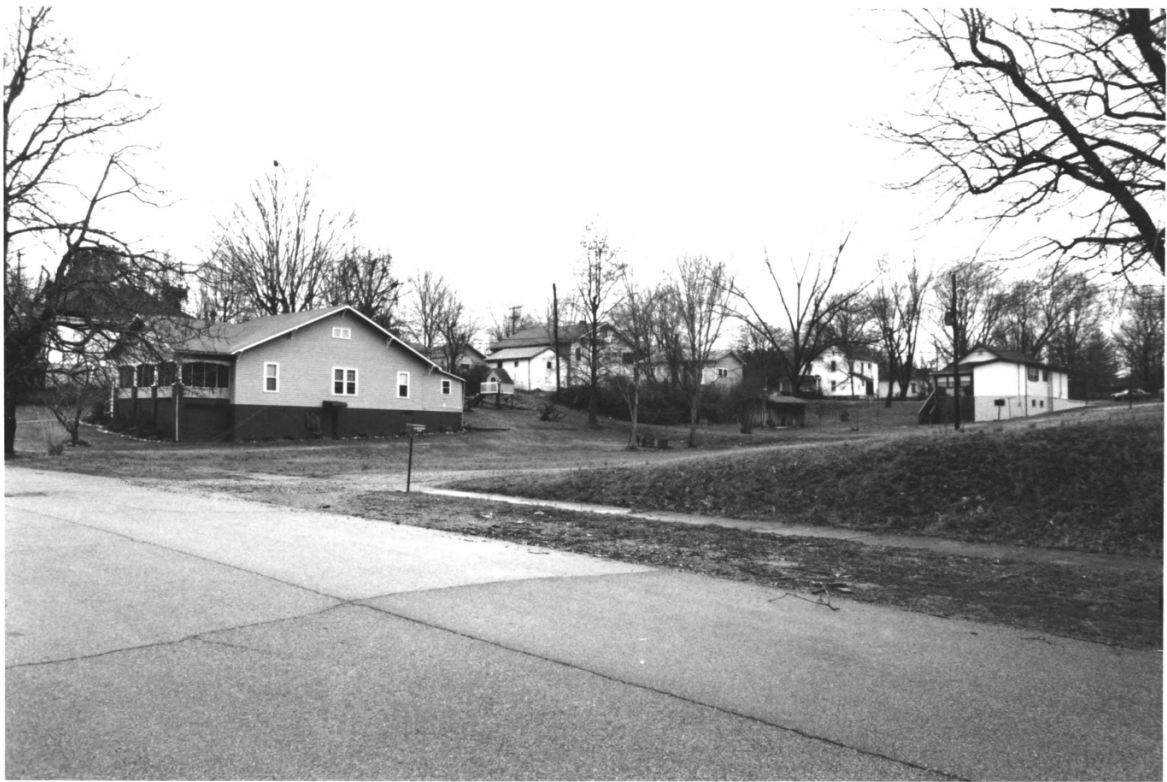
Etowah Historic District McMinn County TN
