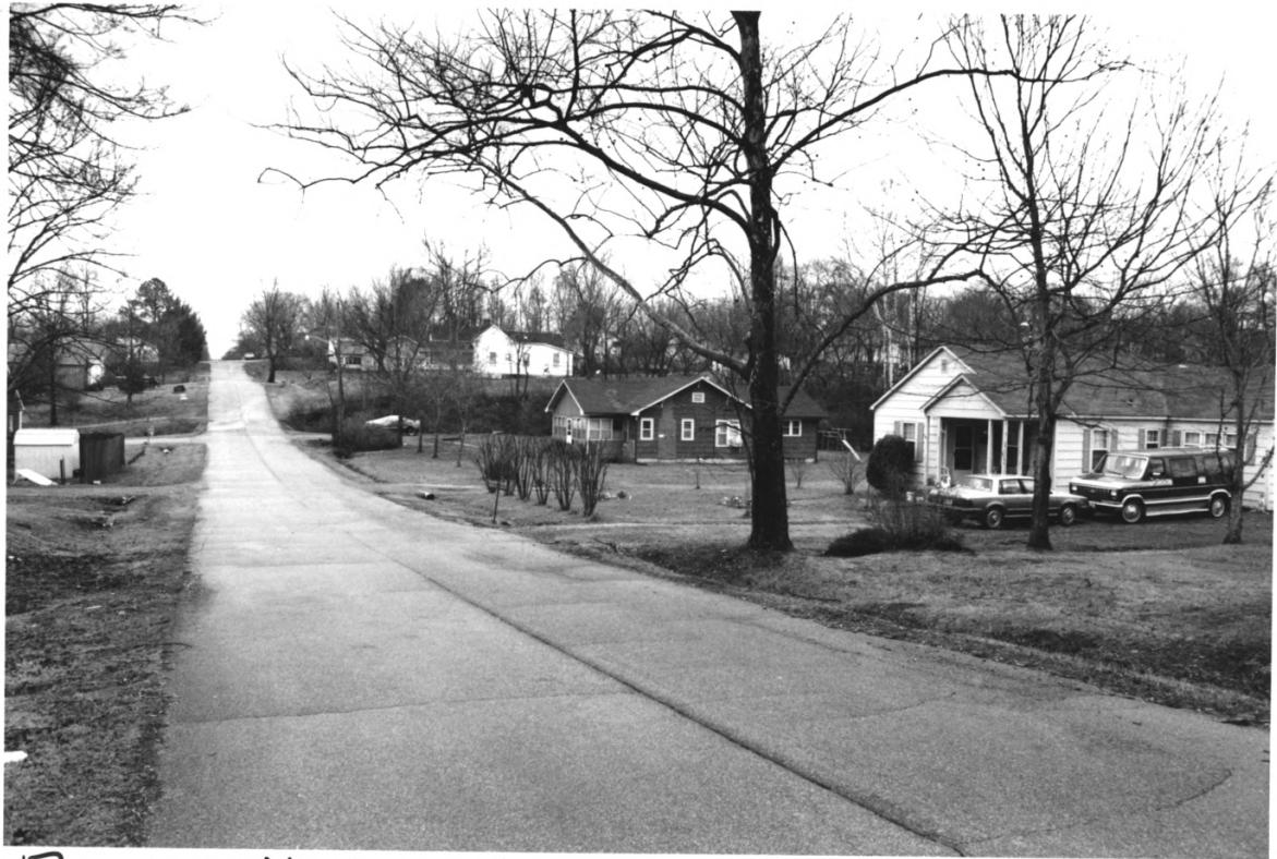
Edowah Historic District McMinn County TN
