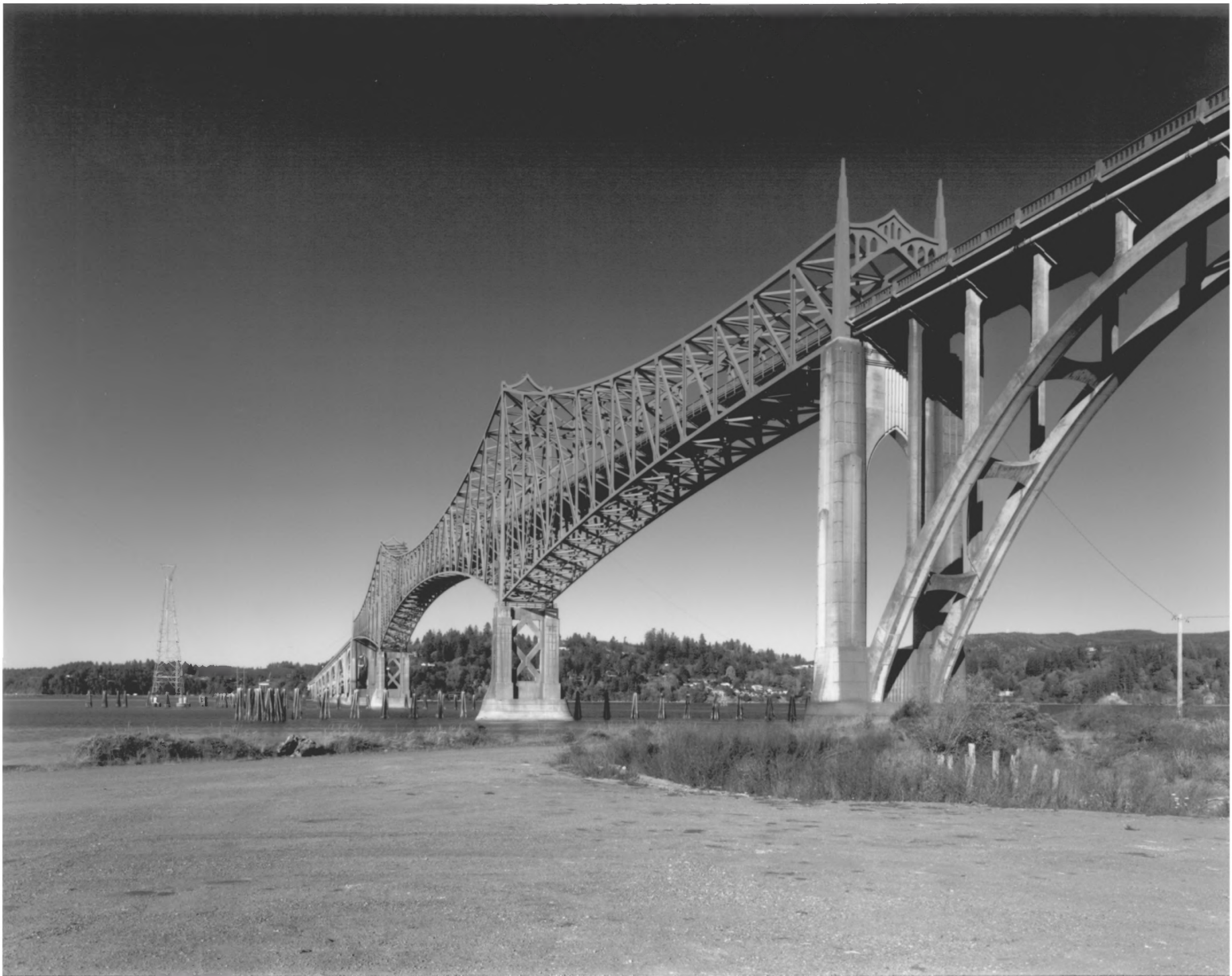
COOS BAY BRIDGE, COOS BAY, OREGON #16
