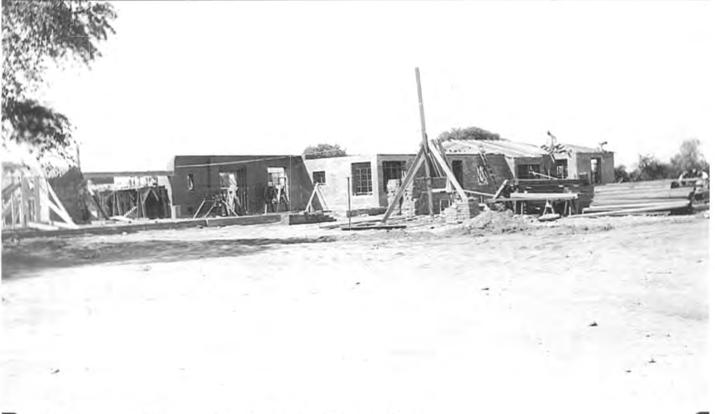
Figure 3. el chaparral under construction, 1937. Courtesy of Hulburd Family.
