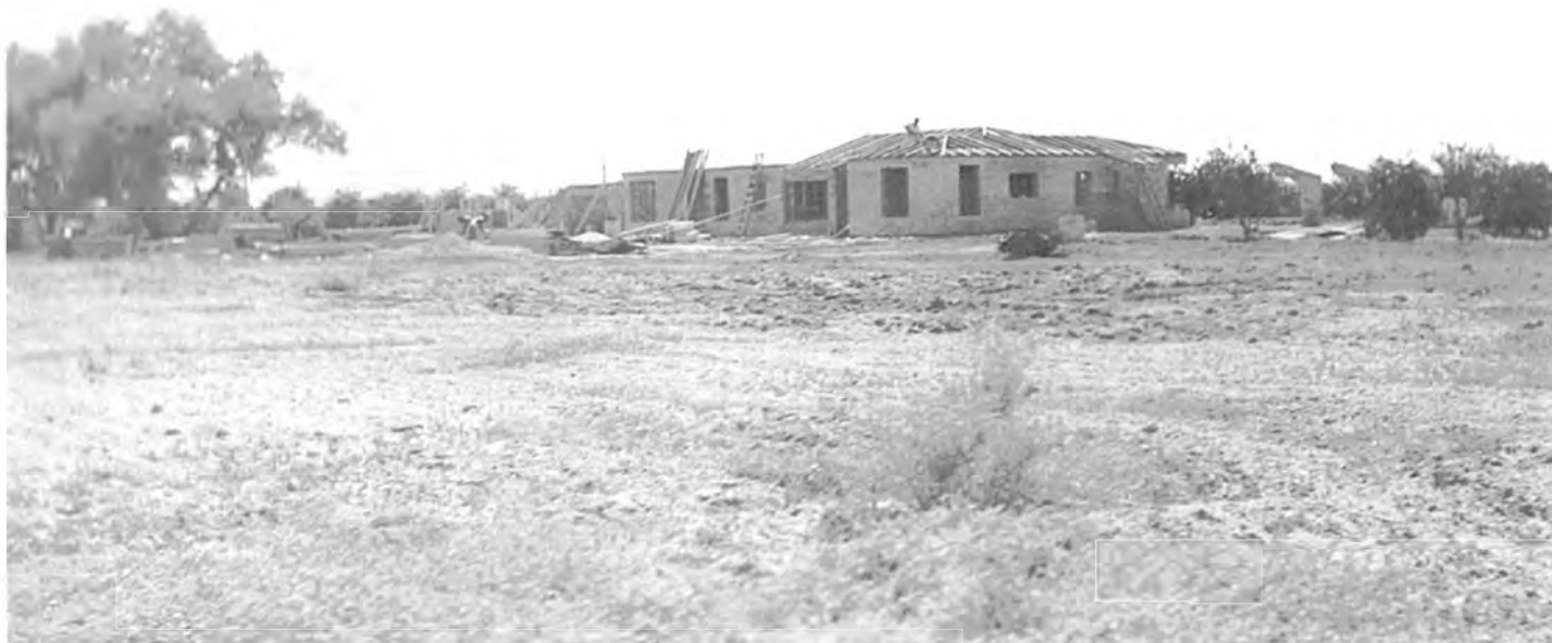
Figure 4. el chaparral under construction, 1937. Courtesy of Hulburd Family.
