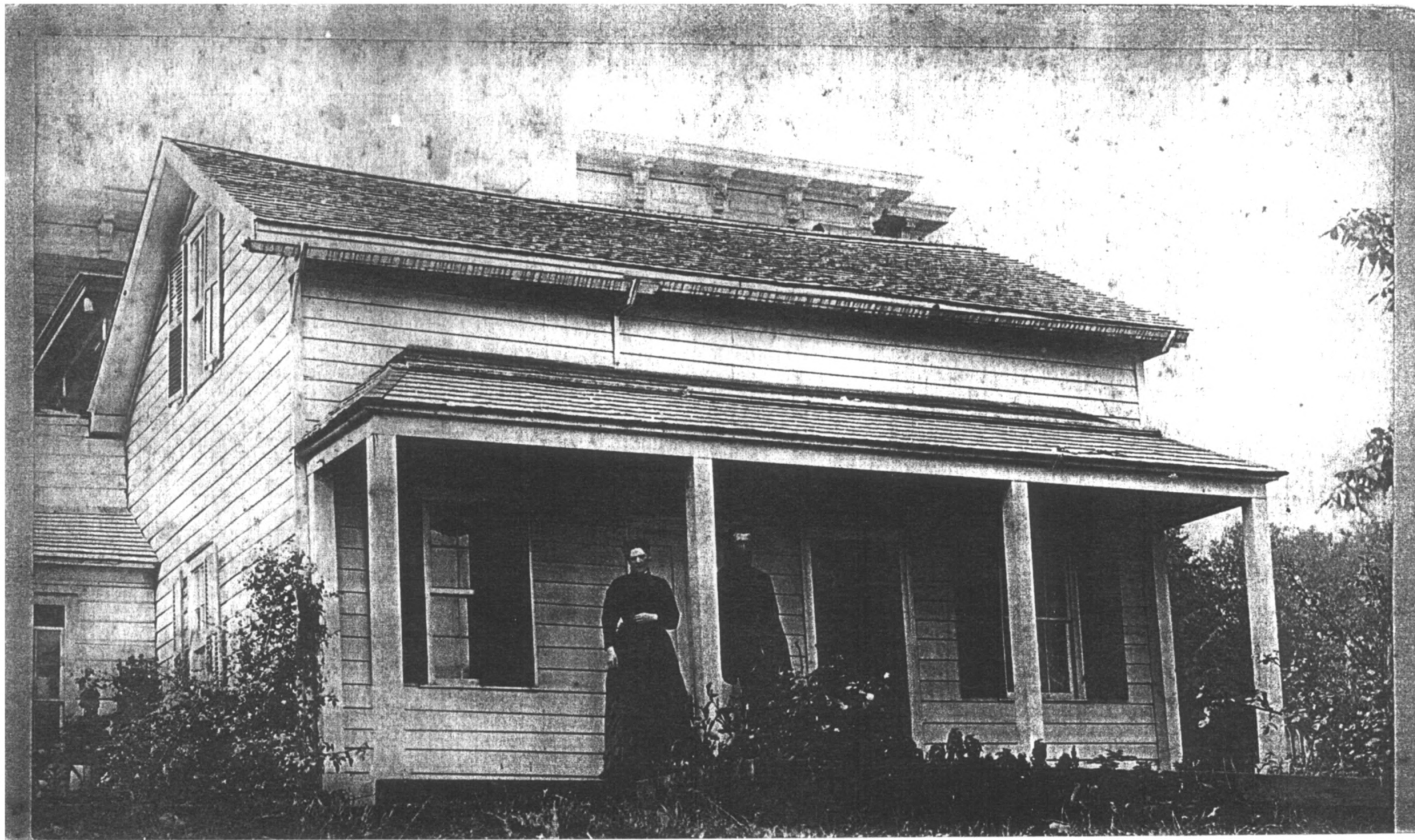
Christian and Mary Leinenweber stand on the porch of Truman Powers' house. The photo was taken in 1883 after the death of Truman Powers. Mary is wearing mourning clothes for her father. The bracketed frieze of the Leineweber's house can be seen in the background. The primed brackets, unpainted siding and missing downspout all indicate the large house addition is in progress.
