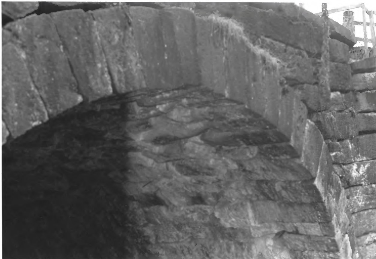
WABASH AND ERIE CANAL CULVERT
