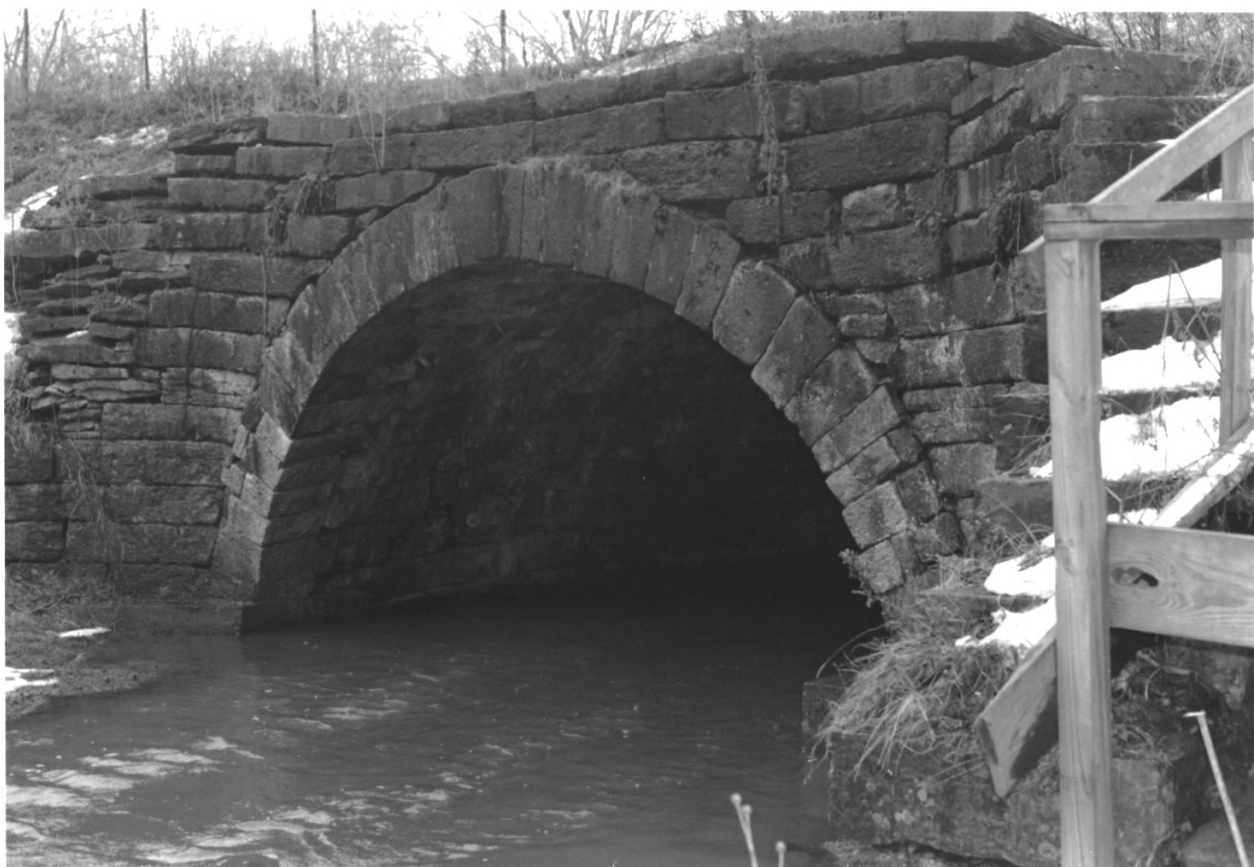
WABASH AND ERIE CANAL CULVERT
