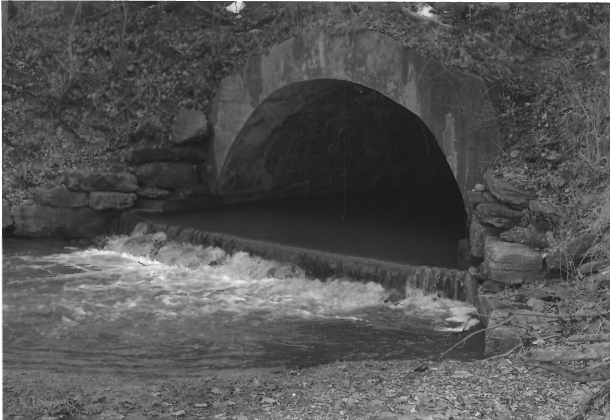
WABASH AND ERIE CANAL CULVERT CARROLL CO., INDIANA 1A
