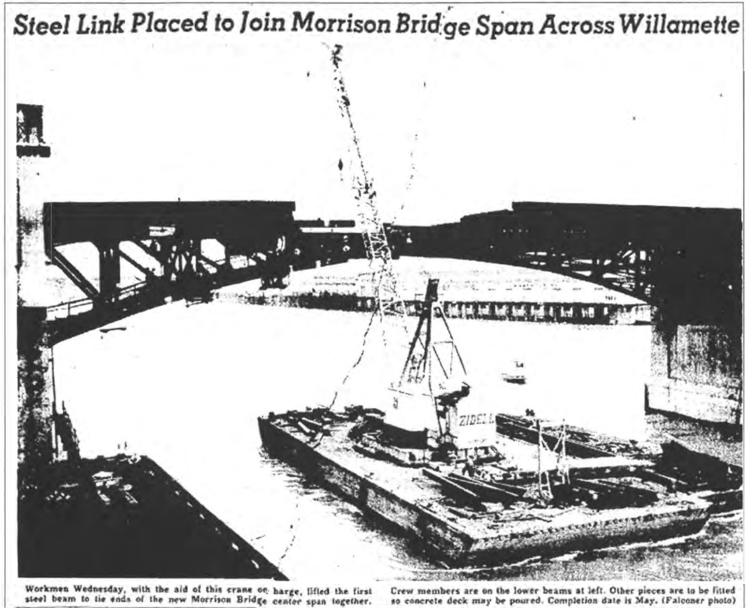
Figure 7: Newspaper Excerpt, Steel Link Placed to Join Morrison Bridge Span Across the Willamette Oregonian , 20-February-1958, 5:1-5
