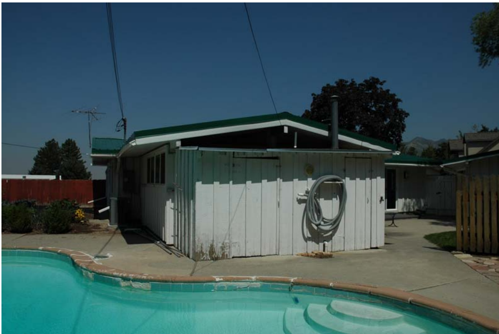
Photograph 4 Southeast elevation of Bourne House, attached shed. Camera facing north.
