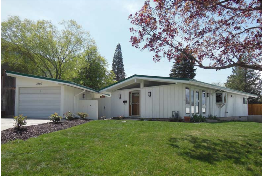
Photograph 1 North and west elevations of Bourne House and garage. Camera facing south.
