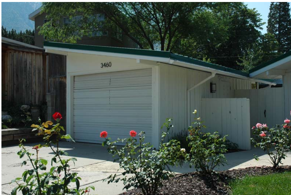
Photograph 8 North and west elevations of garage. Camera facing southeast.
