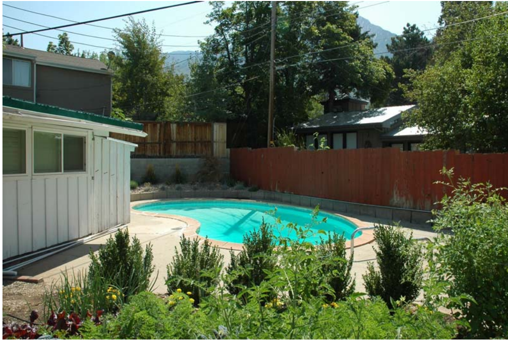
Photograph 5 South elevation of Bourne House with pool. Camera facing southeast.
