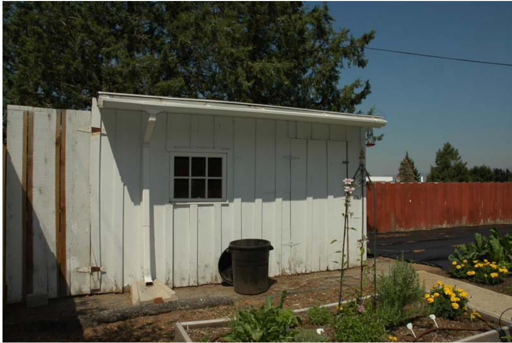
Photograph 9 East elevation of pool house-shed. Camera facing west.
