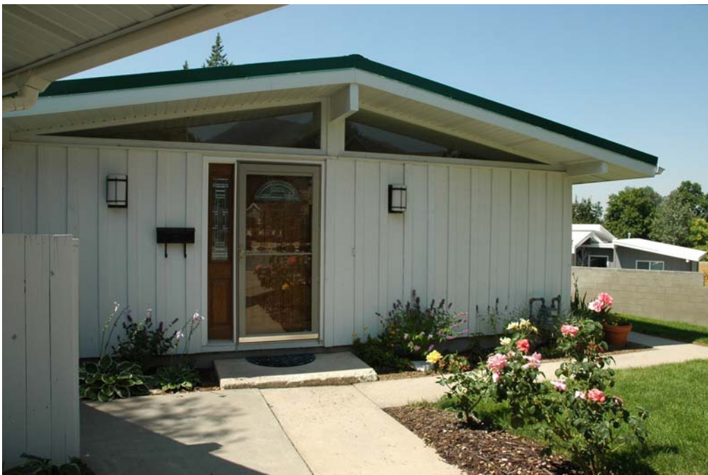
Photograph 2 Northeast elevation of Bourne House. Camera facing southwest.
