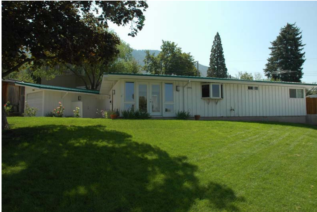
Photograph 7 West elevation of house. Camera facing southeast.
