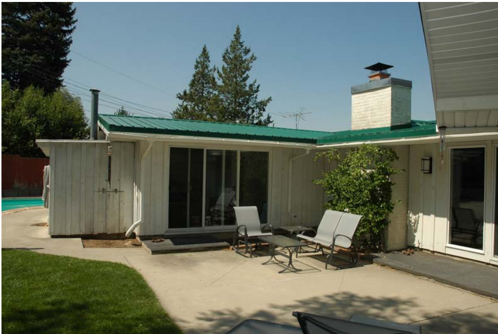
Photograph 3 North and east elevations of Bourne House, patio. Camera facing south.
