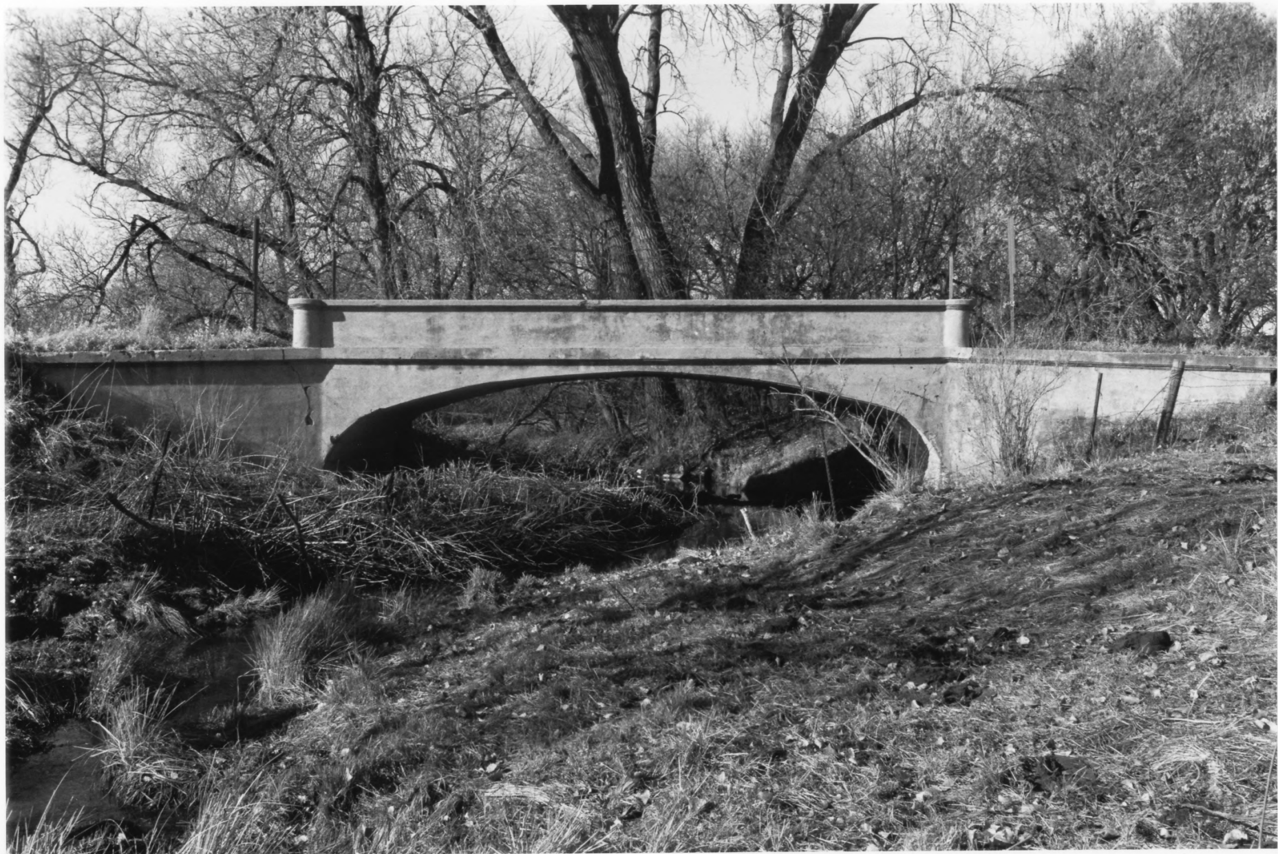
BRIDGE NO. L-4646 ROCK CO., MN PHOTO I.D. 09169#5
