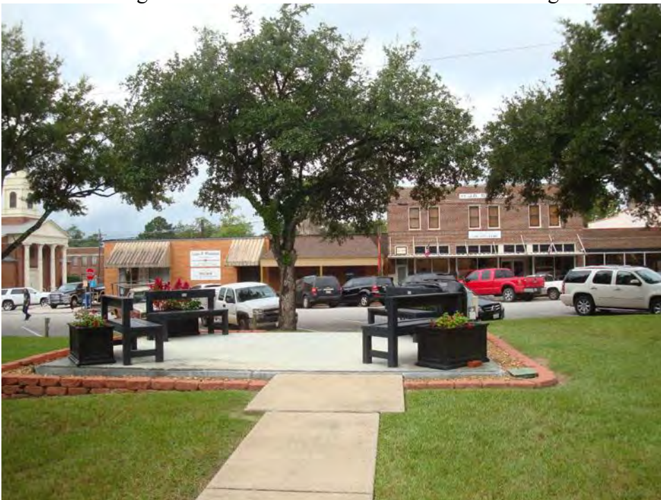
TX_Tyler County_Tyler County Courthouse_0012.tif Noncontributing foundation of the domino hall. Camera facing west.
