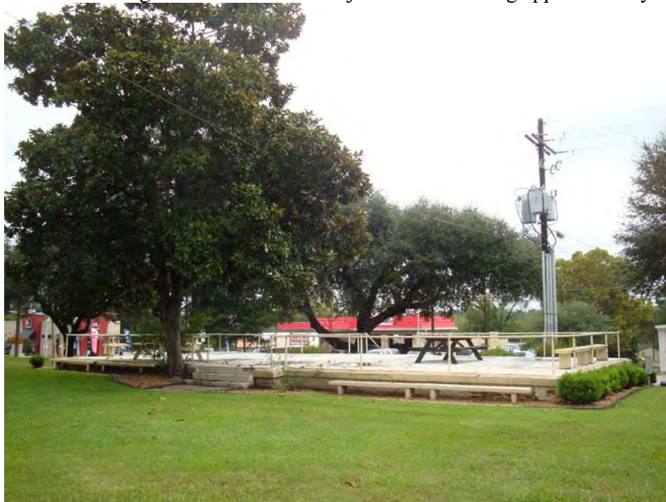
TX_Tyler County_Tyler County Courthouse_0013.tif Noncontributing foundation of the old jail. Camera facing approximately east.
