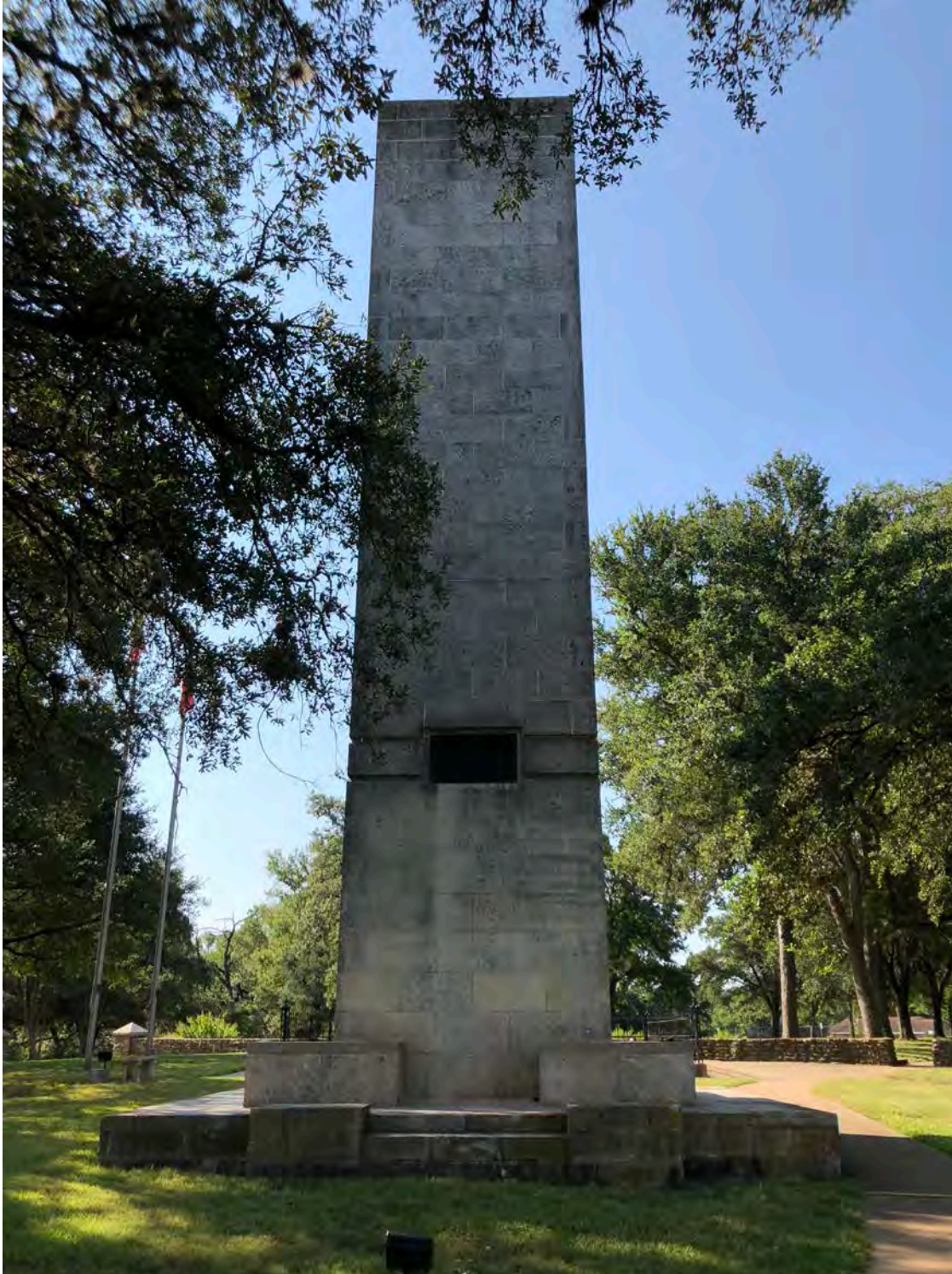
Photo 13: Centennial Monument rear elevation—camera facing southeast.
