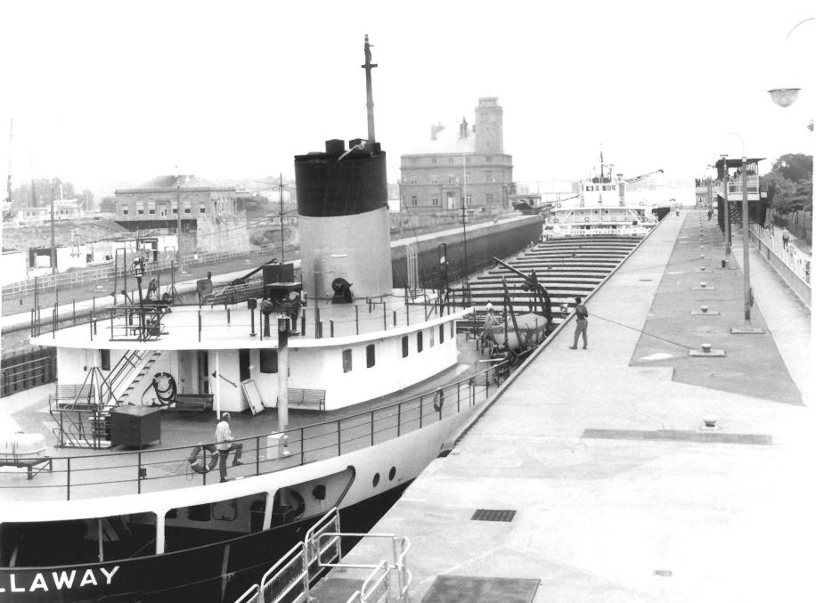
The ore boat in the lock. The lock's water leveliis being reduced to that of Lake Huron.
