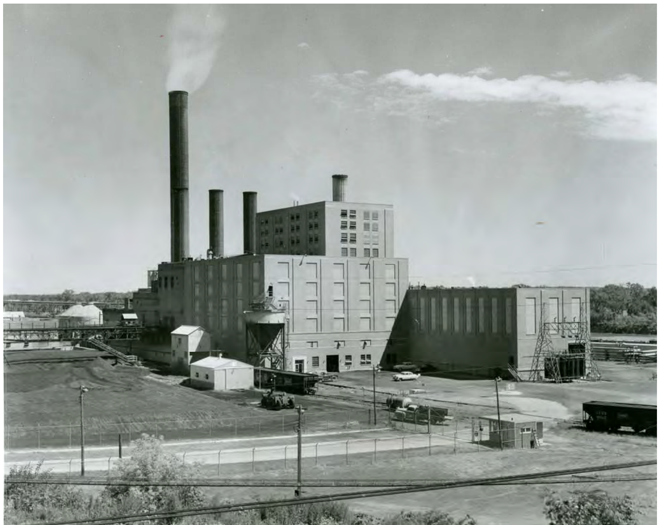
Figure 17: Omaha Power Plant. April 1973. Kriss and McCallum photographers. Image courtesy of Omaha Public Power District.
