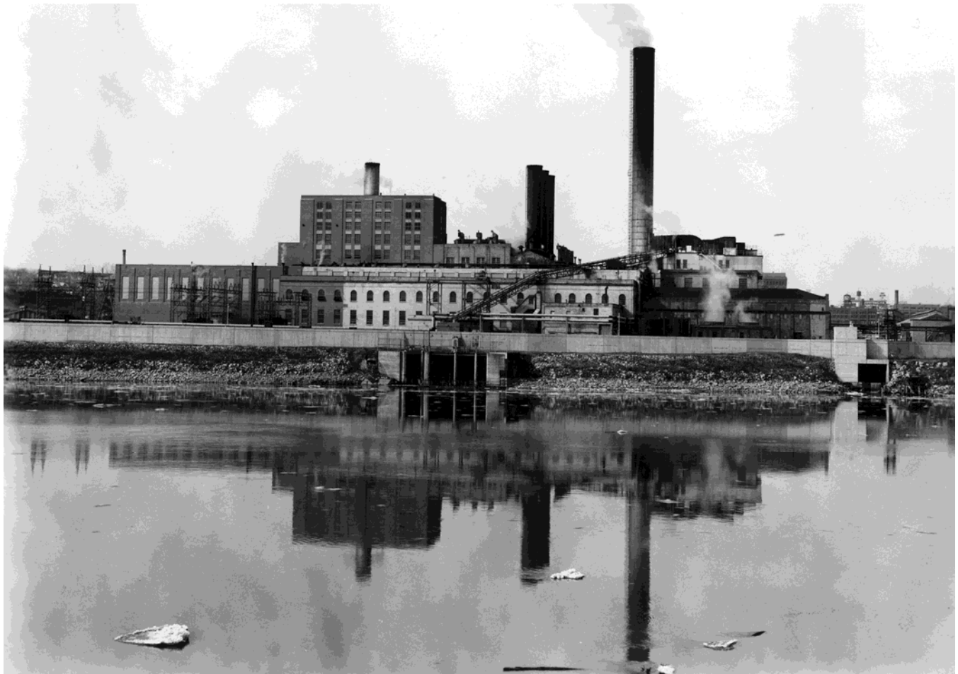
Figure 15: Omaha Power Plant. 1951 c. Ernest Bihler photographer. Image courtesy of Omaha Public Power District.
