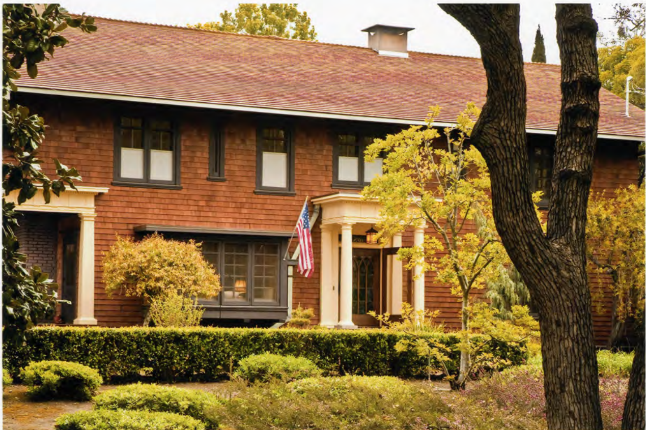
CA_LA County_Merwin House_0003
