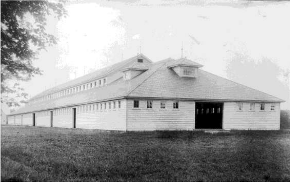
Yearling barn, west end and north eave wall, ca.1920
