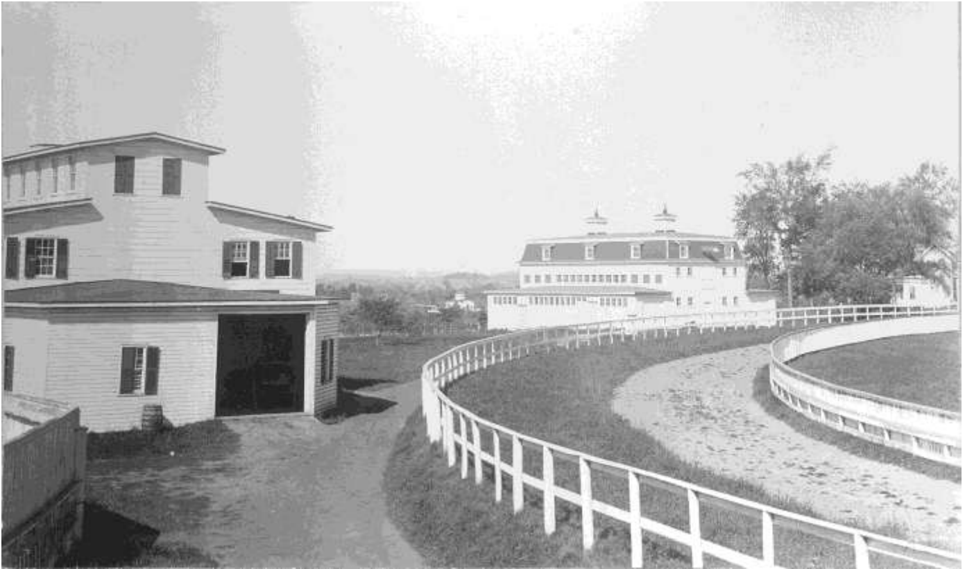
“Broodmare Barn at Turn #1”: Broodmare Barn, left, and Winter Stallion Barn, right, at Turn #1, ca.1920, camera facing WNW
