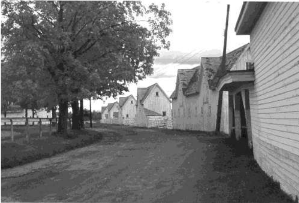
East-West Lane from tool shed looking towards Farm Barn at east end, ca.1950, camera facing east
