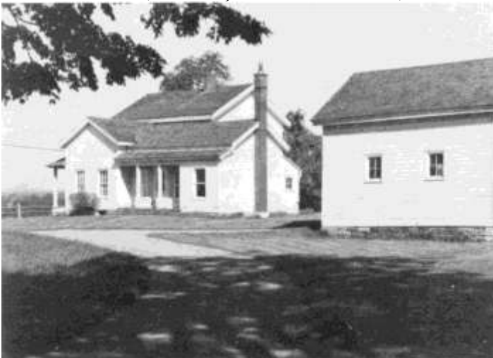
Caretaker's House, south side, camera facing NW
