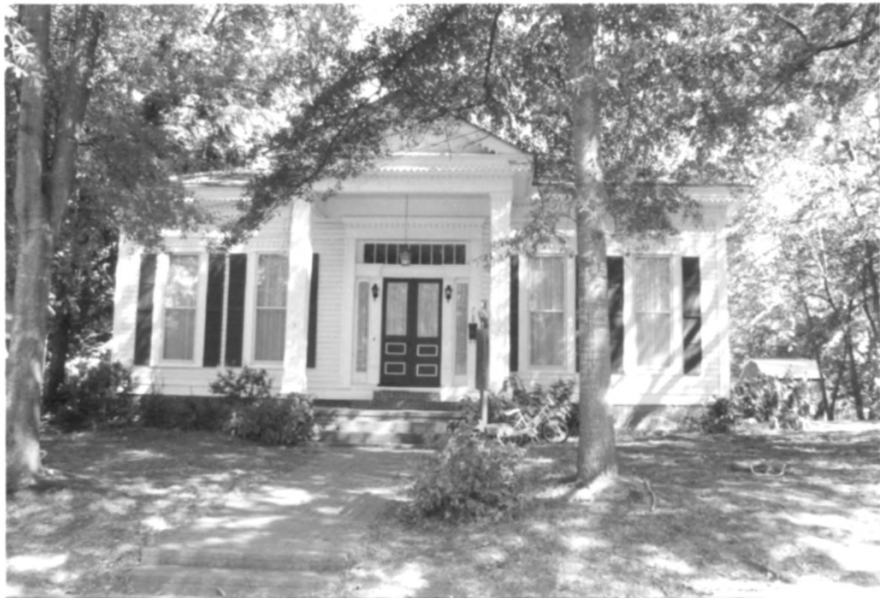
4) Fish Pond House, Corinth Battlefield Corinth, Mississippi Front Facade, view looking east Paul Hawke, Photographer; September 26, 1990
