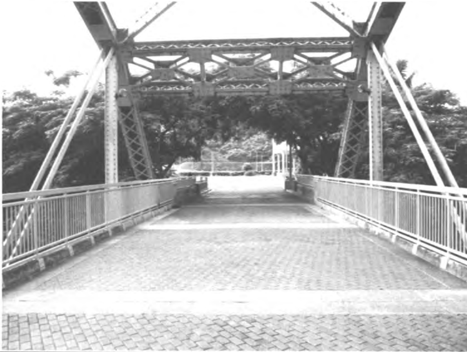
Figure 9. View of pavers used in the bridge's deck.
