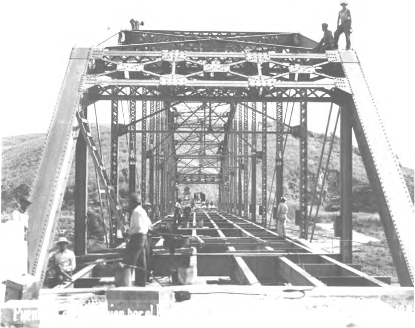
Figure 4. View of the stringers prior to laying the concrete floor, September 14, 1940. Robert R. Prann Collection, Trujillo Alto Bridge, 1939, Contract 120, Archive of Architecture and Construction, University of Puerto Rico.
