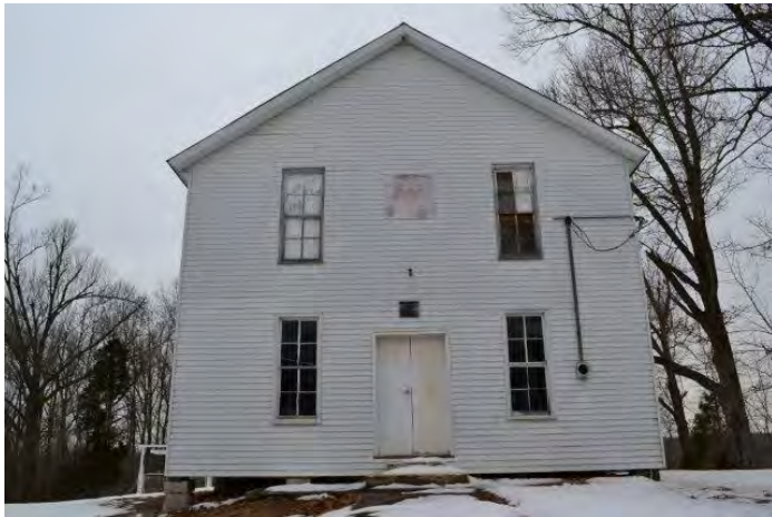
Photo 1: front (southeast) façade
