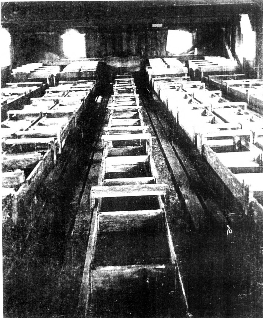
Figure 5. Kettle House Interior. The interior of the Kettle House is shown in this undated photograph labeled on the reverse as "evaporating trays in salt works at South Park." SOURCE: Denver Public Library, Western History and Genealogy Department, image number 4089, Denver, Colorado.
