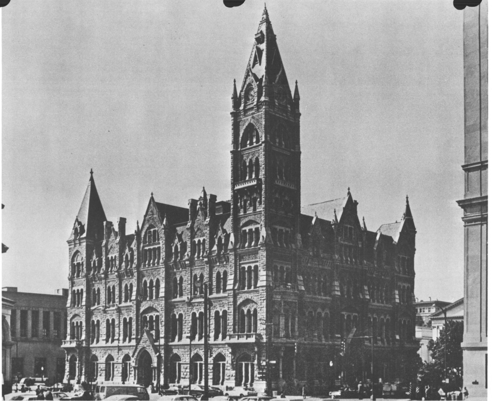
Richmond City Hall, Richmond, Virginia
