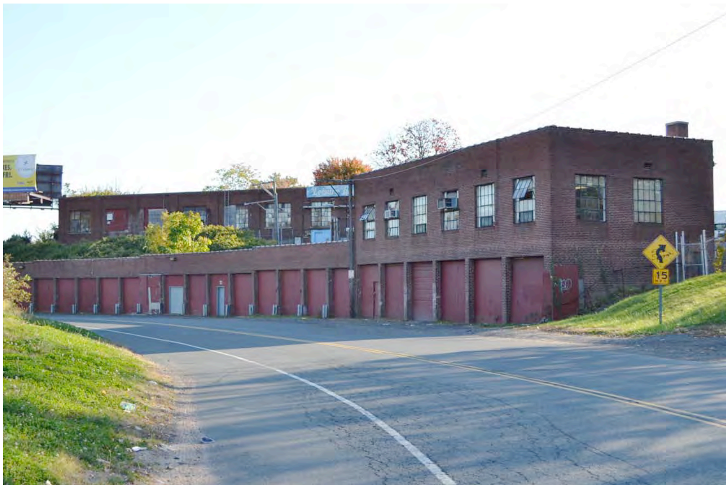
South (side) and east (rear) elevations of 101 Pope Park Highway No. 4 (1930). Camera facing south. Photograph 53 of 58.
