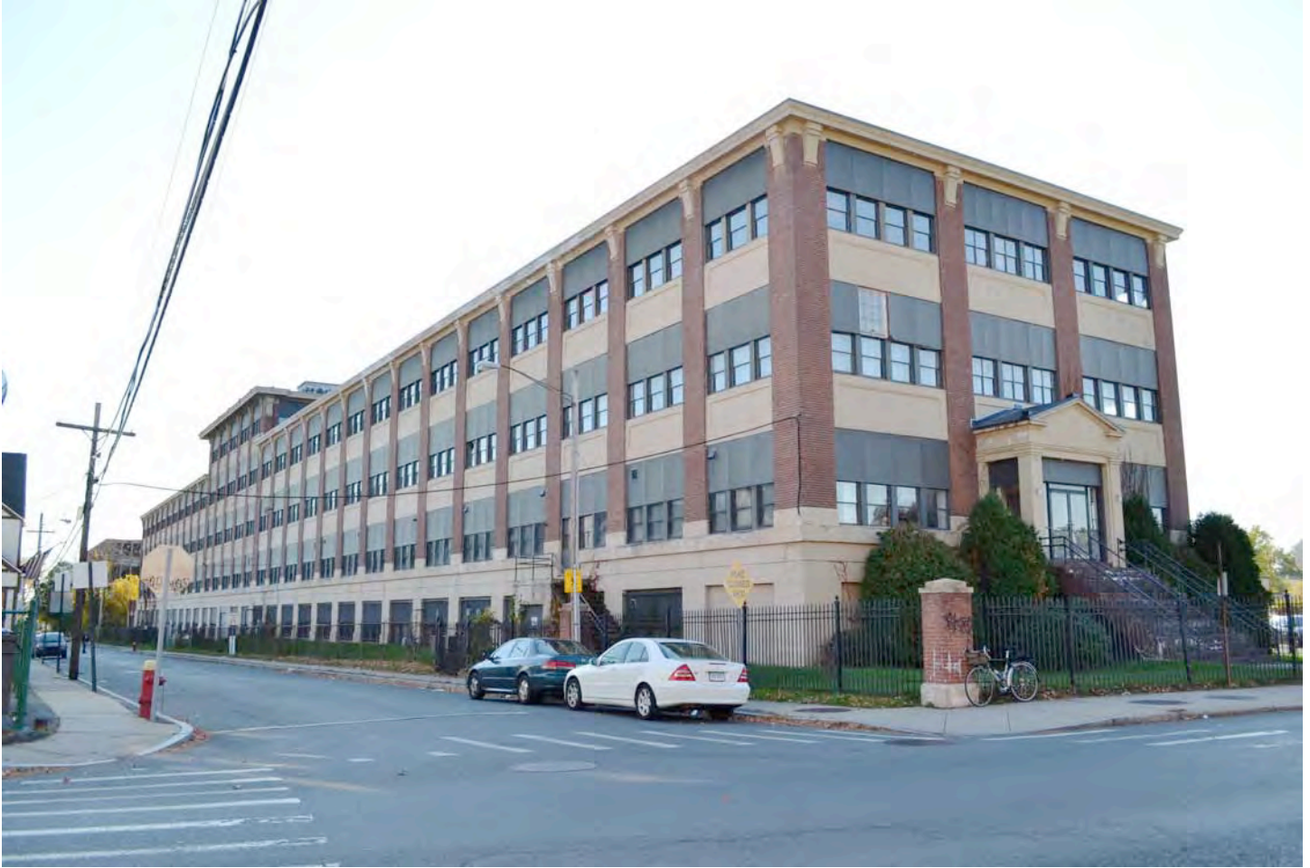
North (front) and east (side) elevations of 237 Hamilton Street (1910, 1915-1916, 1943, and 1951). Camera facing southwest. Photograph 30 of 58.
