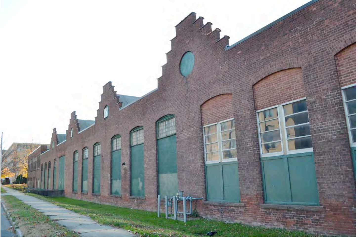
East (side) elevation of 81-99 Bartholomew Avenue (1895). Camera facing southwest. Photograph 28 of 58.
