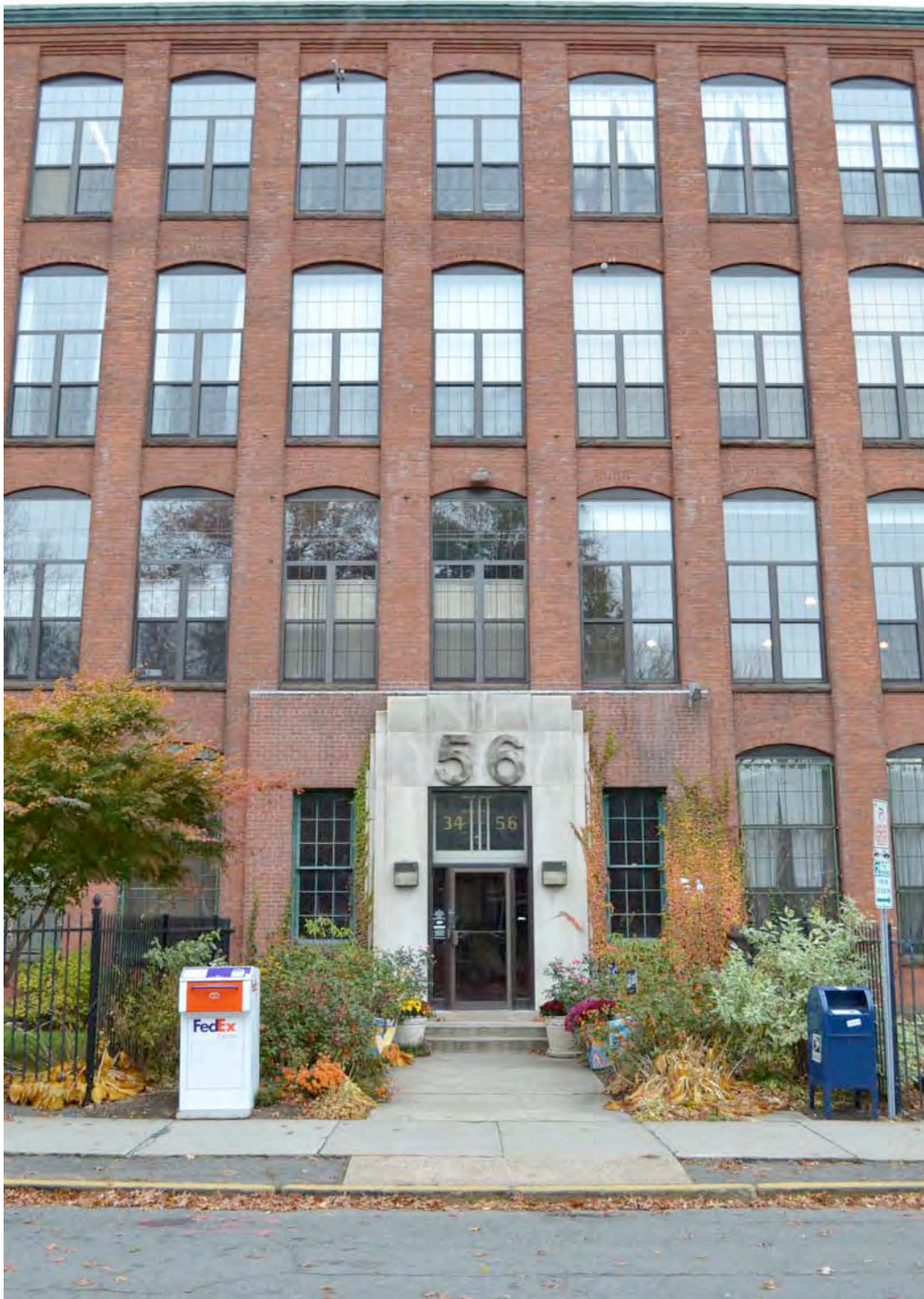
West (front) elevation of 34-56 Arbor Street (1917 and 1936). Camera facing east. Photograph 21 of 58.
