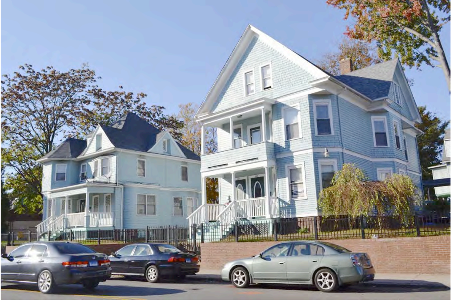
South (front) and east (side) elevations of (from right to left) 1608-1610 and 1618 Park Street (1912 and 1896). Camera facing northwest. Photograph 44 of 58.
