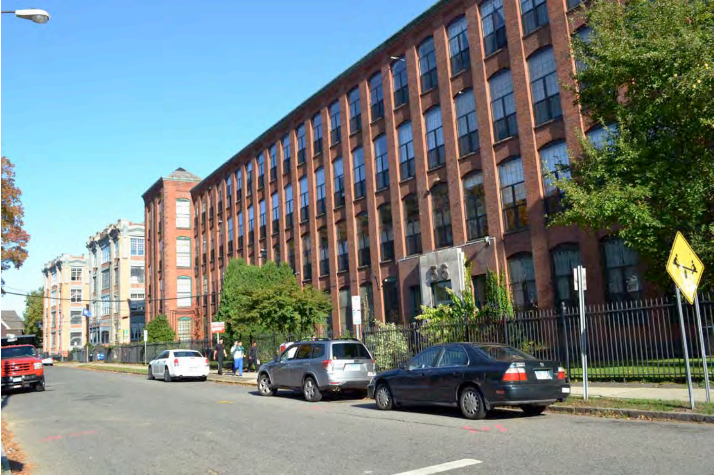
West (front) and south (side) elevations of (from left to right) 16-30 and 34-56 Arbor Street (1912 and 1925, and 1917 and 1936). Camera facing northeast. Photograph 18 of 58.
