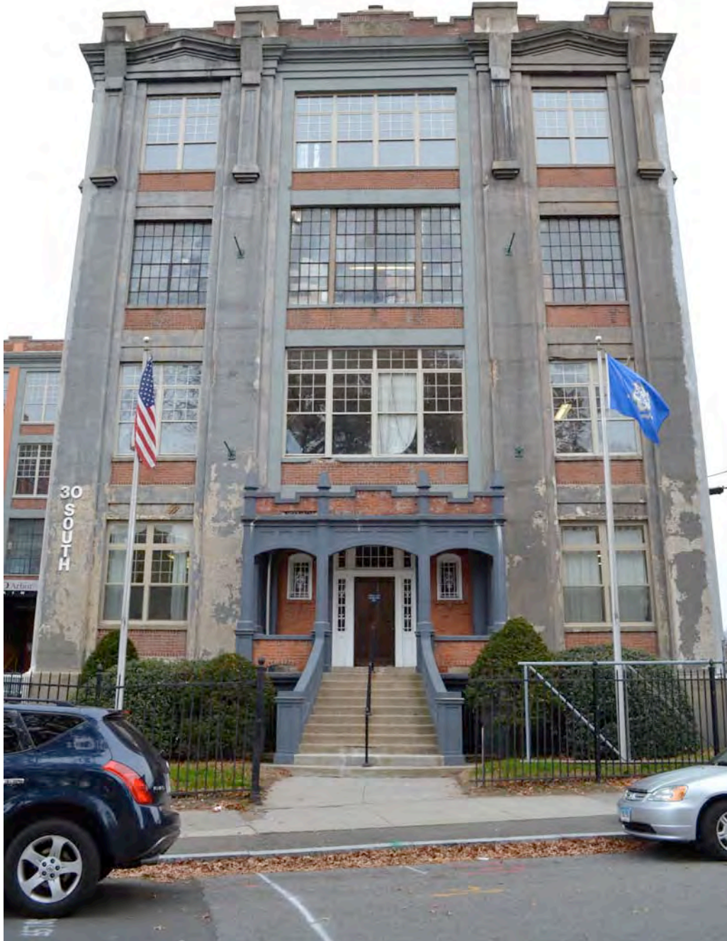
West (front) elevation of 16-30 Arbor Street (1912). Camera facing southeast. Photograph 20 of 58.
