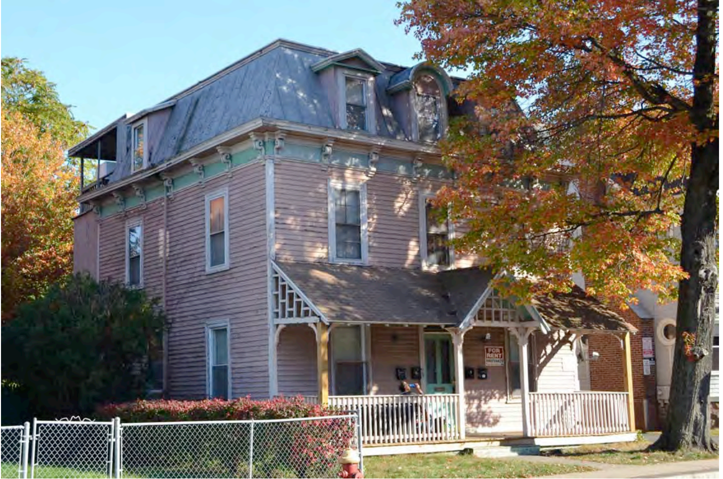
West (front) and north (side) elevations of 34 Sisson Avenue (c. 1885). Camera facing southeast. Photograph 11 of 58.
