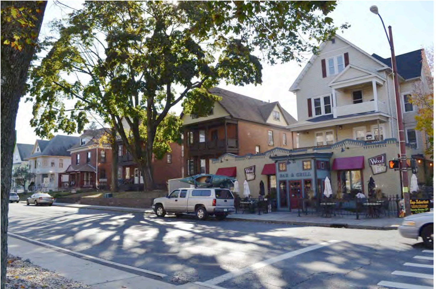
East (front) and north (side) elevations of (from left to right) 77, 79-81, 83-85, 87-89, and 91-99 Sisson Avenue (1898, 1896, 1897, 1909, and 1909/1906). Camera facing southwest. Photograph 4 of 58.
