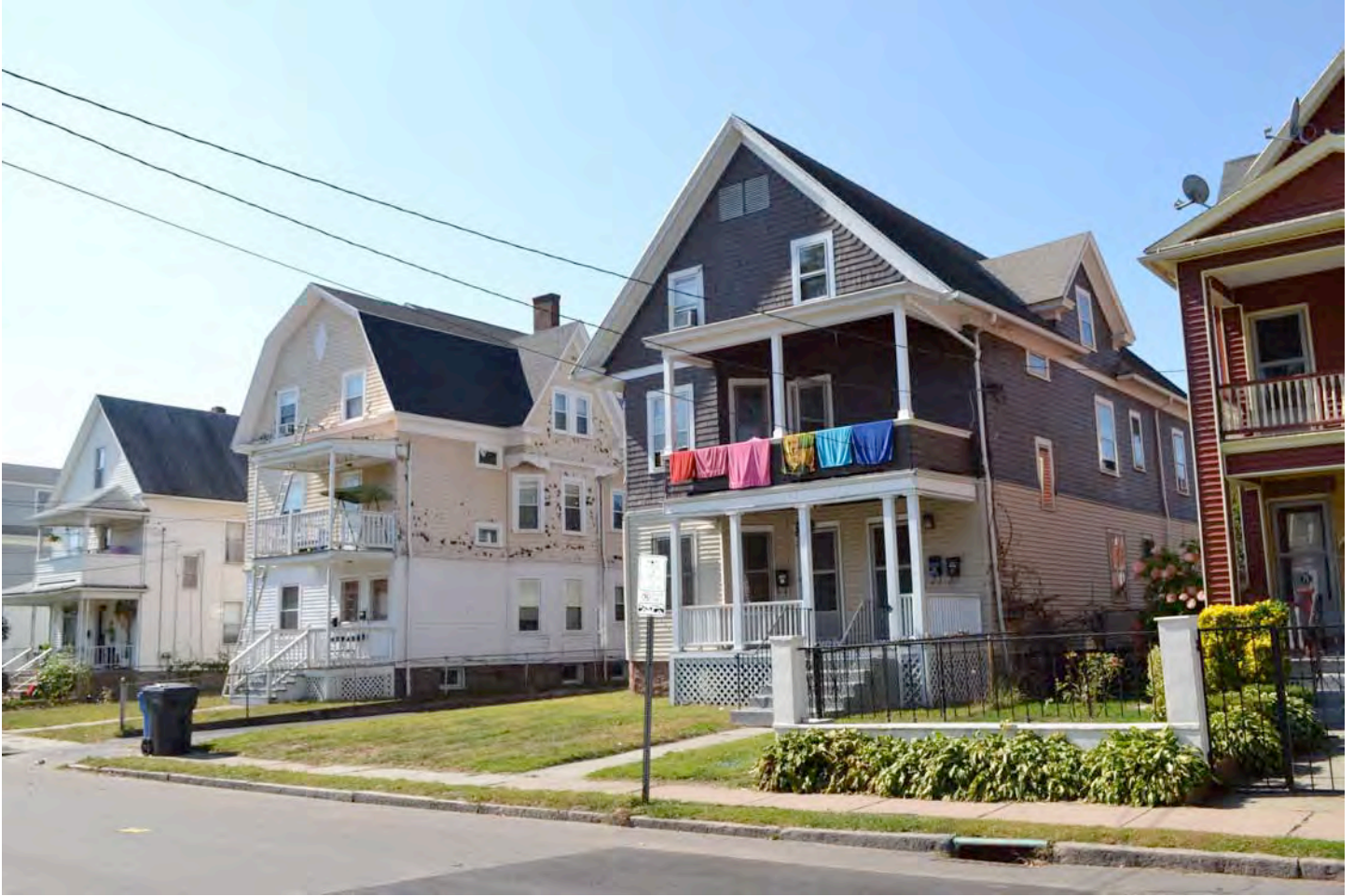
East (front) and north (side) elevations of (from right to left) 59-61, 63-65, and 67-69 Hazel Street (1906, 1906, and 1911). Camera facing southwest. Photograph 13 of 58.
