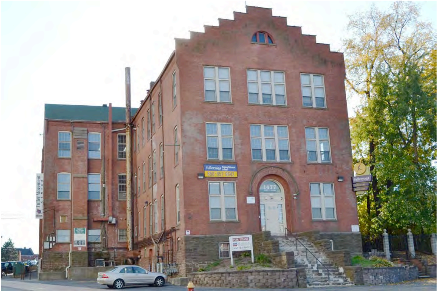
North (front) and east (side) elevations of 1477 Park Street (1895 and 1910). Camera facing southwest. Photograph 24 of 58.
