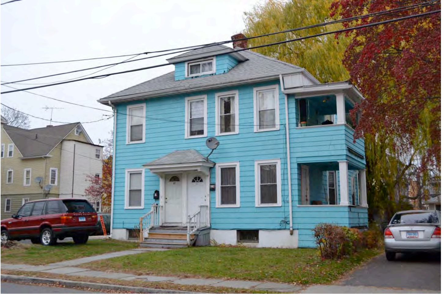
West (front) and south (side) elevations of 82 Hazel Street (1930). Camera facing northeast. Photograph 12 of 58.
