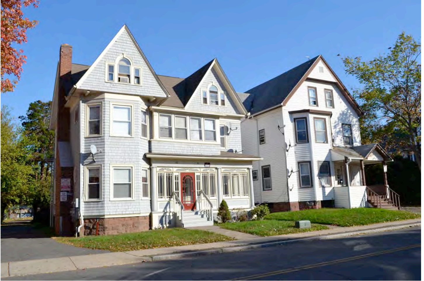
East (front) and north (side) elevations of (from right to left) 26-28 and 30-32 Sisson Avenue (1896 and 1910). Camera facing southeast. Photograph 56 of 58.
