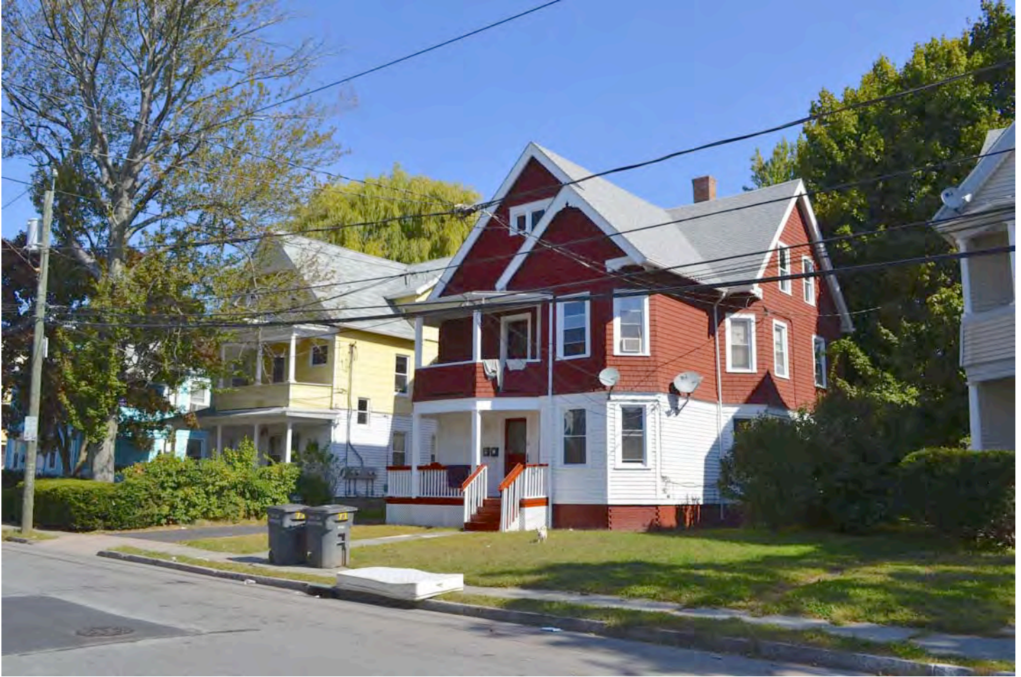
East (front) and north (side) elevations of (from right to left) 72 and 76-78 Hazel Street (1900 and 1902). Camera facing northeast. Photograph 14 of 58.
