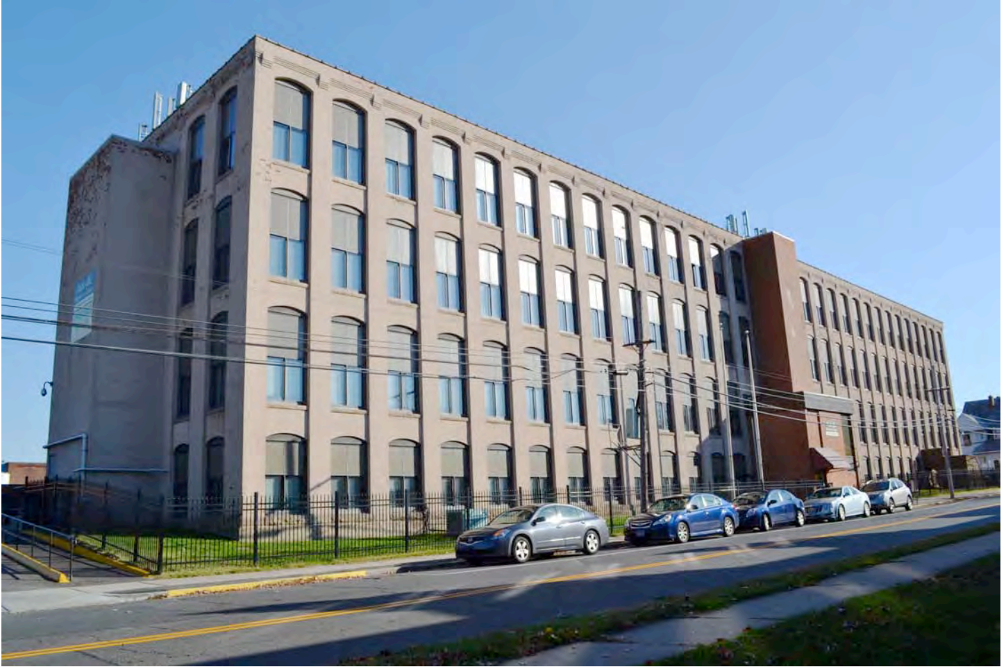
West (front) and north (side) elevations of 110 Bartholomew Avenue (1912, listed in Hartford Assessor's records as 250 Hamilton Avenue). Camera facing southeast. Photograph 29 of 58.
