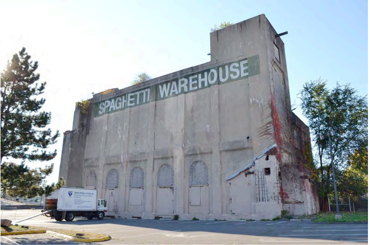
East (front) and north (side) elevations of 45 Bartholomew Avenue (1912). Camera facing southwest. Photograph 27 of 58.
