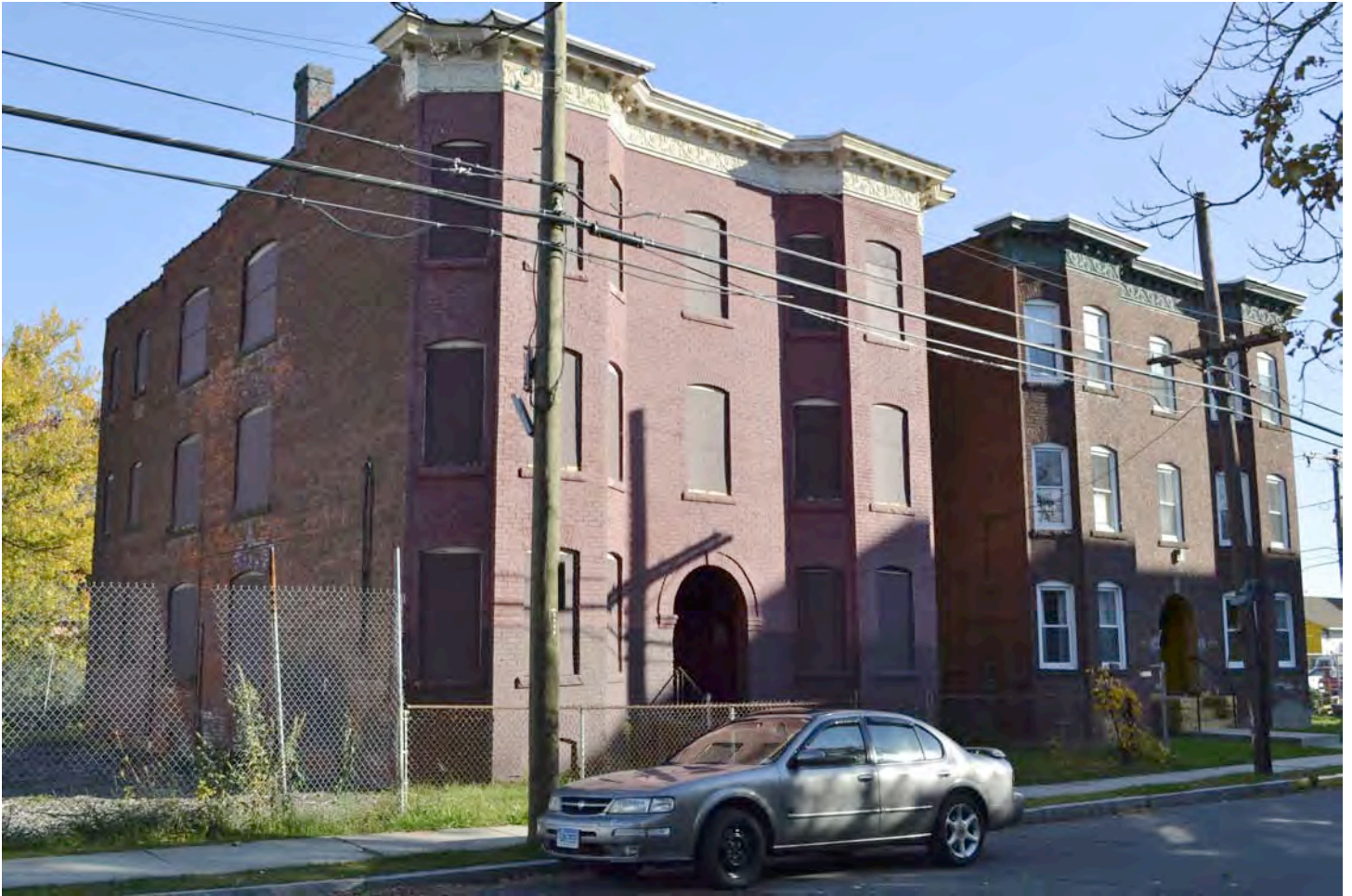
West (front) and north (side) elevations of (from left to right) 160-162 and 164-166 Bartholomew Avenue (1907). Camera facing southeast. Photograph 35 of 58.
