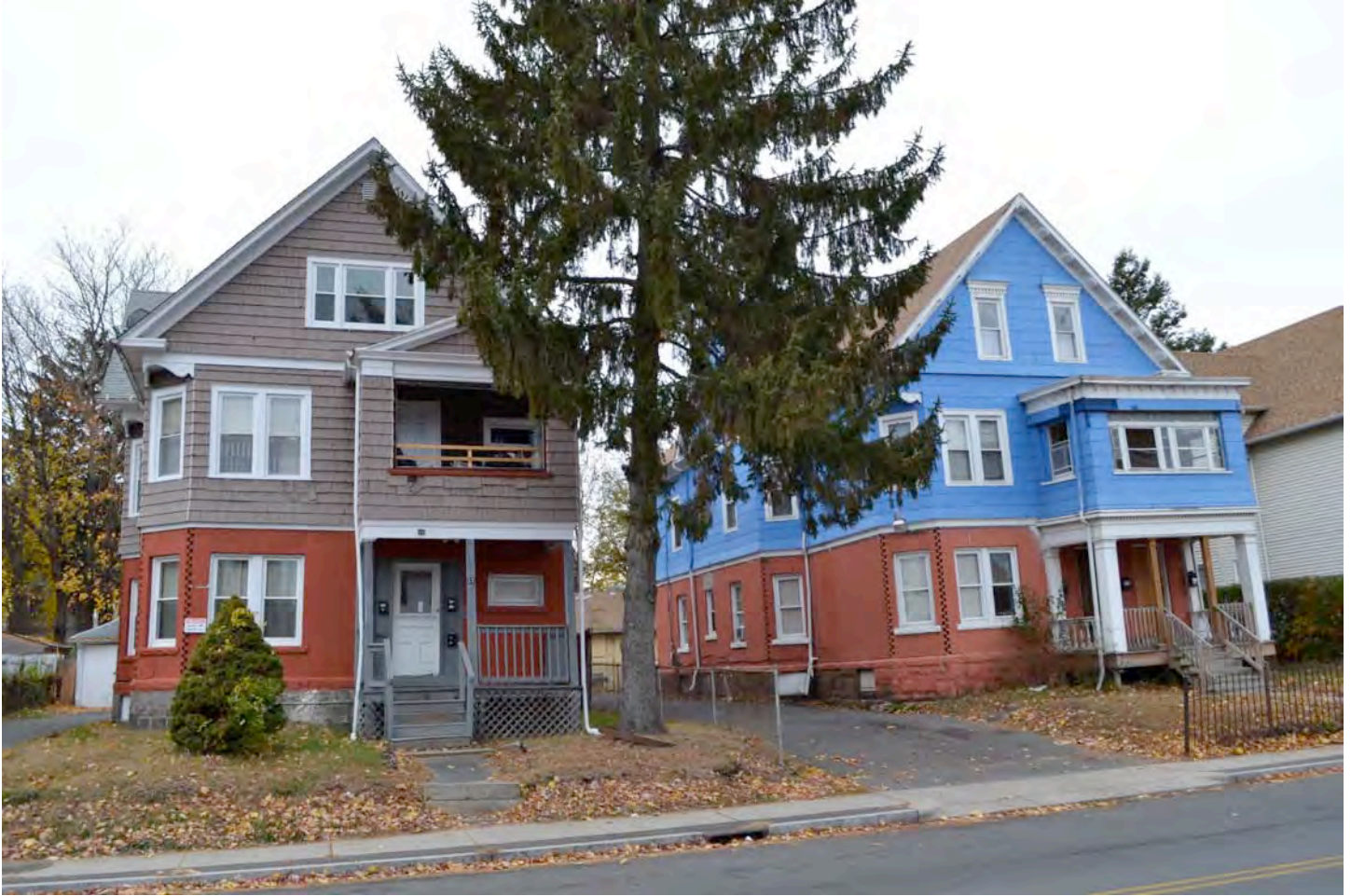
East (front) and south (side) elevations of (from right to left) 57 and 59-61 Sisson Avenue (1902 and 1907). Camera facing northwest. Photograph 8 of 58.
