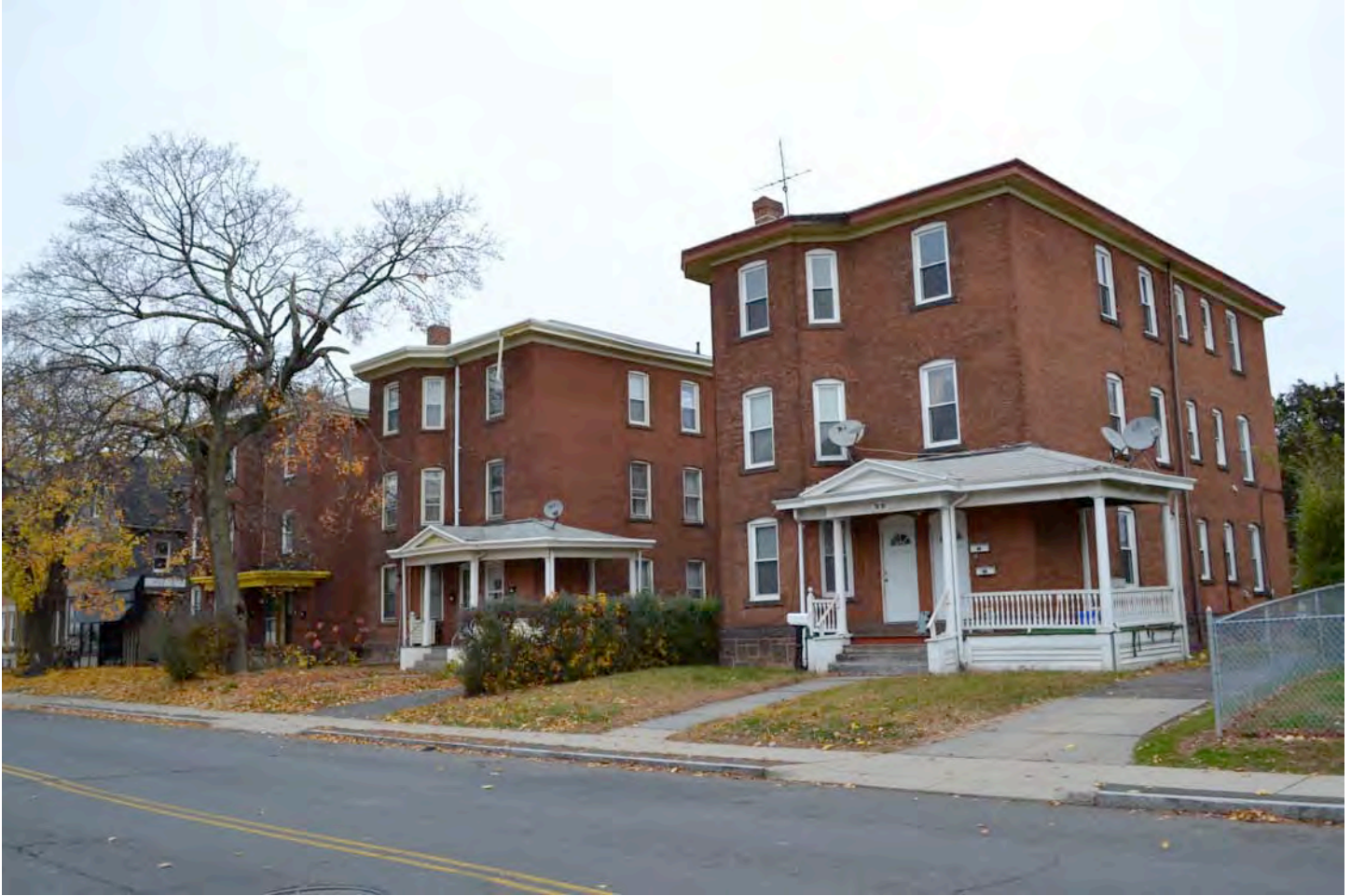
West (front) and south (side) elevations of (from right to left) 74-76 and 78-80 Sisson Avenue (1907 and 1909). Camera facing northeast. Photograph 6 of 58.
