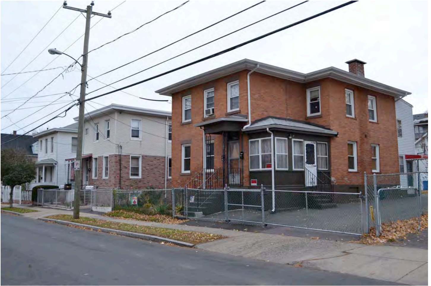
East (front) and north (side) elevations of (from right to left) 105-107, 109-11, and 113 Francis Avenue (c. 1871). Camera facing southwest. Photograph 40 of 58.
