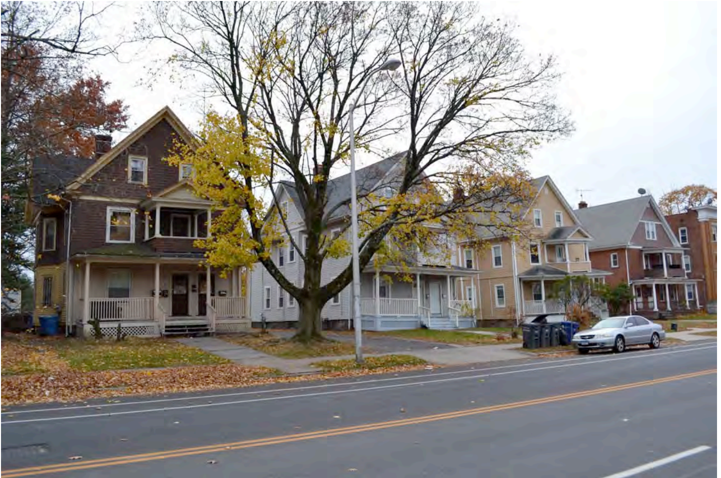
North (front) and east (side) elevations of (from left to right) 867-869, 871-873, 877-879, and 881-883 Capitol Avenue (1910, 1910, 1911, and 1910). Camera facing southwest. Photograph 3 of 58.
