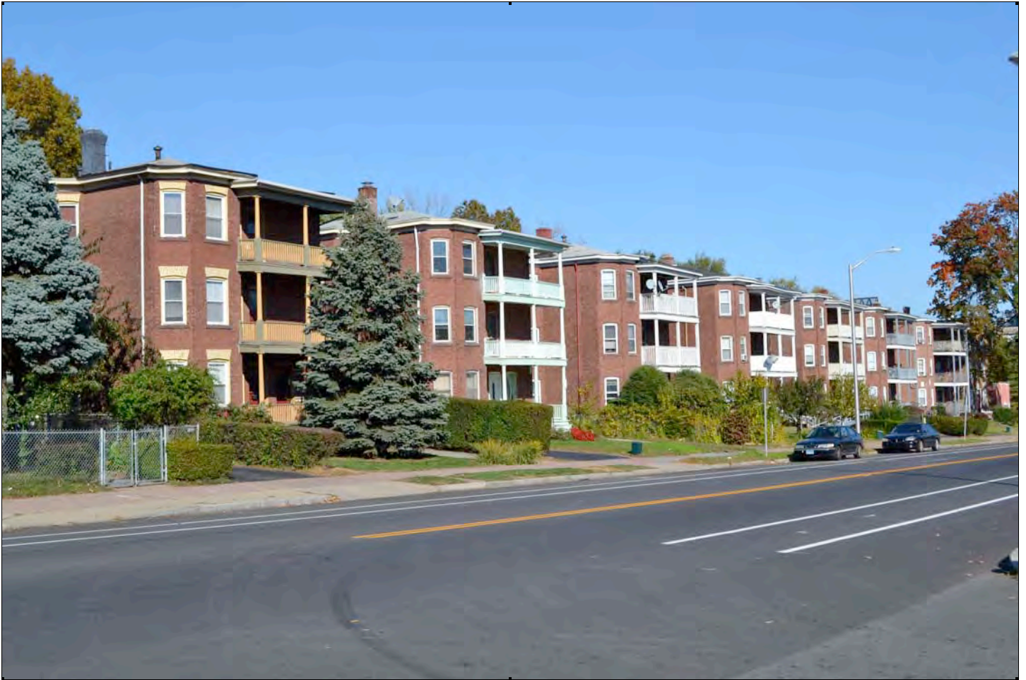
South (front) and west (side) elevations of (from left to right) 788-790, 792-794, 798-800, 804-806, 808-810, 814-816, and 818-820 Capitol Avenue (1911, 1912, 1911, 1910, 1911, 1911, and 1911). Camera facing northeast. Photograph 1 of 58.
