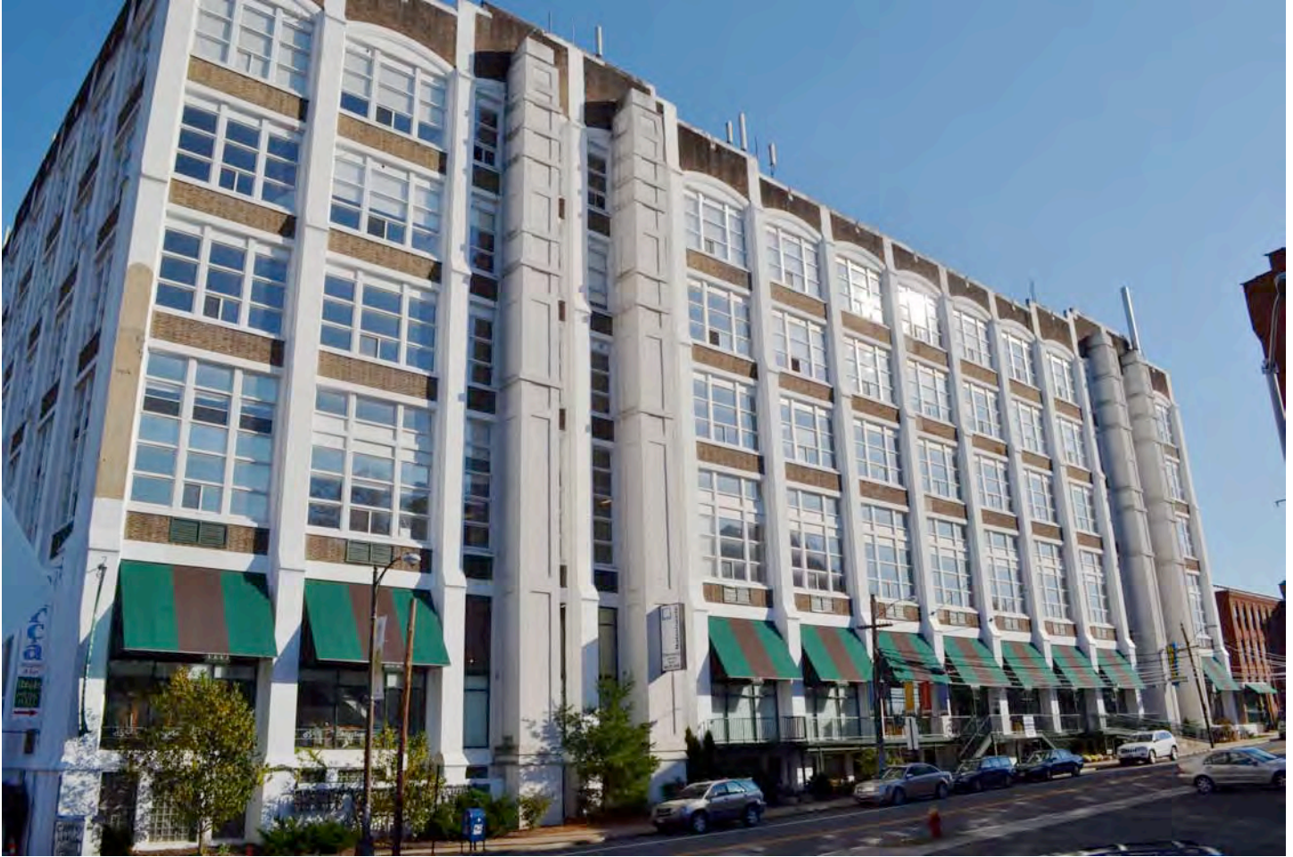
North (front) and west (side) elevations of 1429 Park Street (1920). Camera facing southeast. Photograph 23 of 58.
