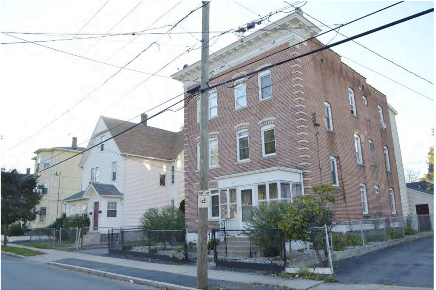
East (front) and north (side) elevations of (from right to left) 133-135, 137-139, and 141-143 Francis Avenue (1913, 1896, 1896). Camera facing southwest. Photograph 41 of 58.
