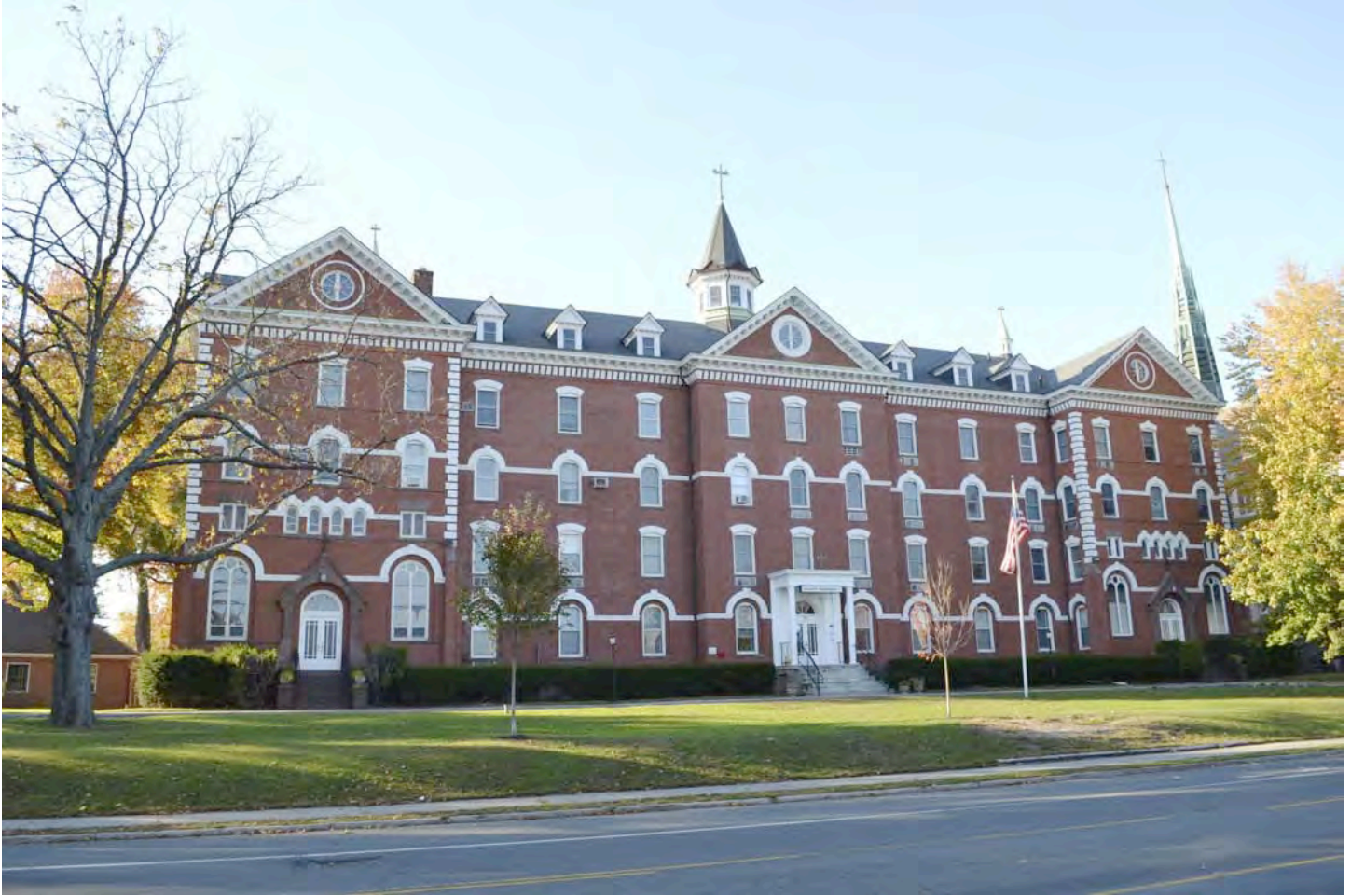
West (front) and south (side) elevations of 85 New Park Avenue (1894 and 1907). Camera facing northwest. Photograph 48 of 58.
