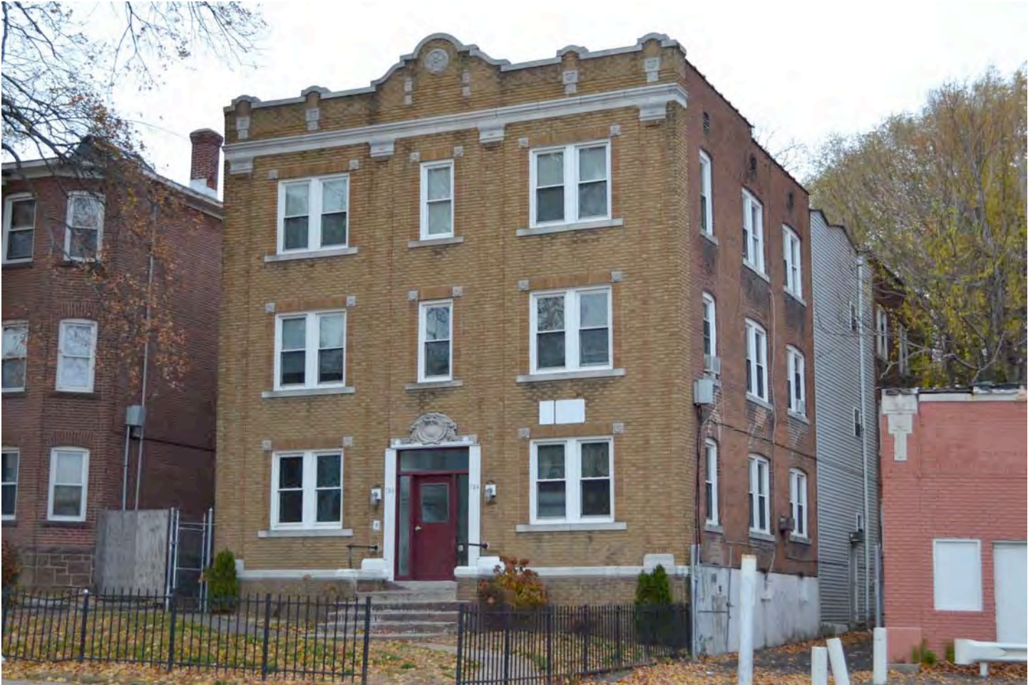
South (front) and east (side) elevations of 784-786 Capitol Avenue (1926). Camera facing northwest. Photograph 52 of 58.
