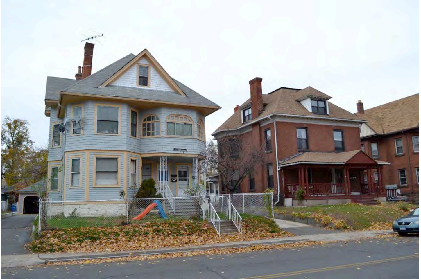
East (front) and south (side) elevations of (from left to right) 79-81 and 83-85 Sisson Avenue (1896 and 1897). Camera facing northwest. Photograph 9 of 58.
