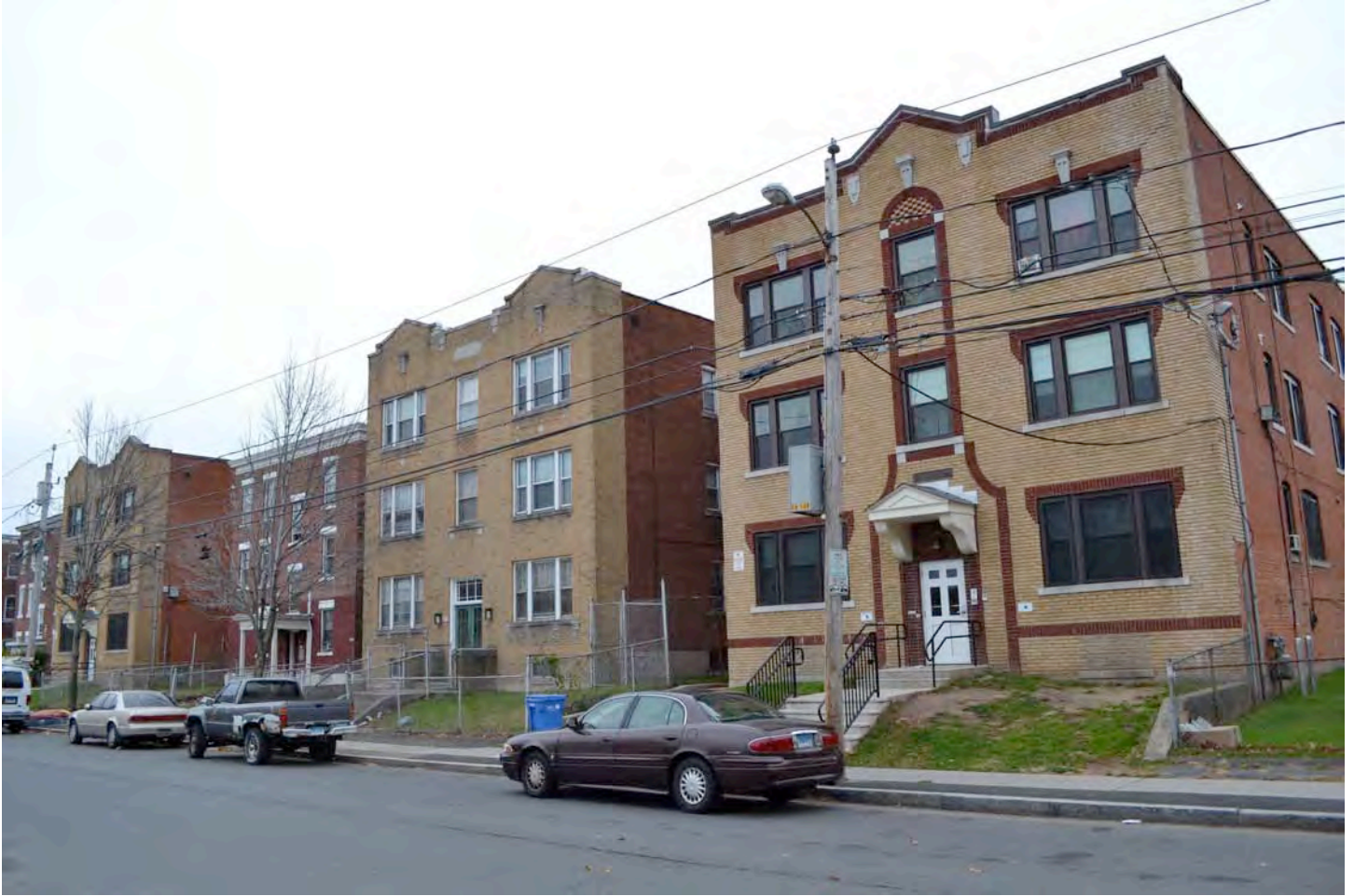
East (front) and north (side) elevations of (from right to left) 31-33, 27-29, 23-25, and 19-21 Orange Street (1924, 1925, 1912, and 1925). Camera facing southwest. Photograph 15 of 58.
