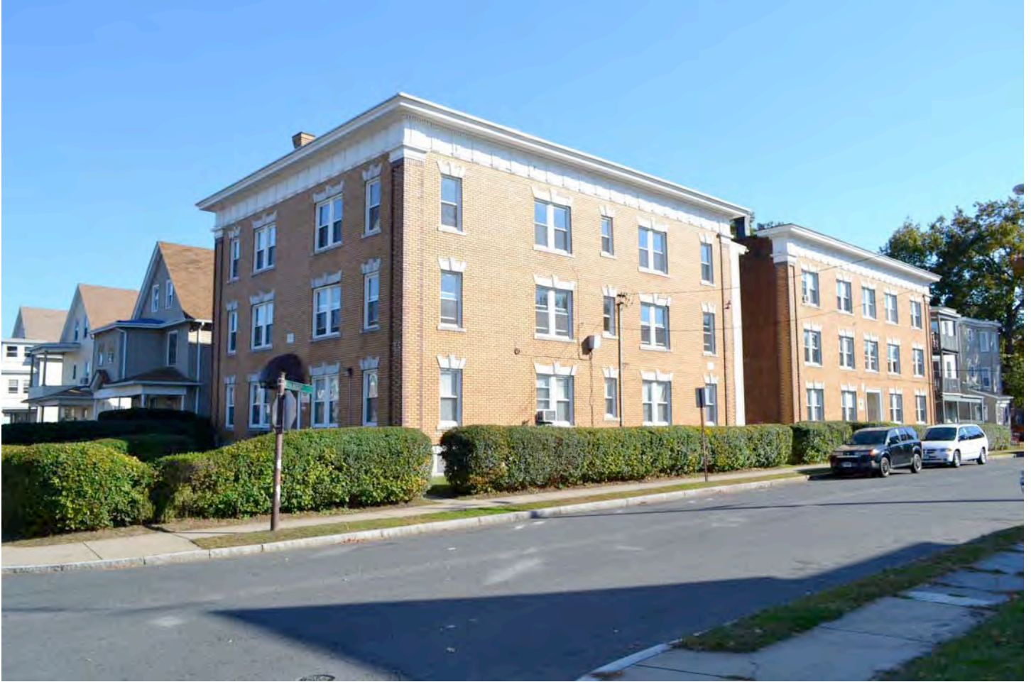
North (front) and west (side) elevations of 821 Capitol Avenue (left, 1915) and west (front) and north (side) elevations of 80 Orange Street (right, 1915). Camera facing southeast. Photograph 57 of 58.
