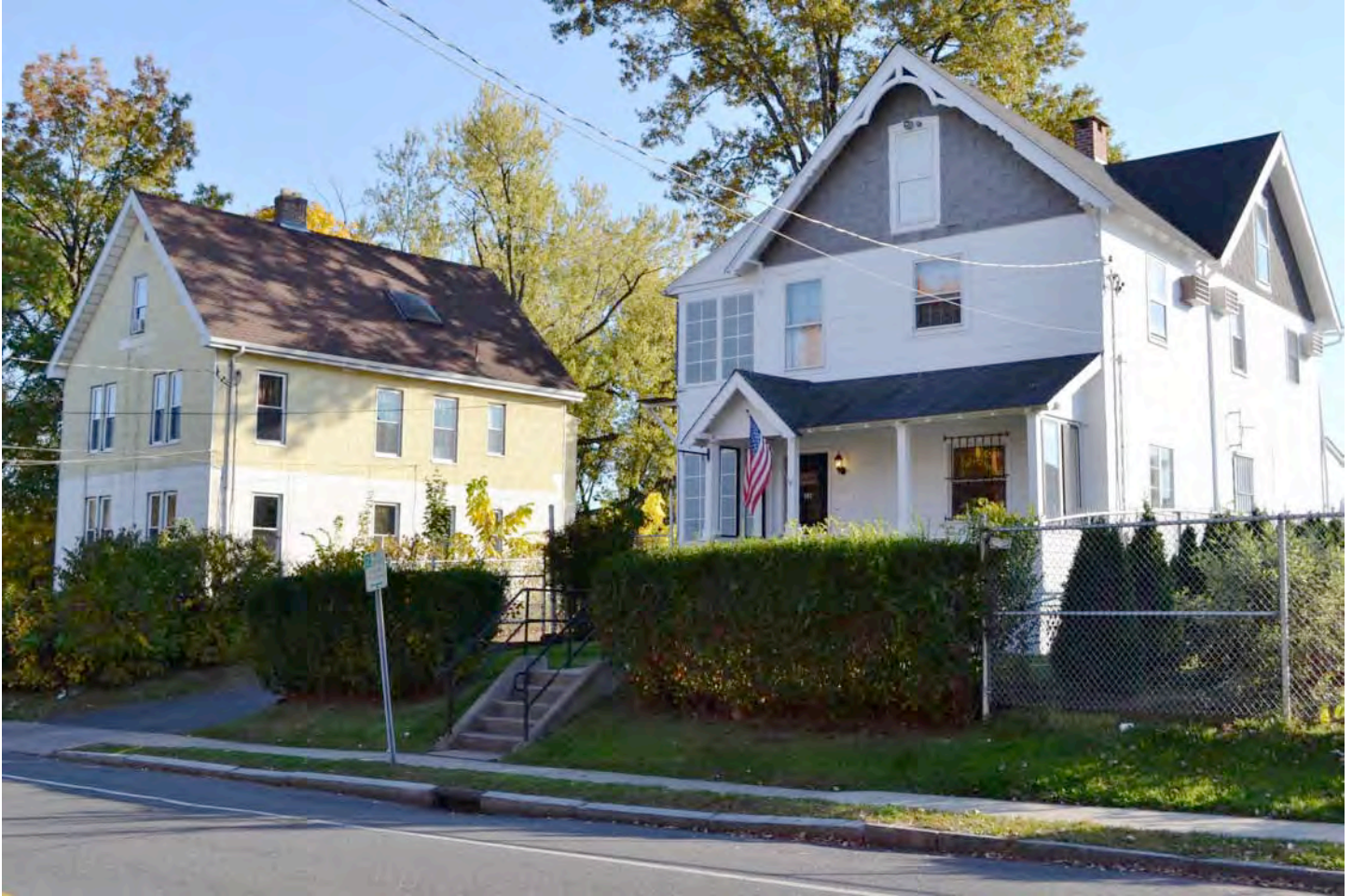
North (front) and west (side) elevations of (from left to right) 191 and 197 Hamilton Street (1893 and 1890). Camera facing southeast. Photograph 33 of 58.
