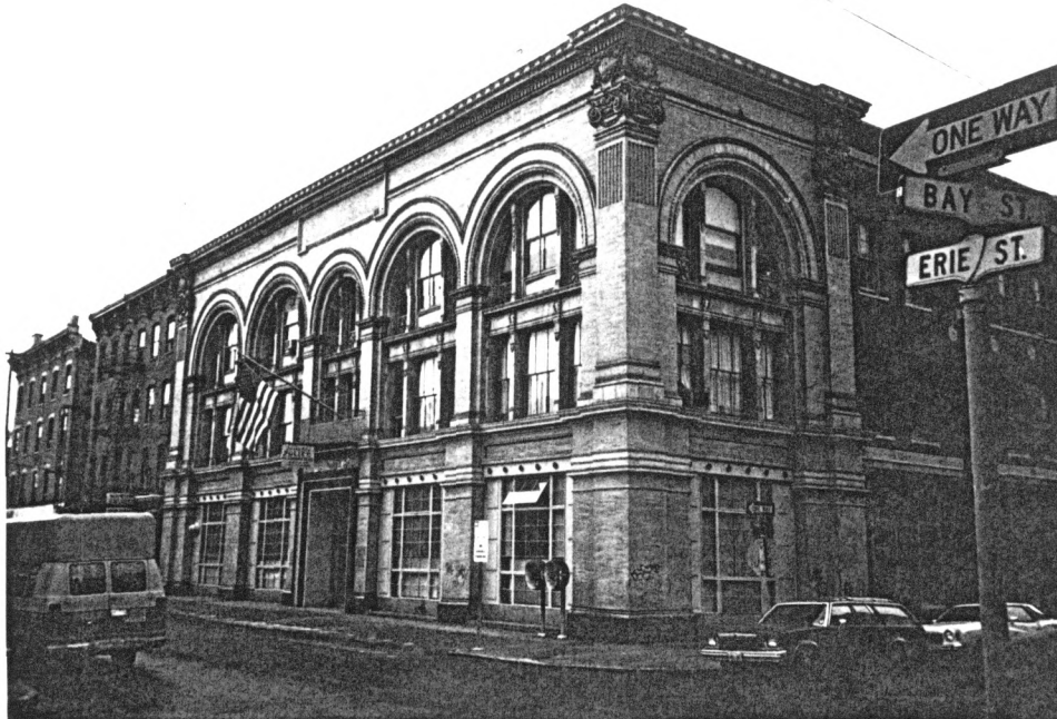
Police Headquarters 8 Erie Street
