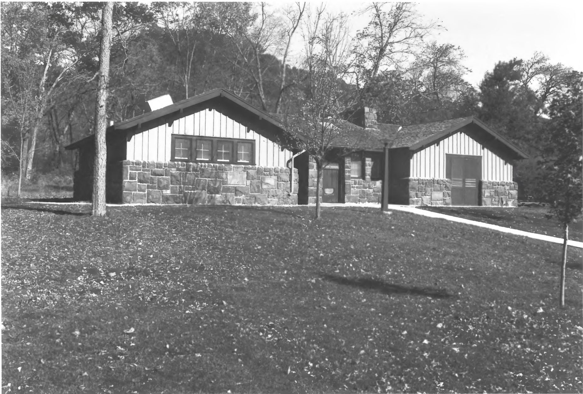
INTERSTATE STATE PARK CHISAGO CO. MN BLDG #5 PHOTO I.D. 09336#8
