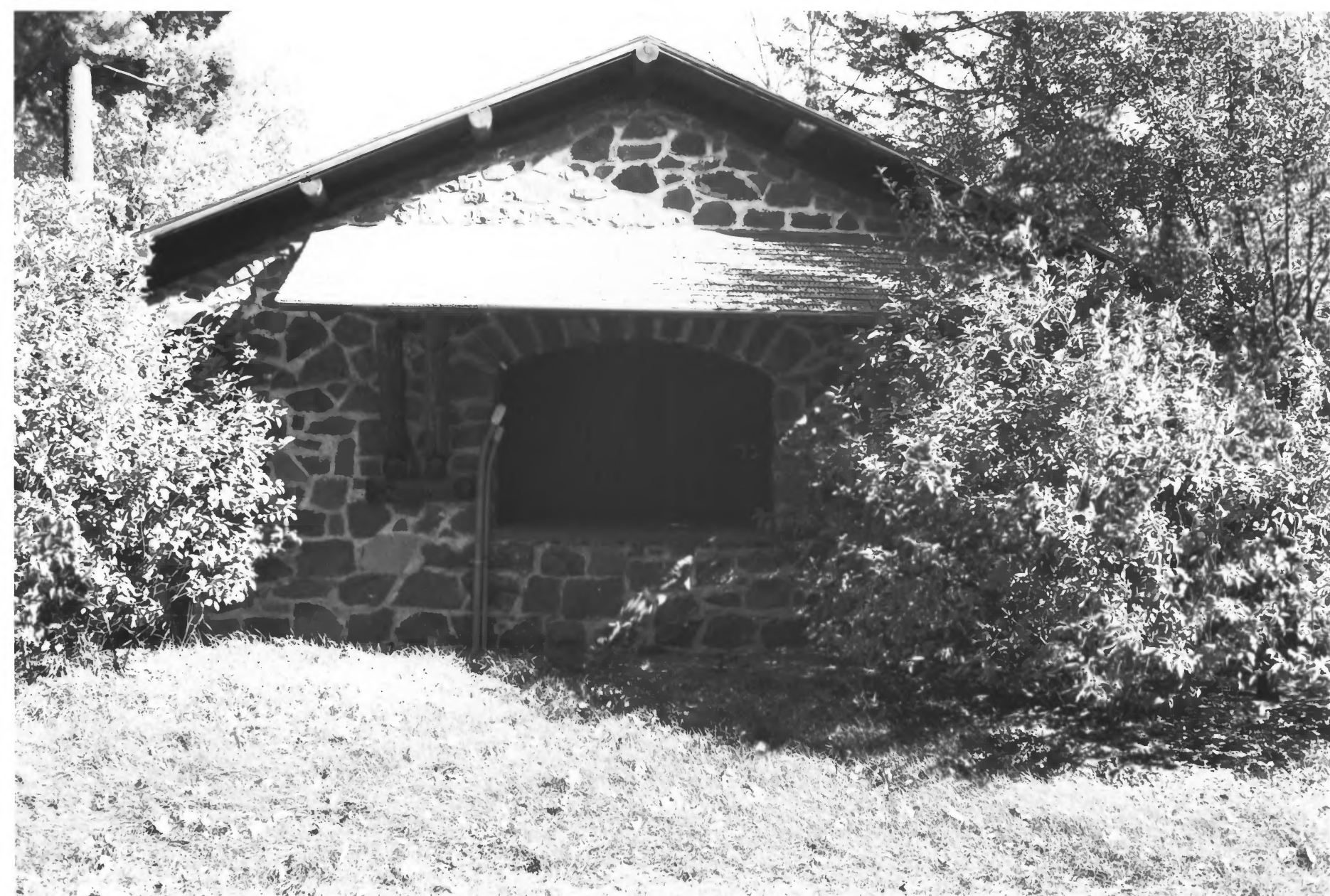
INTERSTATE STATE PARK CHISAGO CO., MN BLDG # 2 3, PHOTO I.D. 09336 #15
