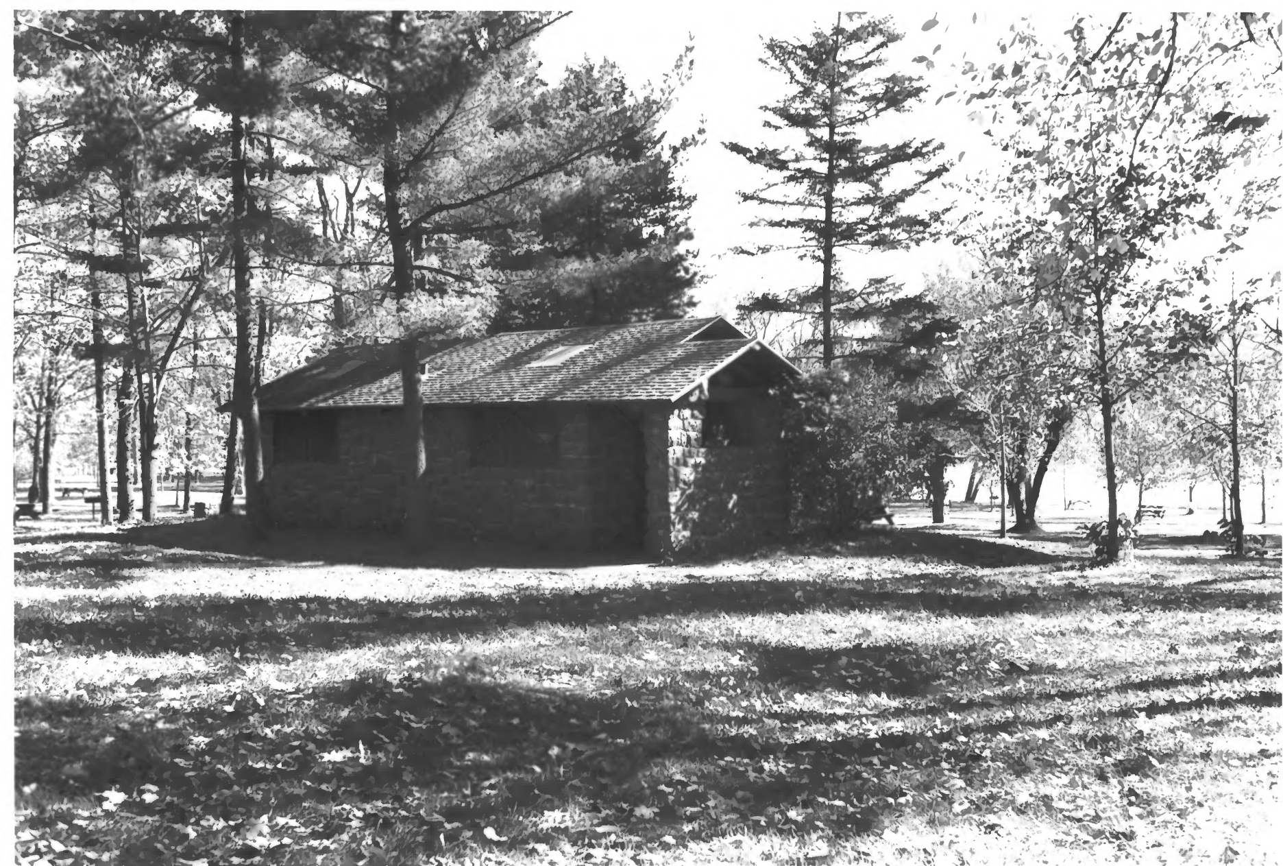
INTERSTATE STATE PARK CHISAGO CO., MN BLDG # 7 PHOTO I.D. 09336 #14
