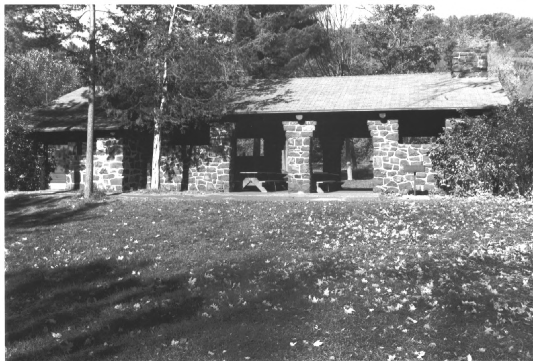
INTERSTATE STATE PARK CHISAGO CO. MN BLDG #3 PHOTO I.D. 09336 #4
