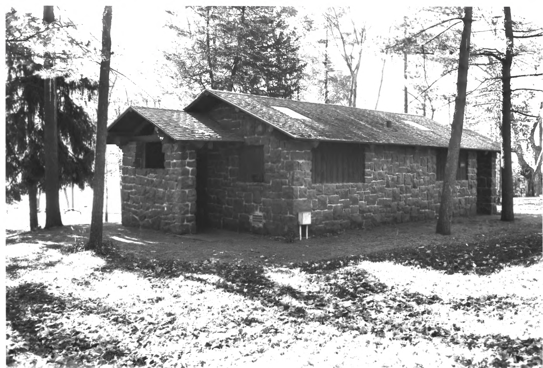
INTERSTATE STATE PARK CHISAGO CO., MN BLDG# 1 PHOTO I.D. 09336#1
