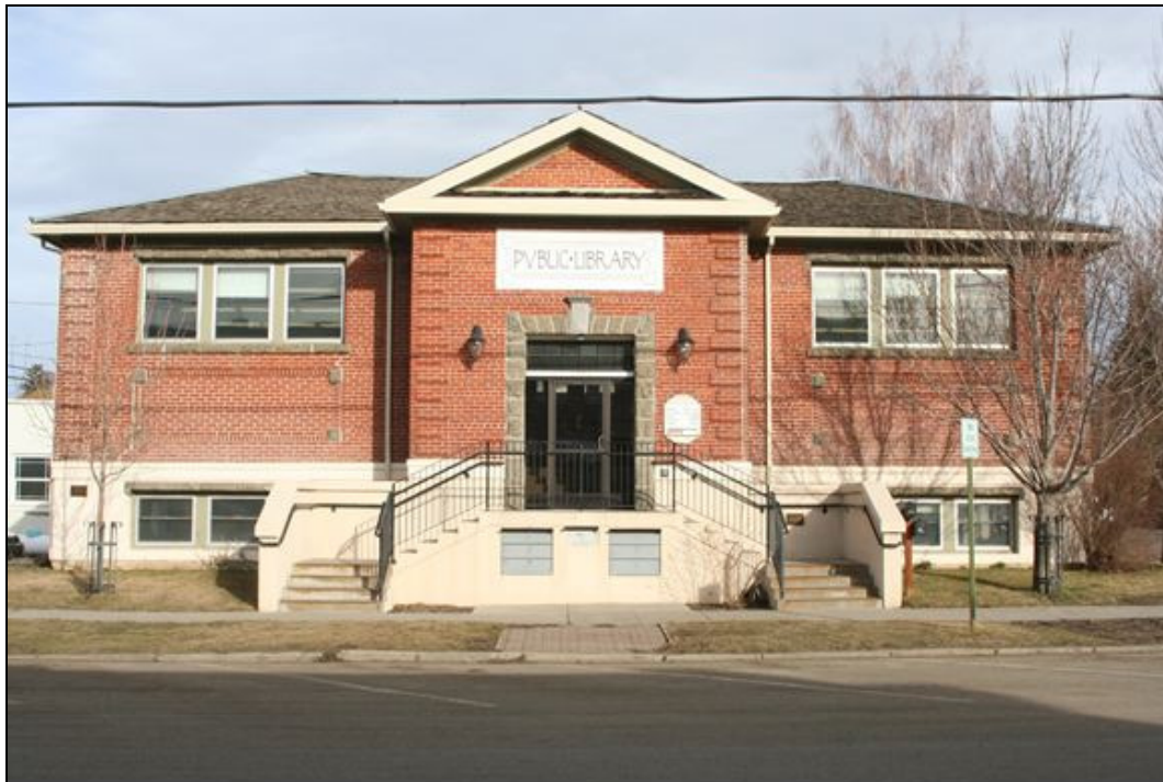
Photo 2 of 14: West façade (front), looking east.
