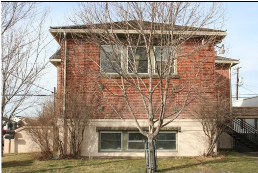
Photo 8 of 14: South façade, looking north.
