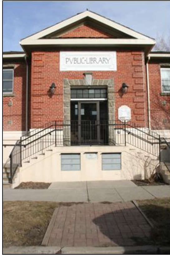
Photo 3 of 14: West façade, looking east at central entrance.
