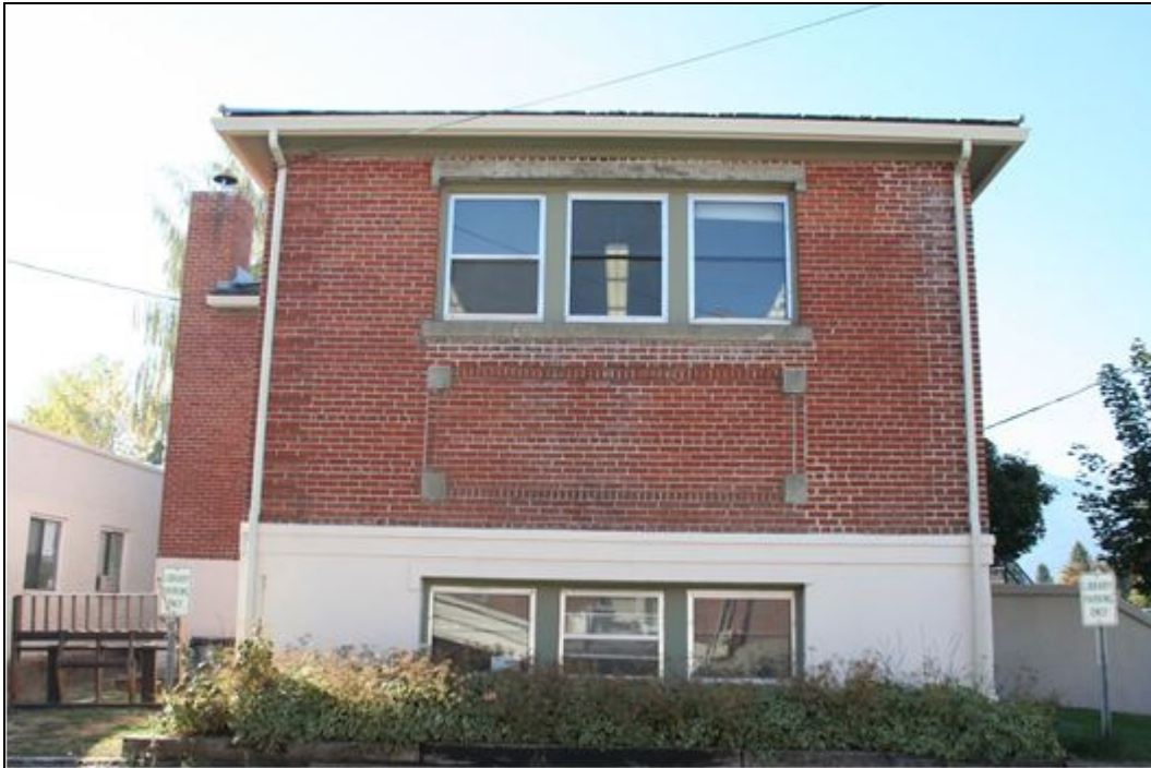
Photo 5 of 14: North façade, looking south.
