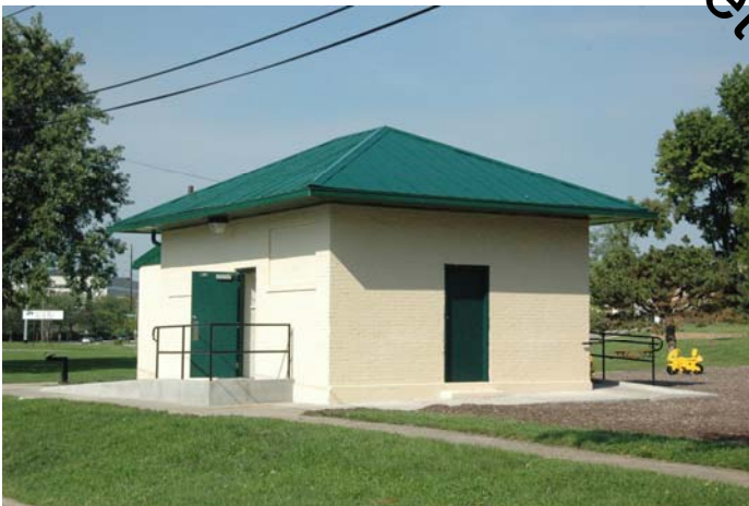
Photo 14: Restroom: view to west
