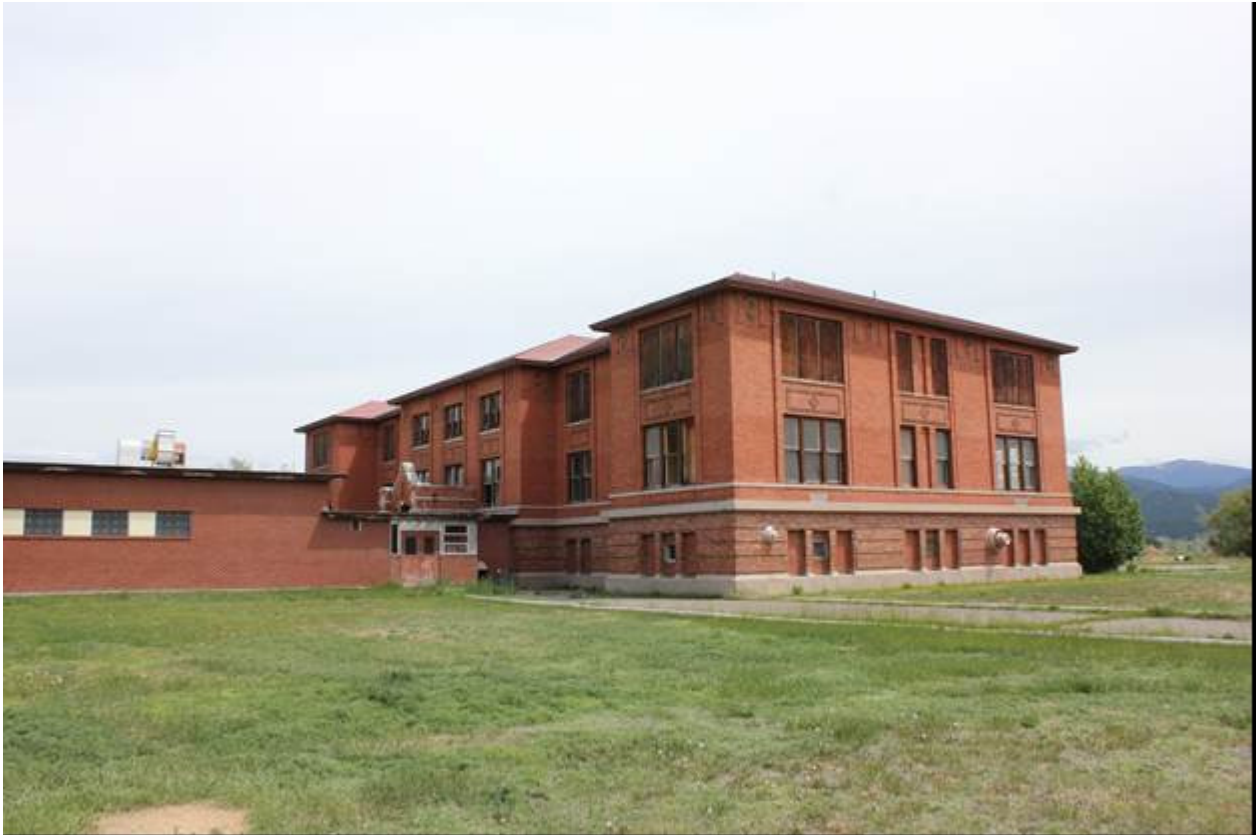
0003 of 0039 Griffin Hall (right) and Food Center (left), South elevations, view to northeast.
