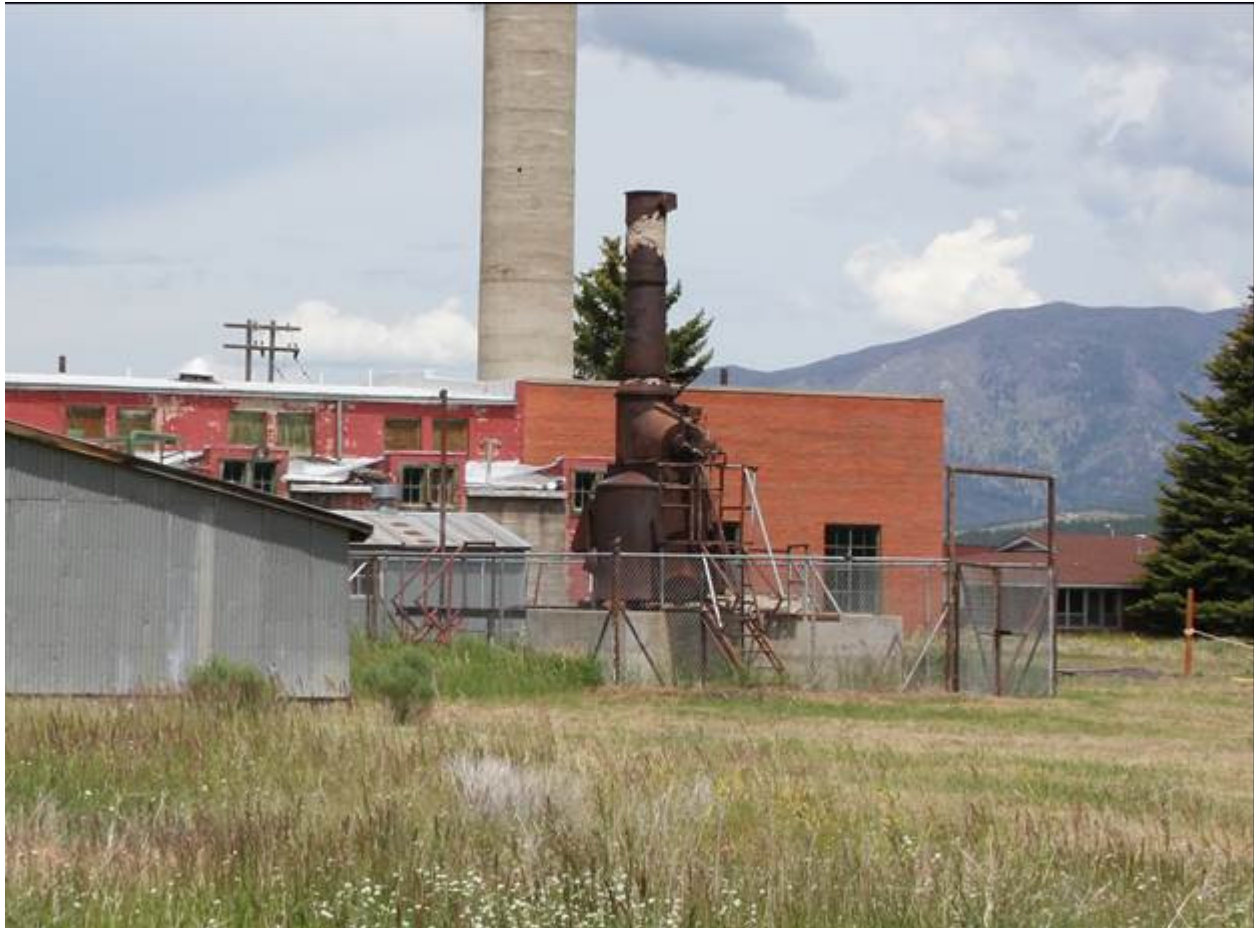
0025 of 0039 Boiler, view to northeast.
