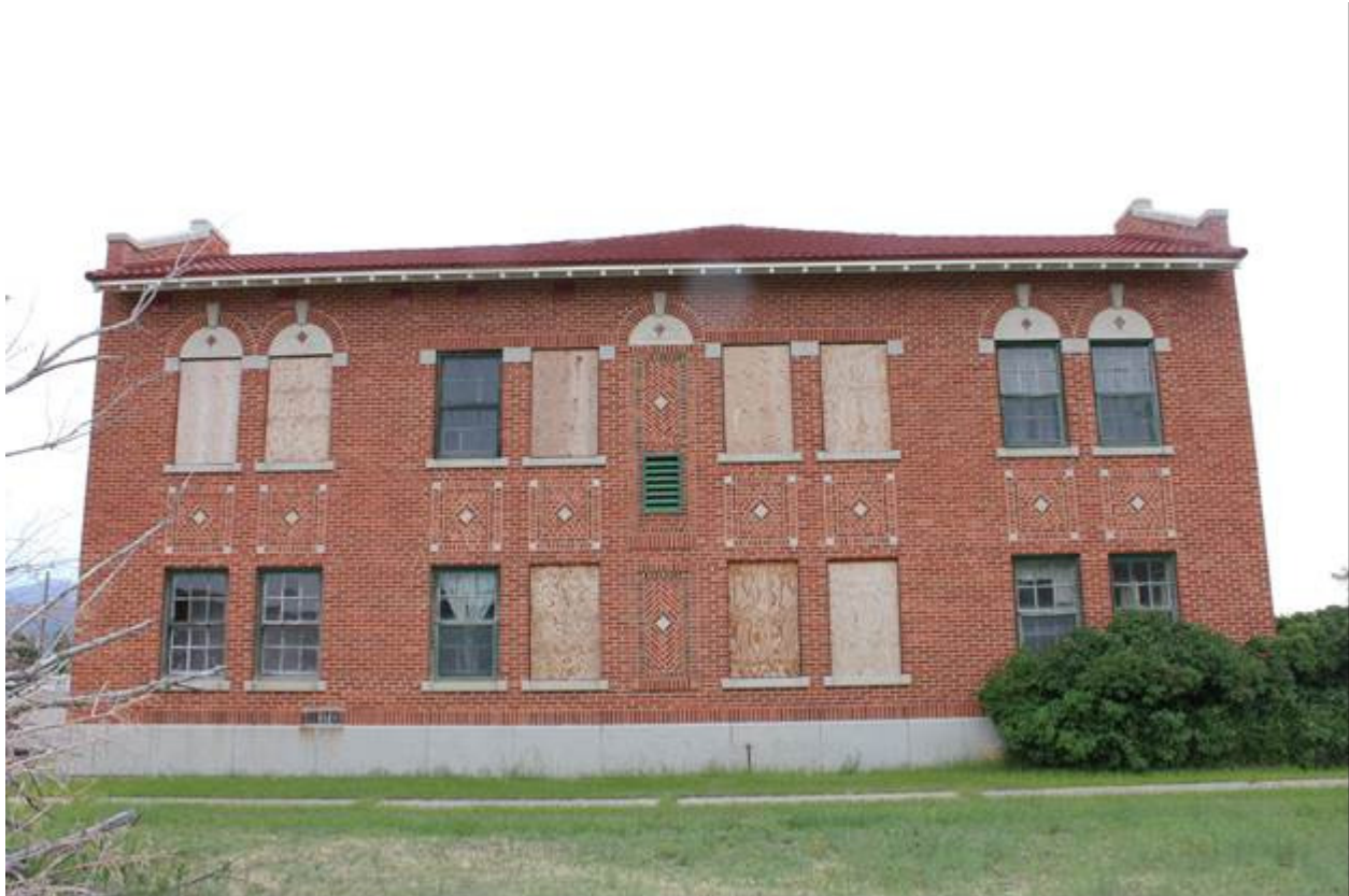
0010 of 0039 Cottage #5, West elevation, view to the east.
