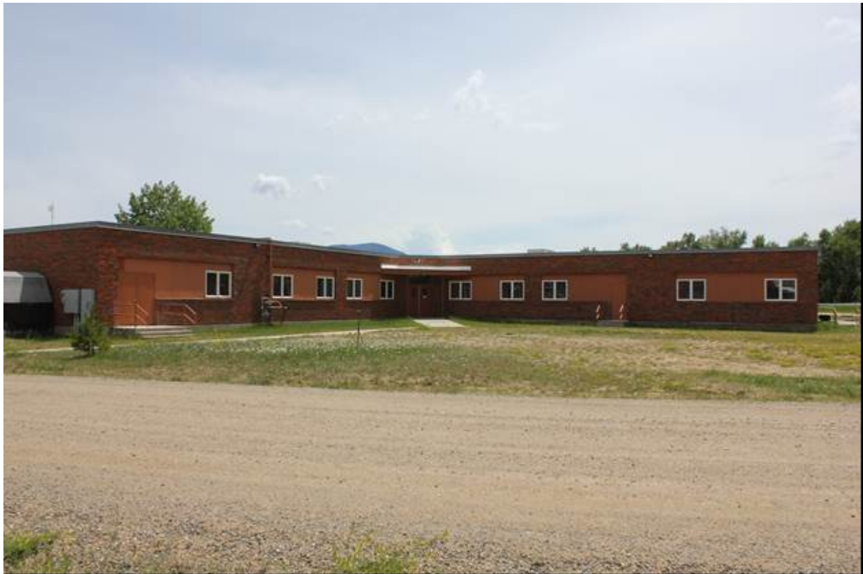
0018 of 0039 Southern X Dormitory, Northwest elevation, view to southeast.
