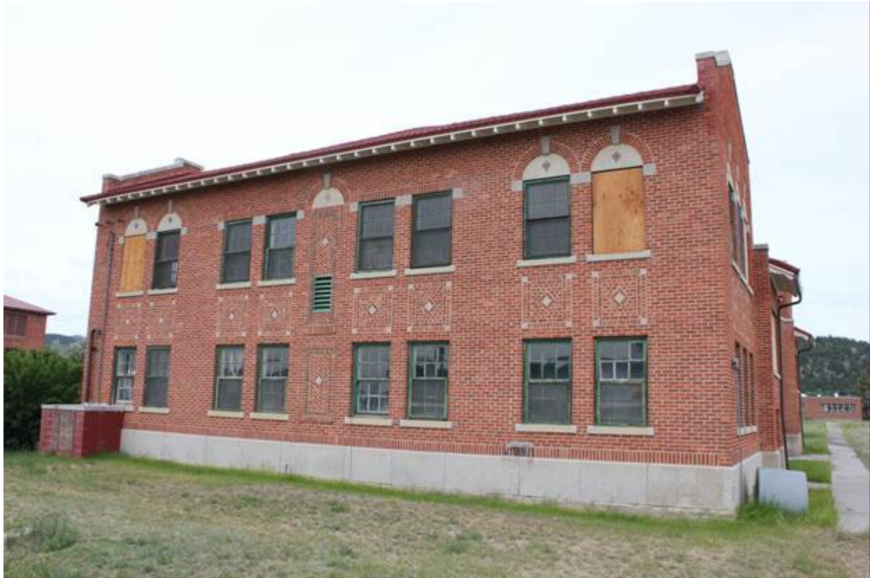
0009 of 0039 Cottage #5, East elevation, view to southwest.
