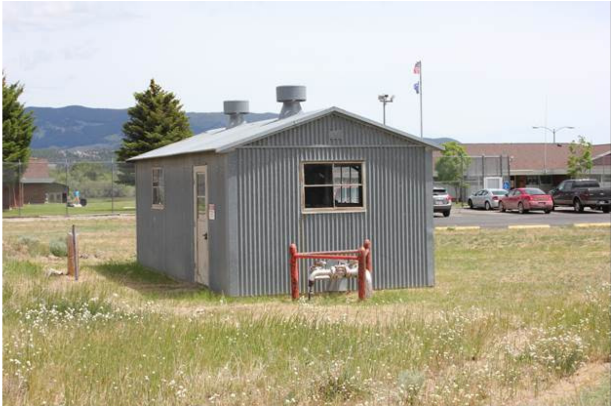
0039 of 0039 Metal Electrical Shed, North and West elevations, view to southeast.
