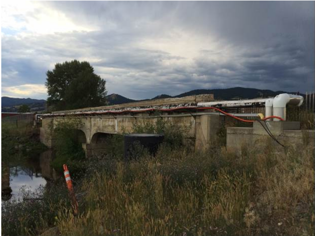
0033 of 0039 Bridge, view to the west-southwest
