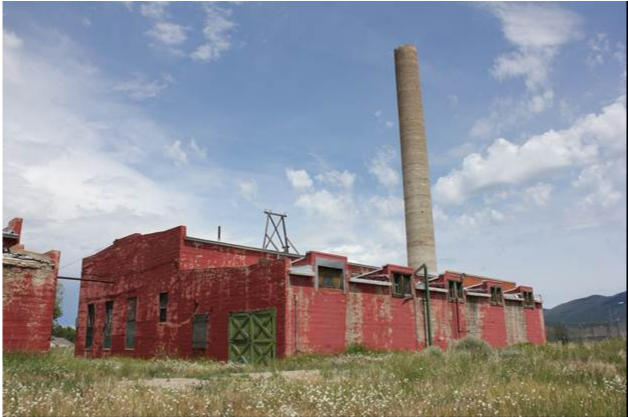
0031 of 0039 Power House, West and South elevations, view to northeast.
