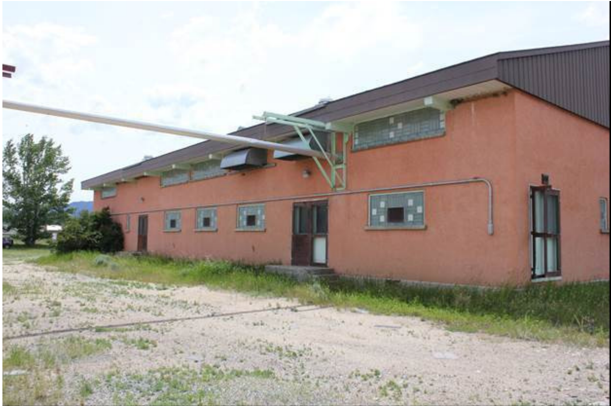
0027 of 0039 New Laundry, East elevation, view to southwest.
