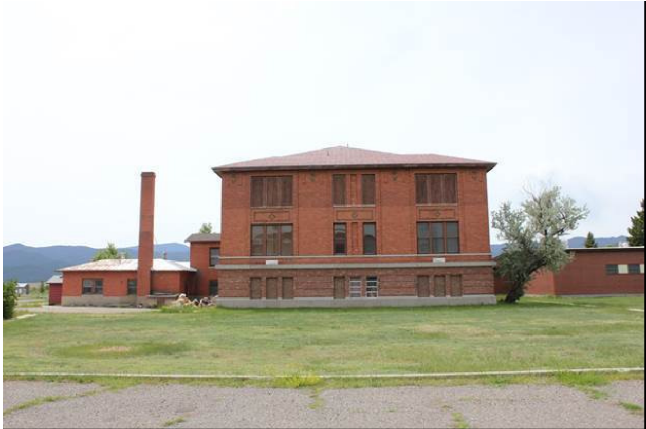
0006 of 0039 Griffin Hall, North elevation, view to south.
