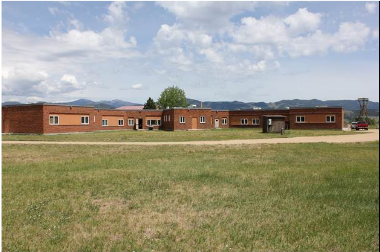
0019 of 0039 Southern X Dormitory, Southwest elevation, view to northeast.
