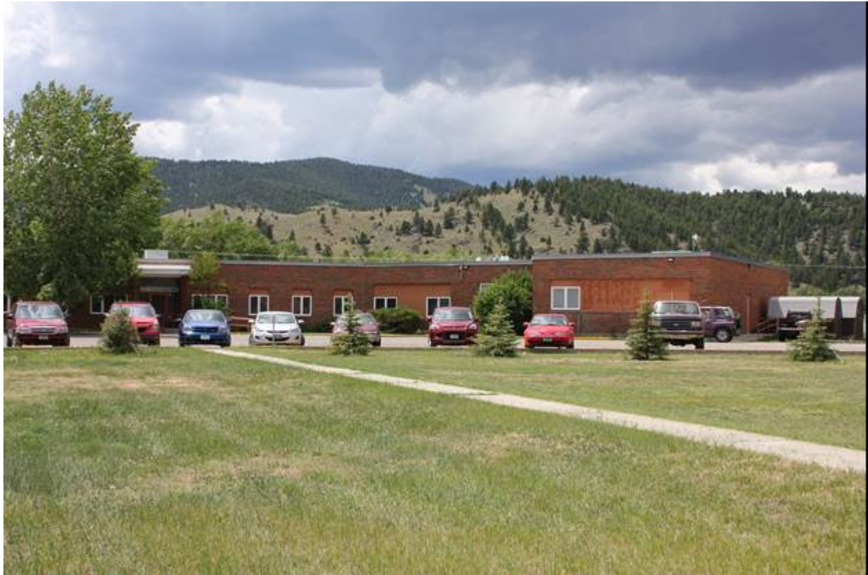
0016 of 0039 Southern X Dormitory, Northeast elevation (N1/2), view to northwest.
