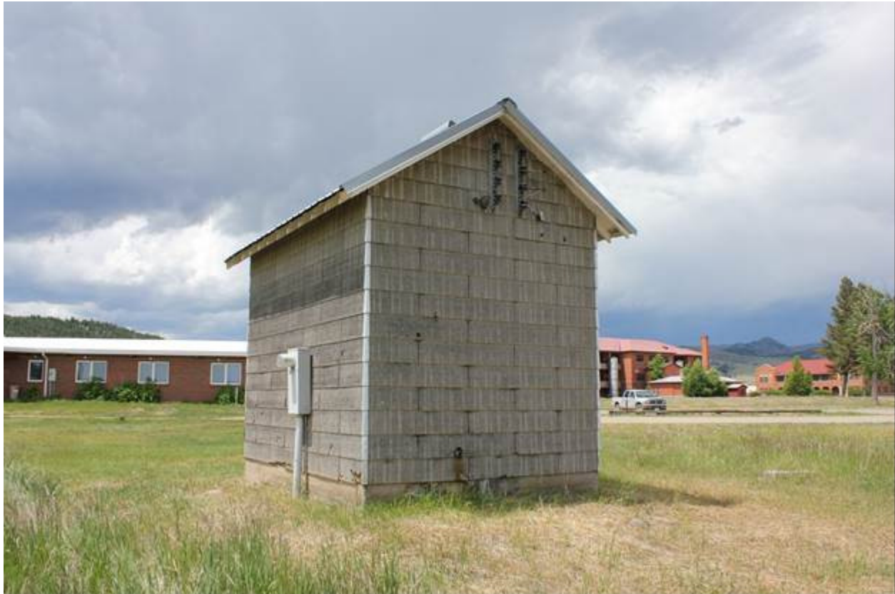
0038 of 0039 Electrical Shed, South and East elevations, view to northwest.
