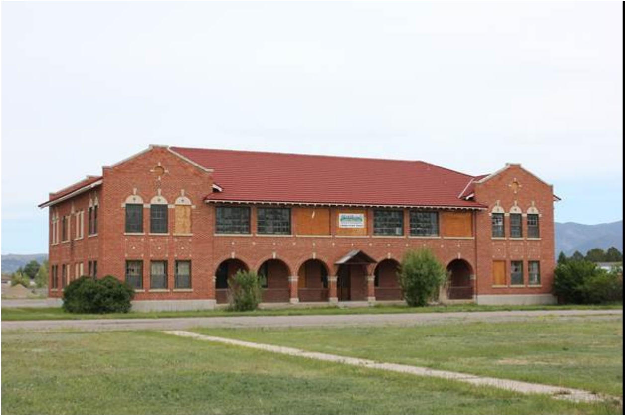
0007 of 0039 Cottage #5, South elevation, view to north-northeast.
