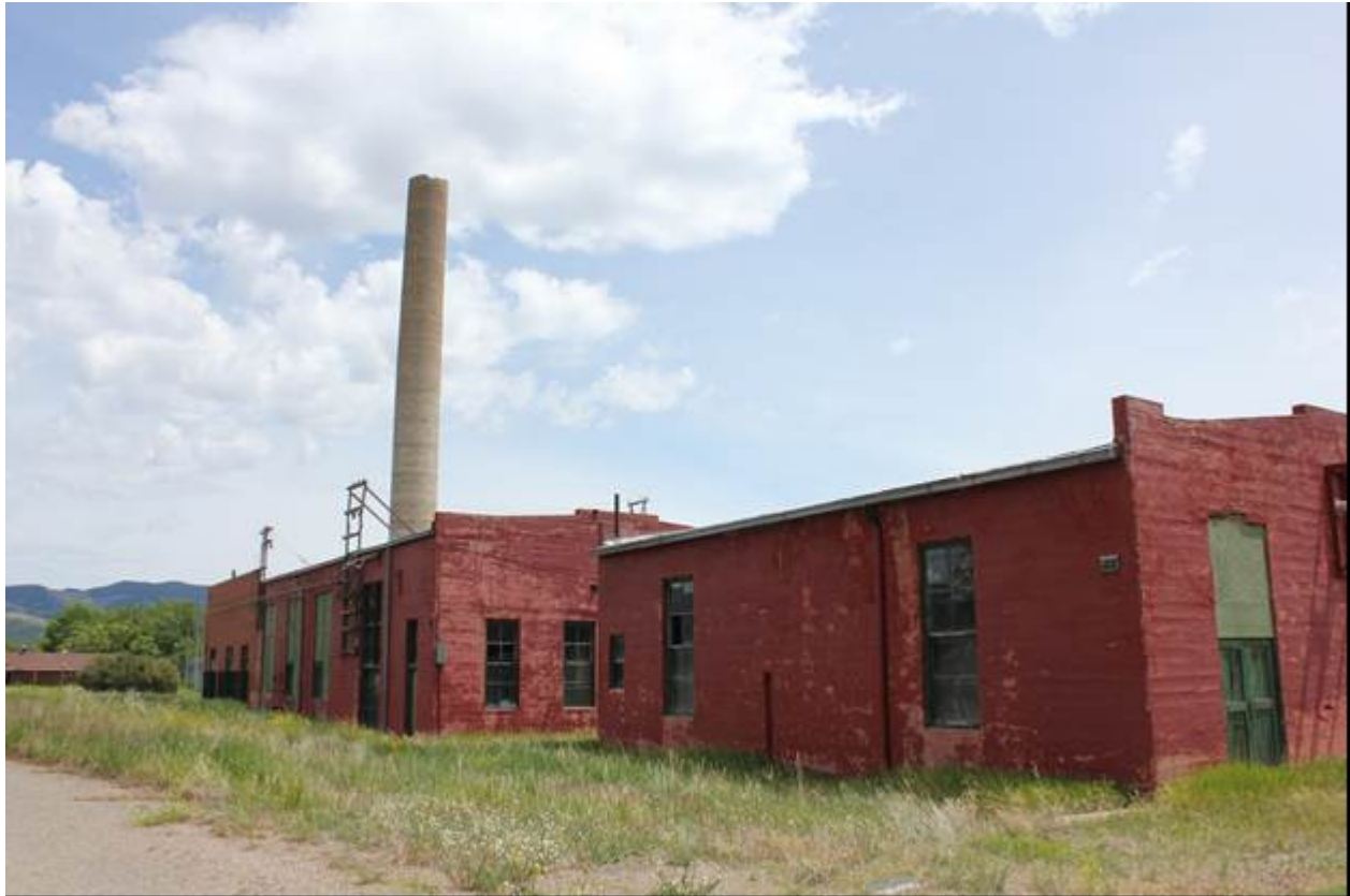
0030 of 0039 Old Laundry (foreground) and Power House (background), North elevations, view to southeast.
