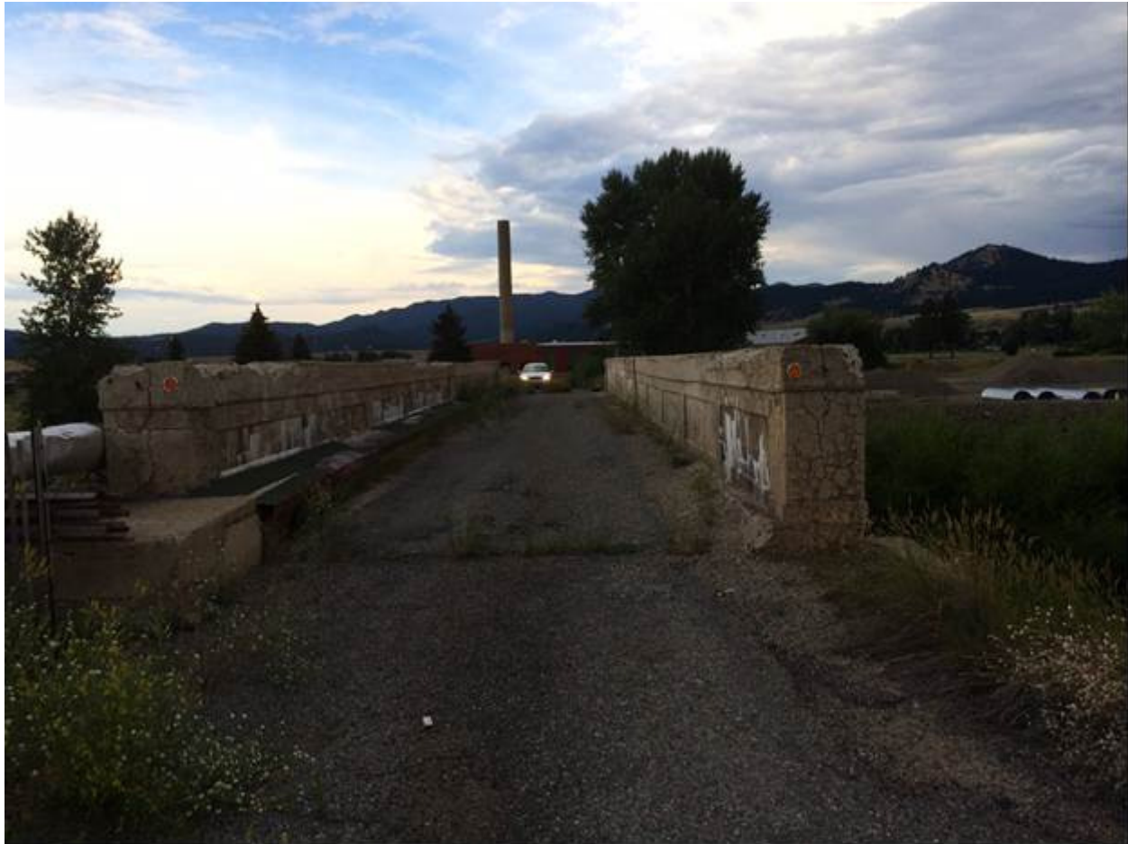
0032 of 0039 Bridge, view to the southwest
