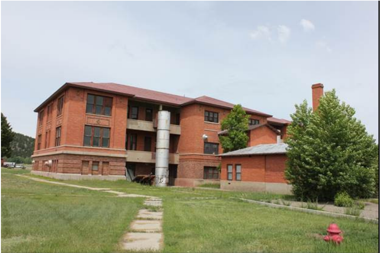
0004 of 0039 Griffin Hall, East elevation, view to northwest.
