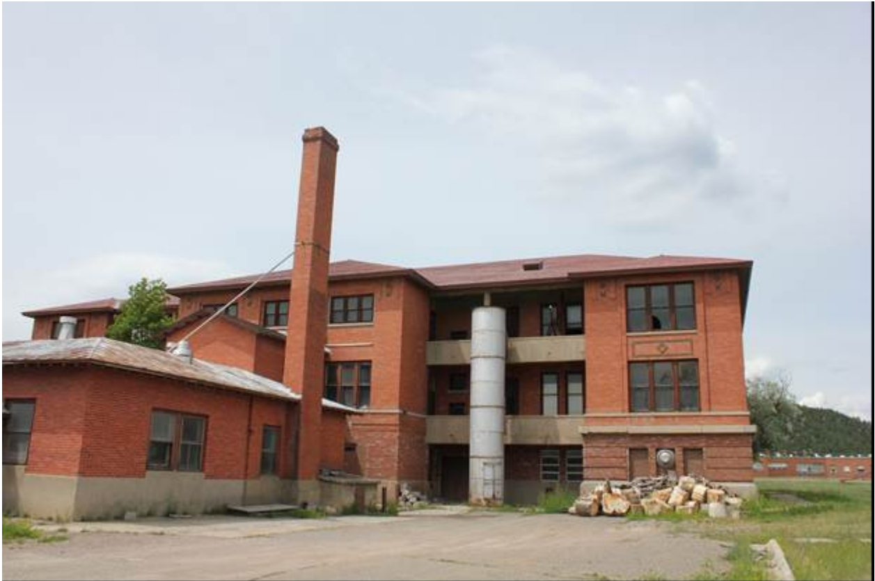
0005 of 0039 Griffin Hall, East elevation, view to east-southeast.
