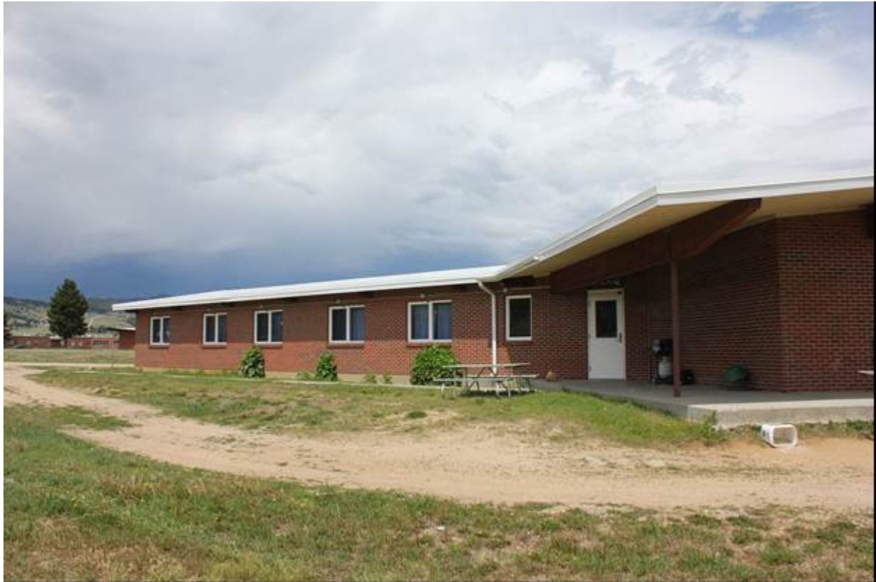
0021 of 0039 Ranch Boys' Dormitory, Southwest and West elevations, view to northeast.
