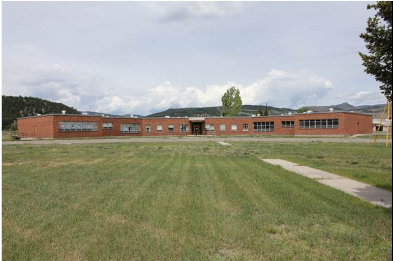
0011 of 0039 Northern X Dormitory, Southeast elevation, view to northwest.
