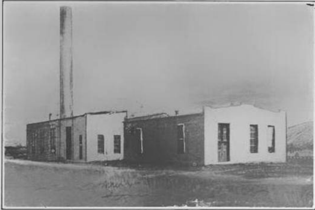
Power House and Laundry.
