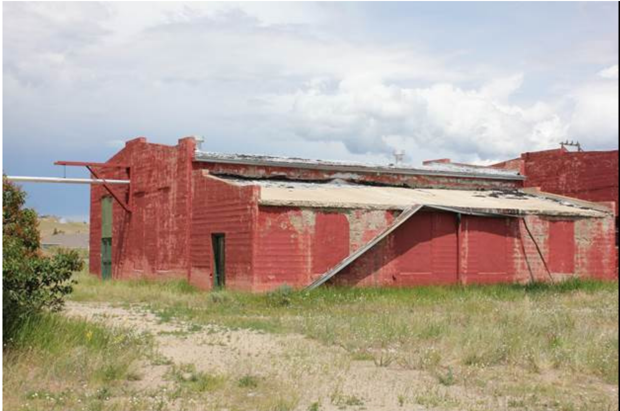
0029 of 0039 Old Laundry, West and South elevations, view to northeast.
