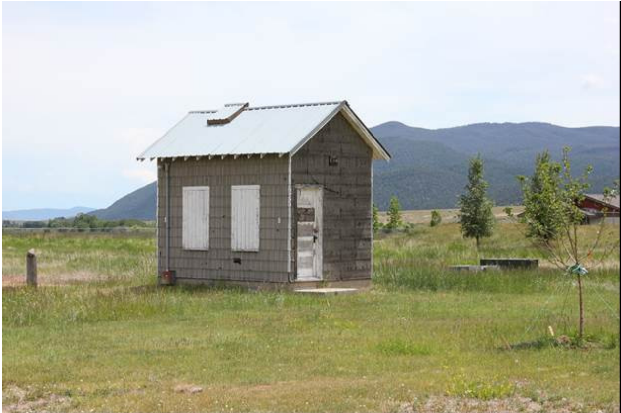
0037 of 0039 Electrical Shed, North and West elevations, view to southeast.
